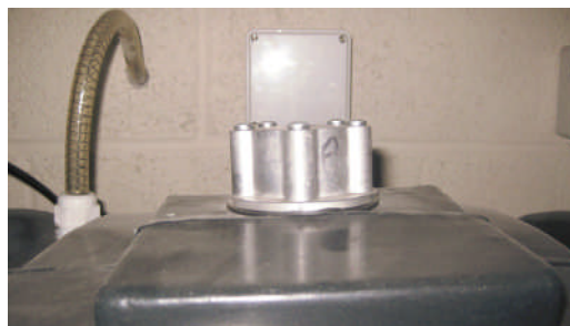
Fig 1.1 The top of the probe, on top of an oil storage tank.
