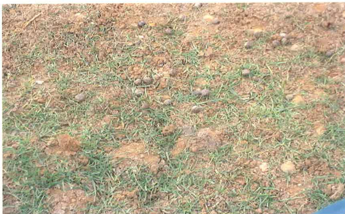
Plate 1.1 Poor vegetation cover on Silvermines TMF surface
