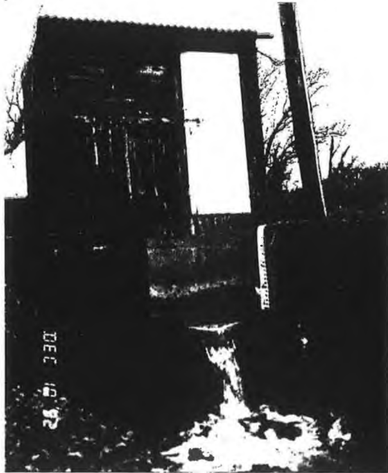
PHOTO 1 Crossmolina Spring and V-notch weir
