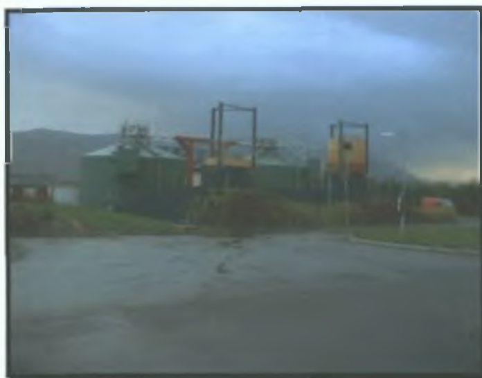
Figure 5.3 Mesophilic Anaerobic Digestion at Tralee
