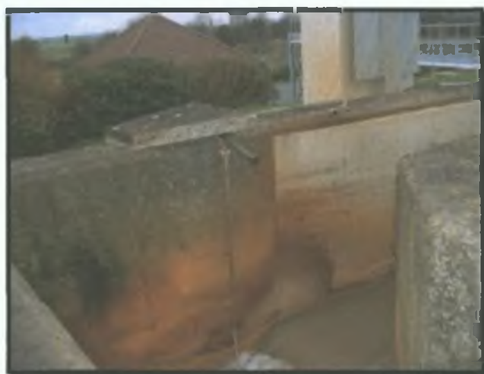
Figure 5.9 Ferric chloride dosing at Tullamore wastewater treatment plant.
