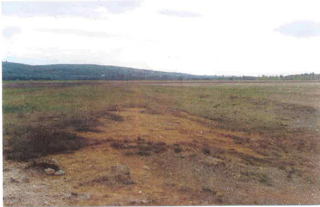
Figure 1.7 Tailings dam at Silvermines with obvious acid burn in foreground.
