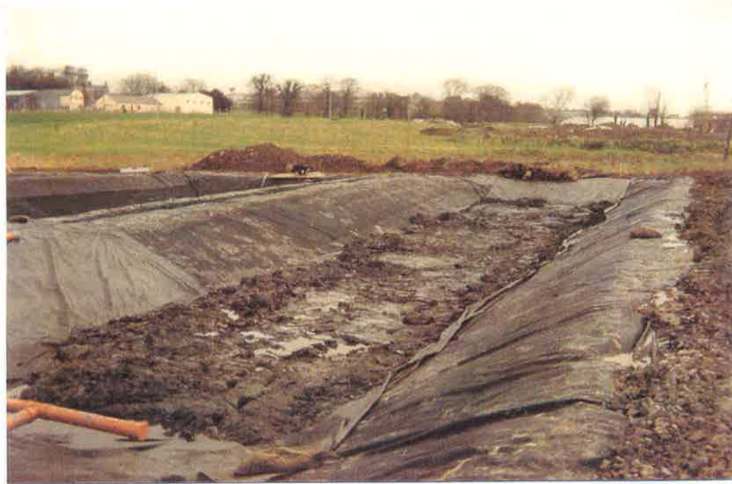
Fig. 3.7 TMF Wetland with pyritic tailings in place.
