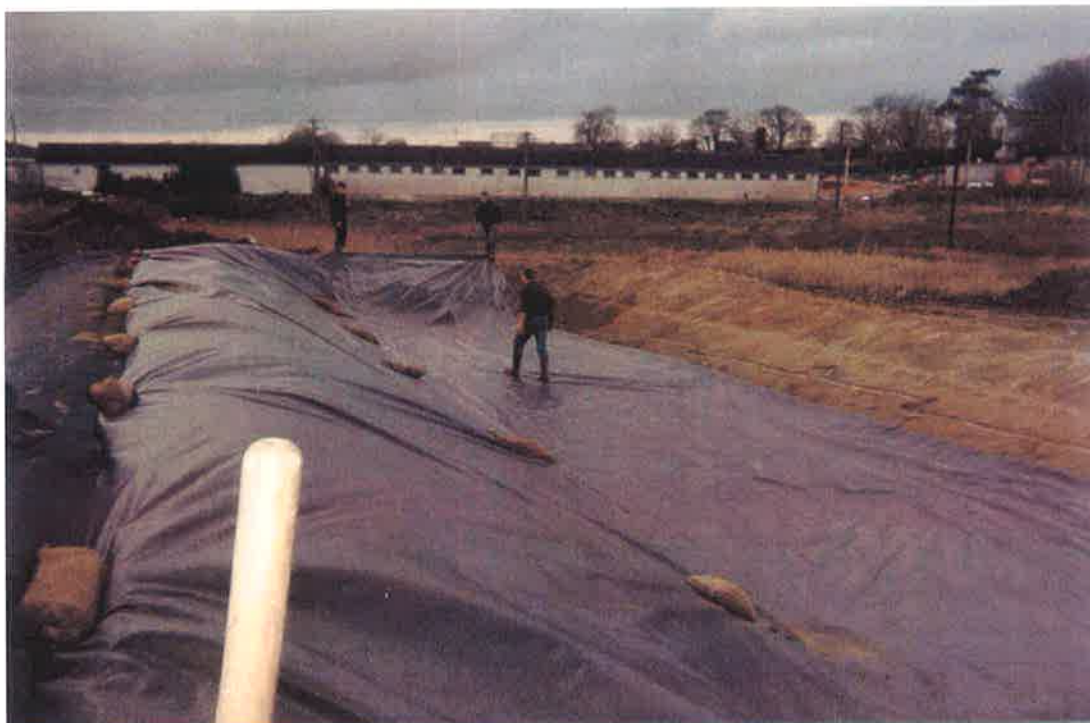
Fig. 3.5 Laying plastic construction sheeting as a protective layer for the EPDM liner.
