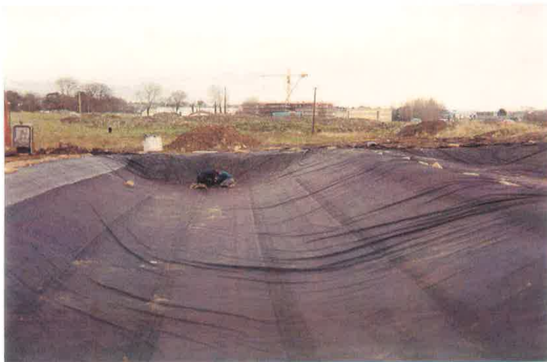
Fig. 3.5 Laying plastic construction sheeting as a protective layer for the EPDM liner.
