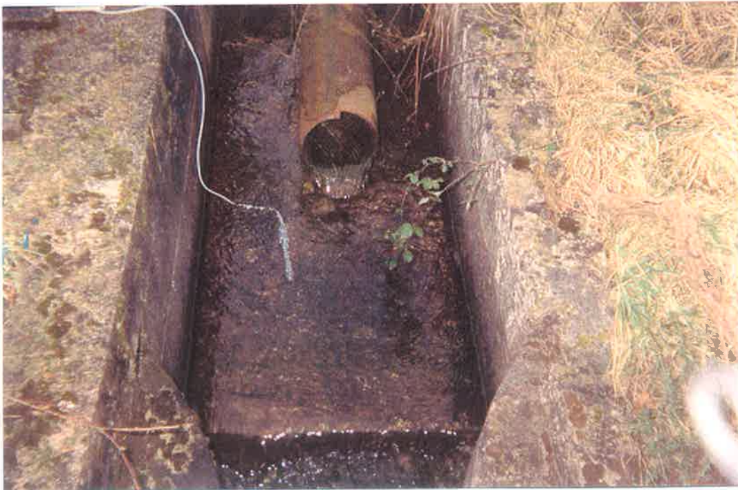
Fig. 3.19 Drainage discharging into the Kilmastulla River following passage through Wetlands 1, 2, 3, and 4 at Silvermines.
