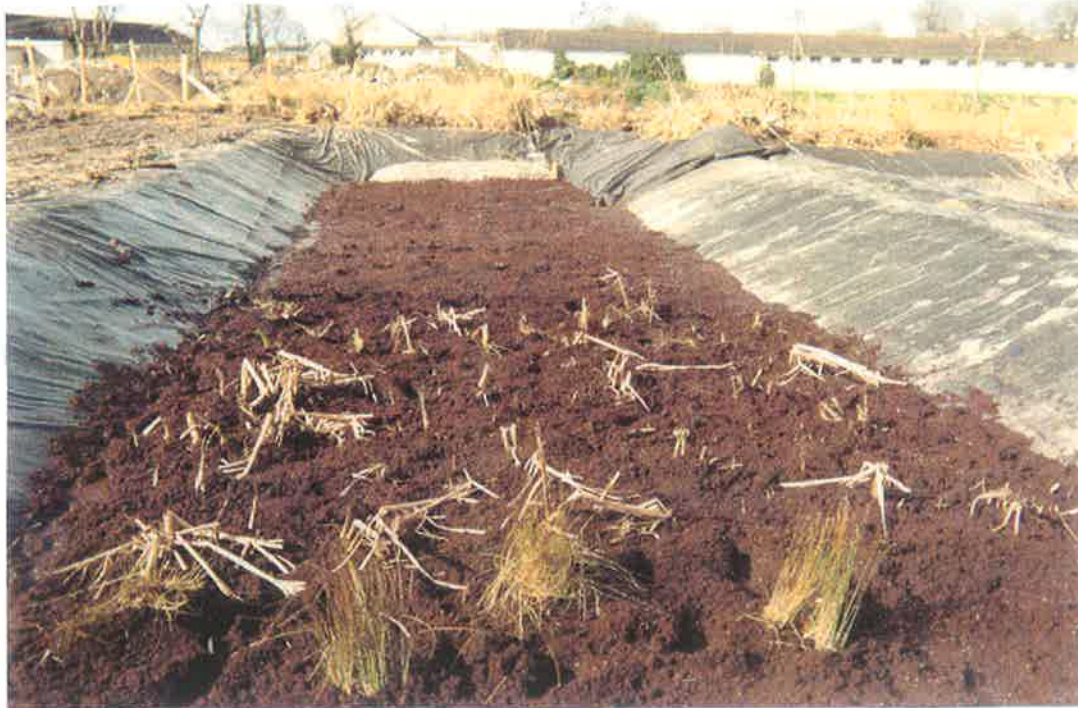
Fig. 3.8 Peat cover over the tailings in the TMF Wetland in March, 1998 with initial planting of wetland macrophytes.
