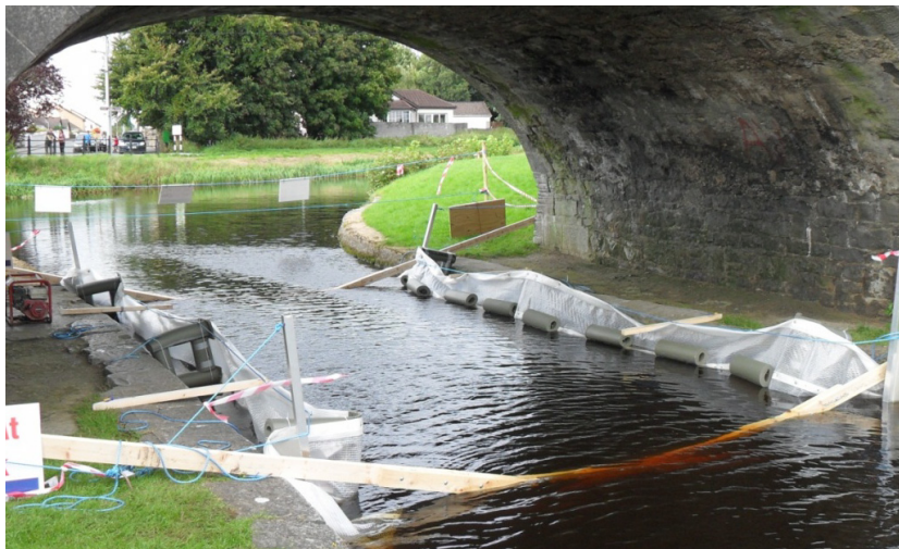
Figure 2. Impermeable curtains used to hold treated water within treatment area along canal walls. Photograph by Sara Meehan.
