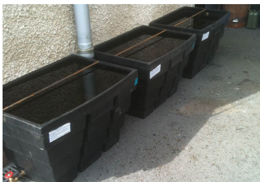
Figure 2. Bioboxes outside of Sligo drinking water treatment plant (photograph by Sara Meehan).
