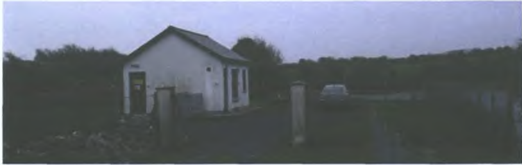
Figure 6.1: Kinvara PWSS Raw Water Source at Loughcurra South (image Authors own)
