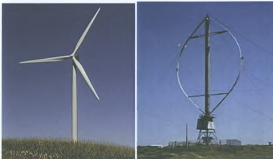
Plate 2.2: HAWT (left) and VAWT (right)
