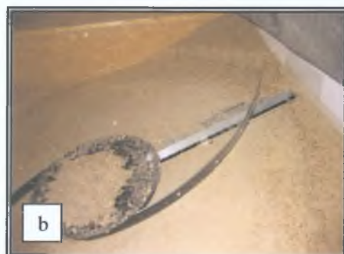
Plate 4.9: (a) Biomass Boiler and (b) Automatic Feed in a Wood Pellet Boiler, Lough Key Forest Park, Co. Roscommon
