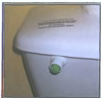
Plate 4.13: Retrofit Water Conservation Device for WC
