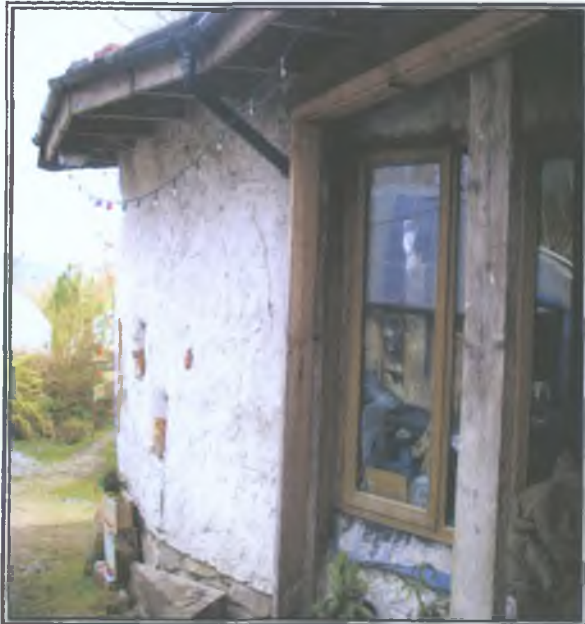
Plate 4.20: Straw Bale Office, KEEP
