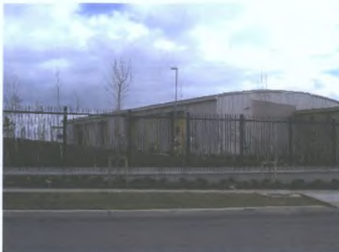
Plate 16: Dun Laoghaire-Rathdown Composting Facility for MSW.
