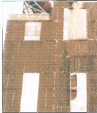
Asbestos cement vertical cladding
