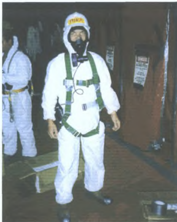
Figure 3.8 Person Dressed in Full Personal Protective Equipment for Protection Against Exposure to Asbestos ( www.environmentalhazards.com/asbestos/index.htm )
