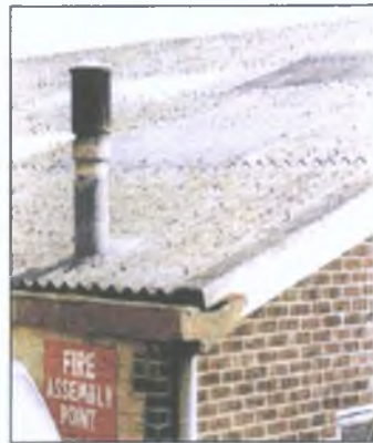
Asbestos cement external flue, rainwater gutter and profile roofing sheets
