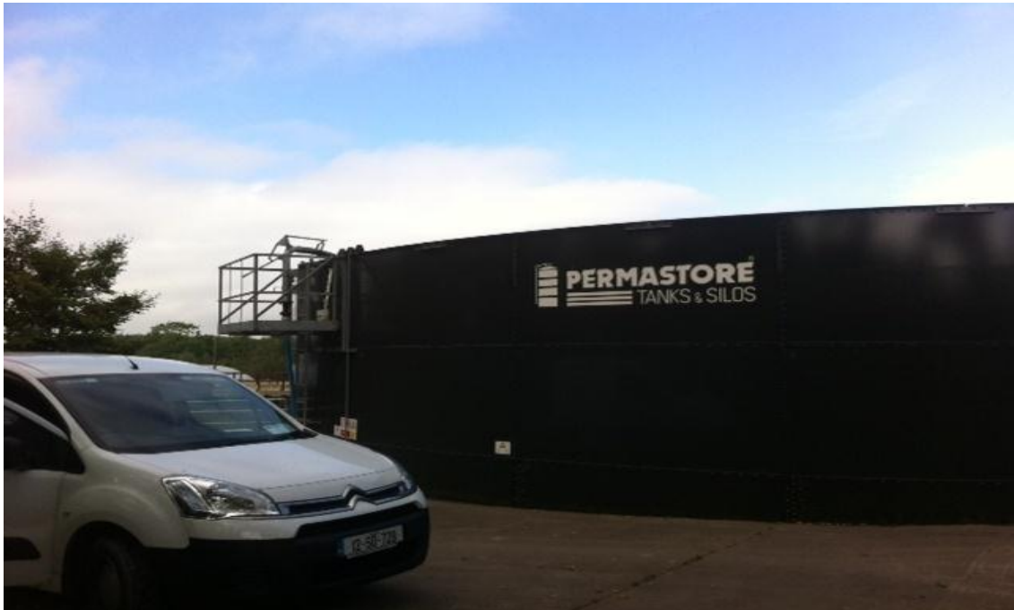
Plate 3.4: Storage tank used for dairy parlour washings at Hillsborough, Co. Down
