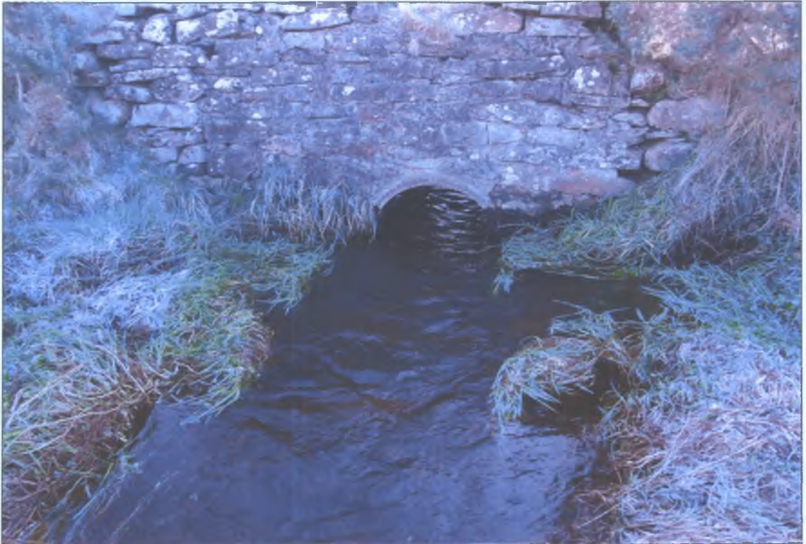
Plate 5.1 Round concrete culvert (So7) on Sonnagh River, Co. Mayo (S. Neylon)
