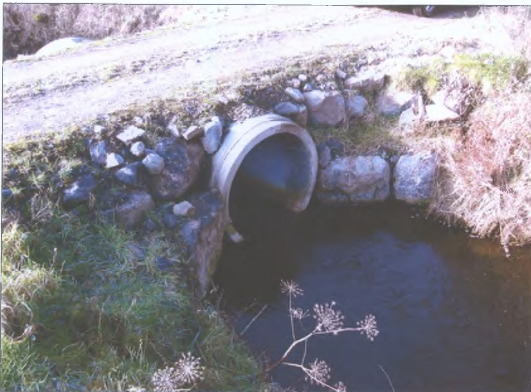
Plate 2.3 Round culvert on Gweestion River, Co. Mayo (S. Neylon)
