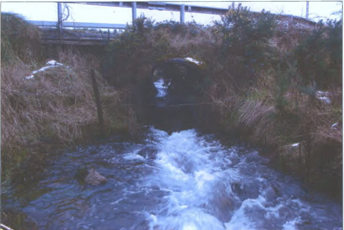
Plate 5.2 Round concrete culvert (So13) on Sonnagh River, Co. Mayo (S. Neylon)
