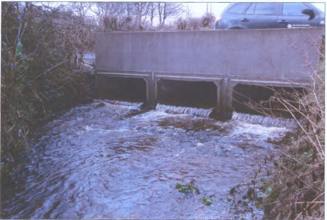
Plate 2.2 Box culverts on Brusna River, Co. Mayo (S. Neylon)
