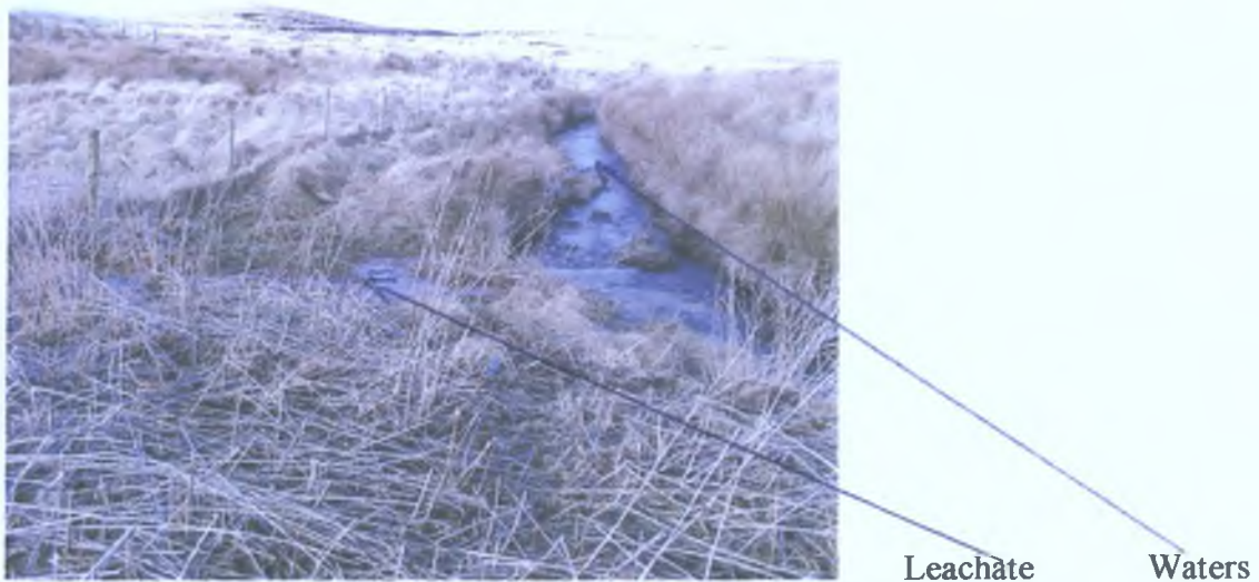
Plate 2.2 Seepage of leachate from Muckish landfill into receiving waters.
