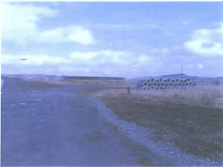
Plate 2.3 Drumaboden Puraflo system.
