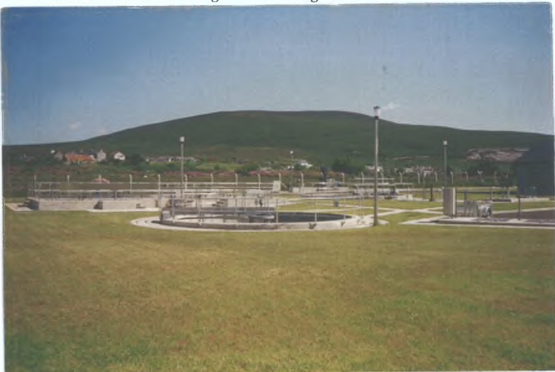
Plate 5.1: Overview of Bangor Erris Sewage Treatment Works
