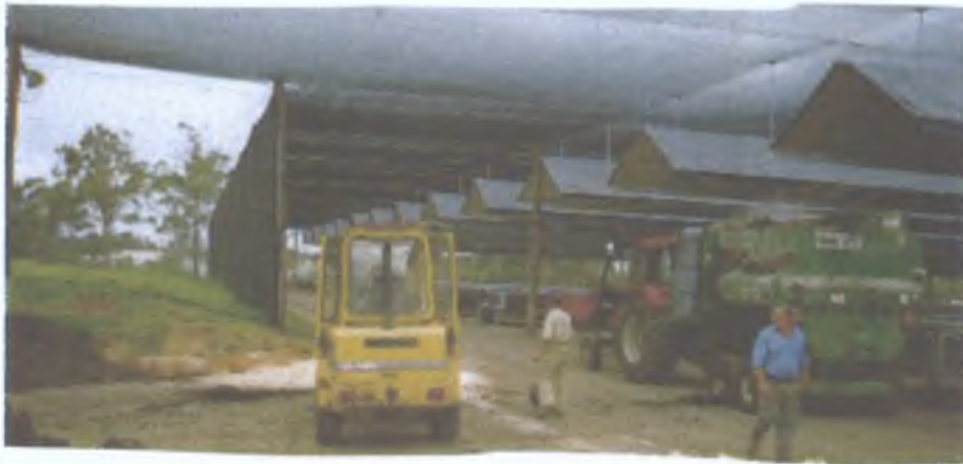
Plate 2.3: Vermitech Ltd. Site At Redlands, Australia, Using Continuous Flow System (adapted from Lotzof, 1999).
