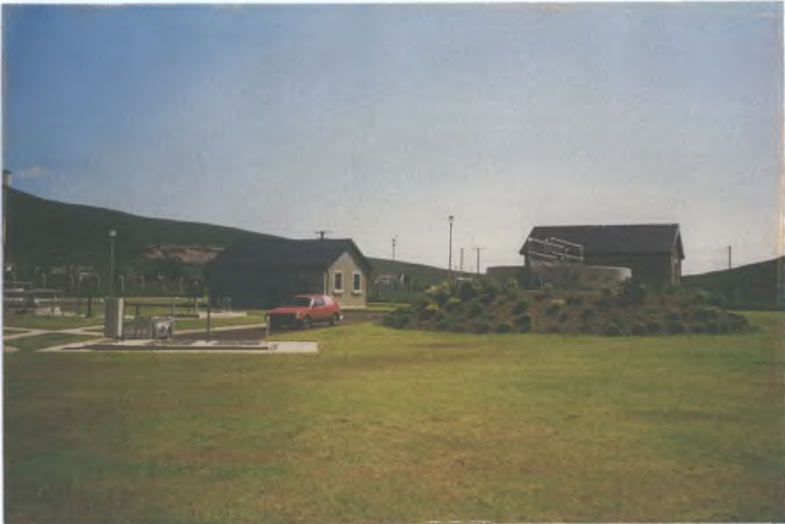
Plate 5.2: View Of Dewatering Building And Thickening Unit
