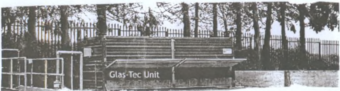
Plate 2.5: Small Scale Vermicompost Units
