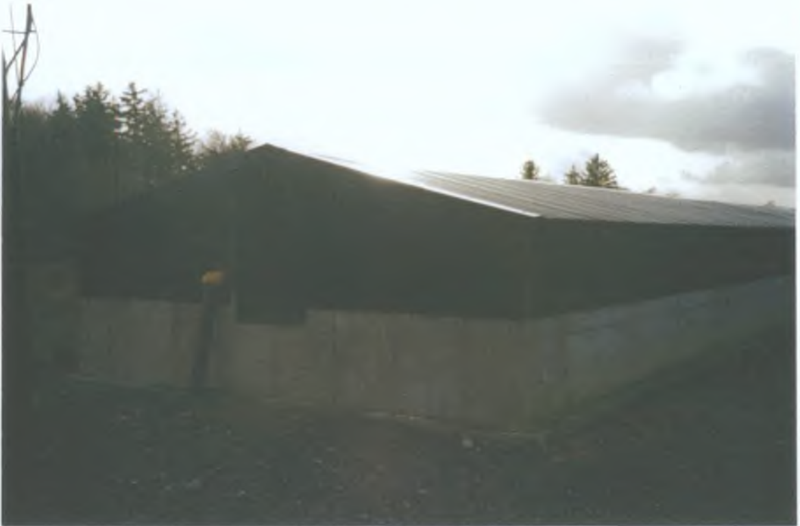
Plate 2.8: External View of Liquid Vermicomposting Unit At Toomevara STP, Co. Tipperary.
