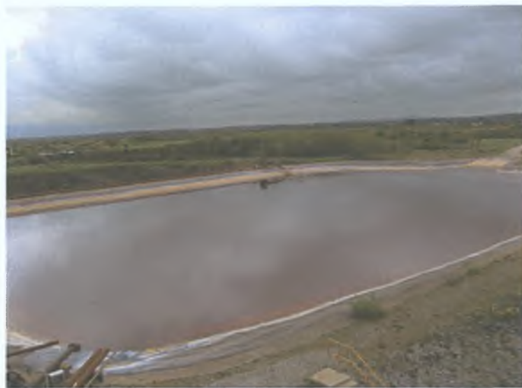
Plate 3.1 South Pond which provides storage capacity for clarifier feed water.
