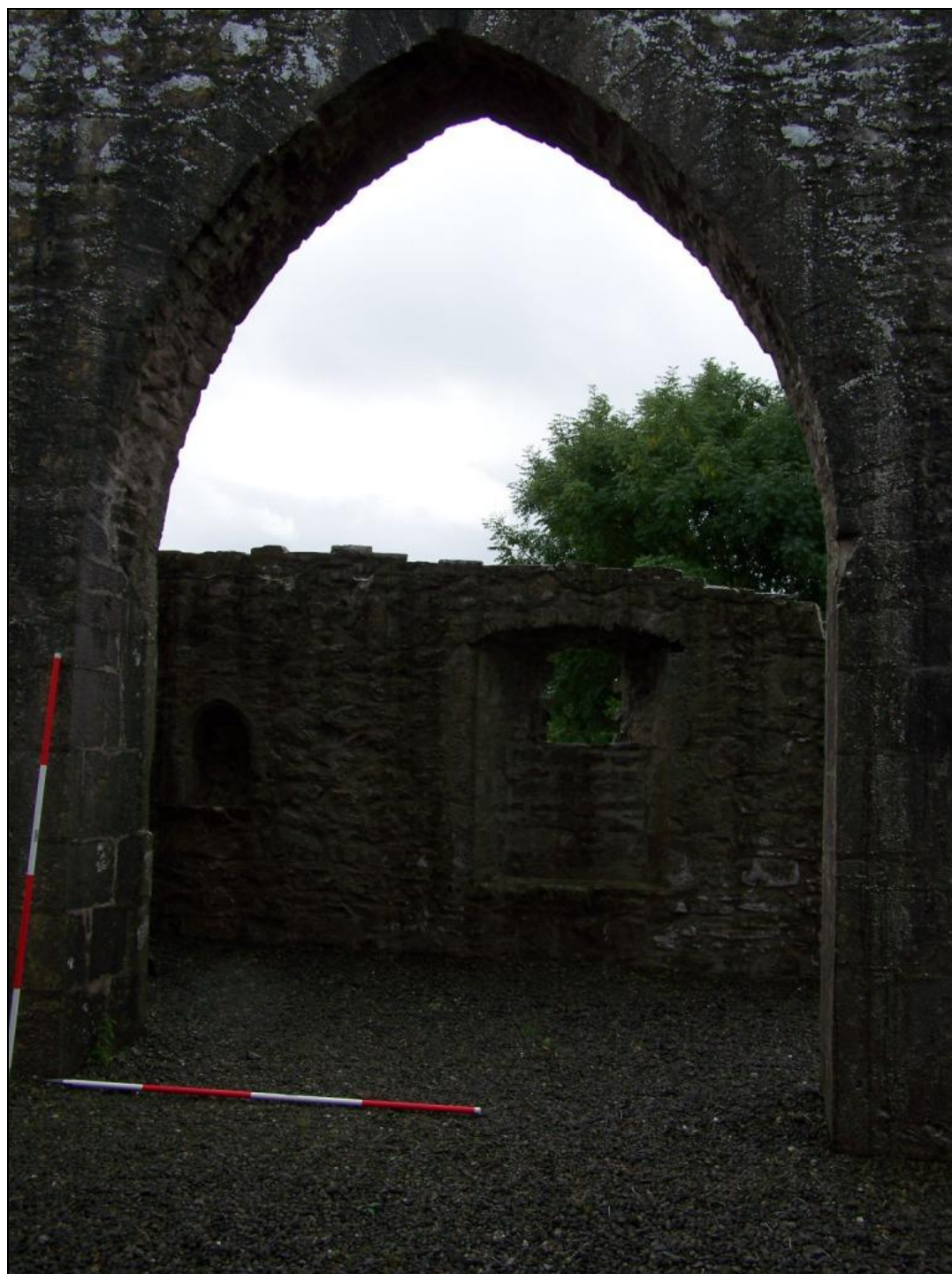
Figure 19: Archway leading to side aisle
