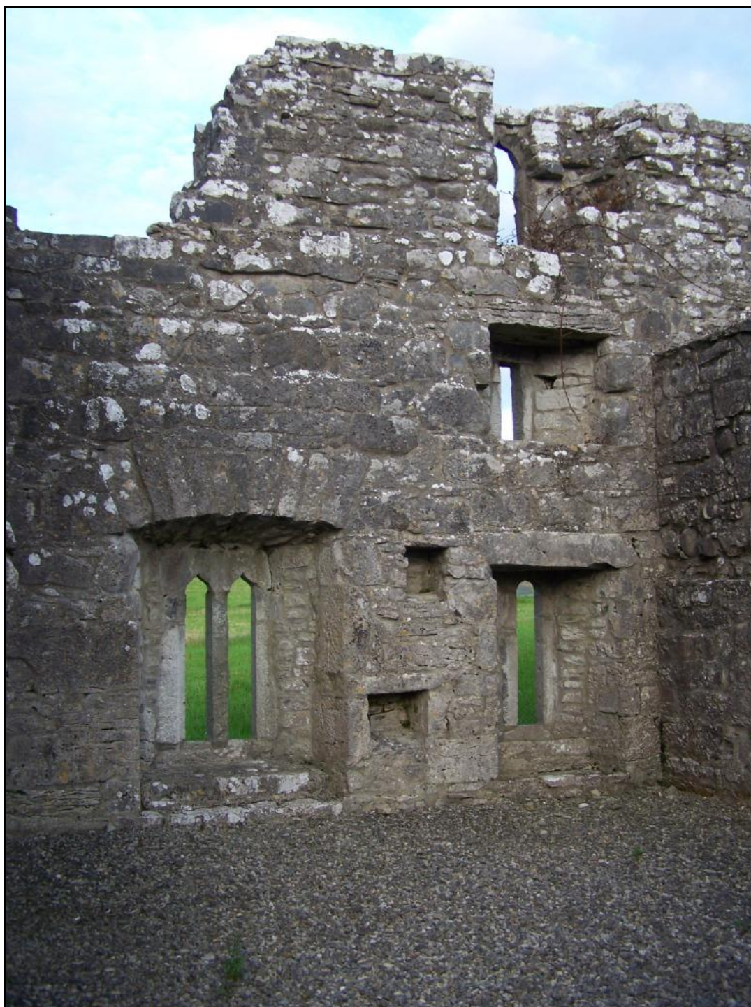
Figure 23: Part of the east range of Burriscarra friary
