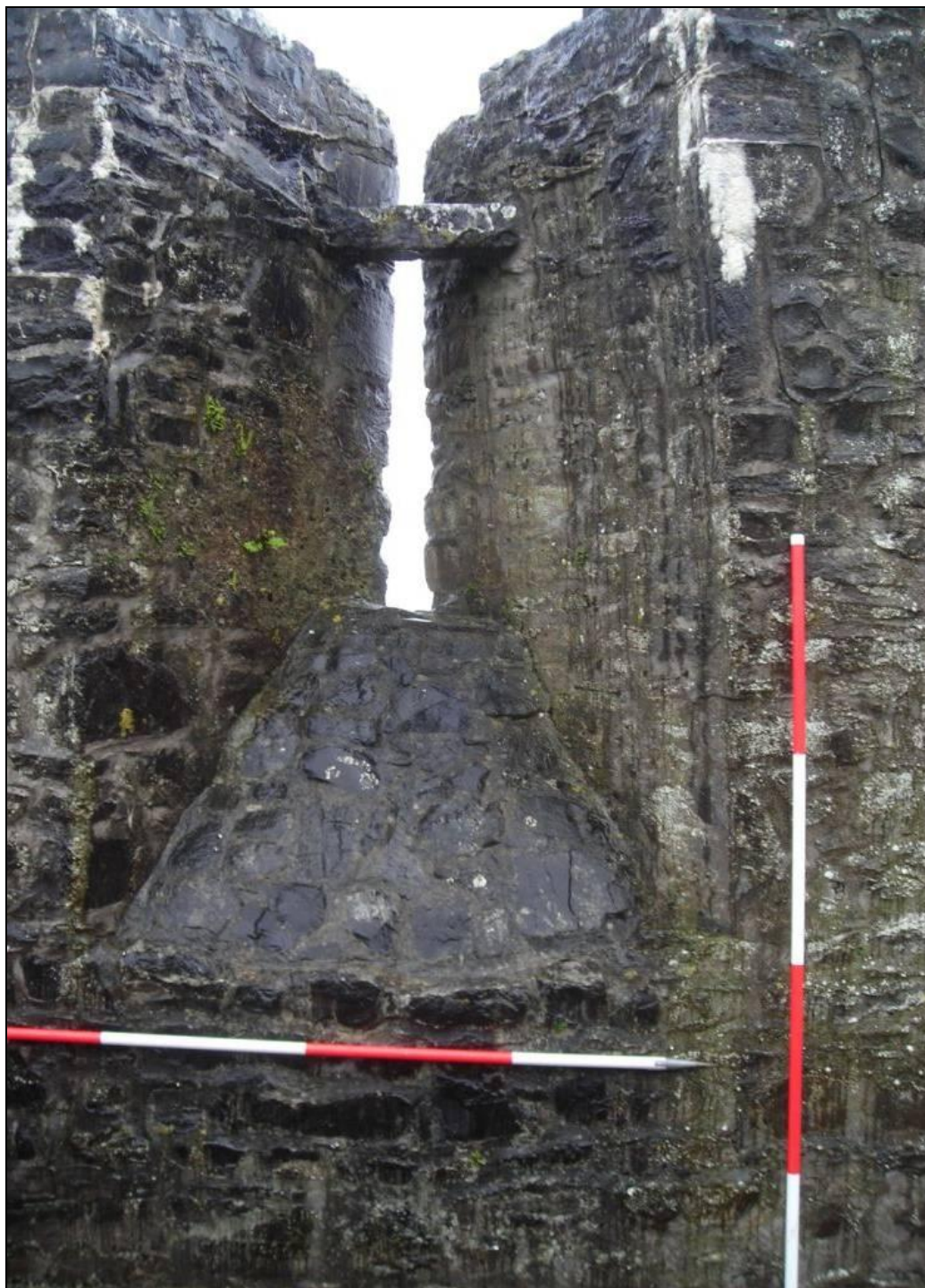
Figure 33: Window in south wall
