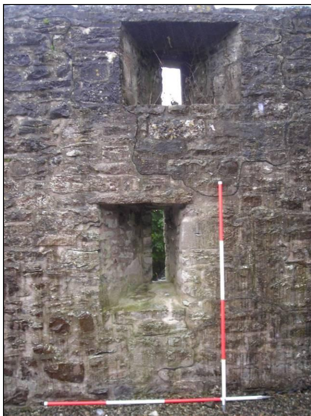
Figure 31: Windows in south wall
