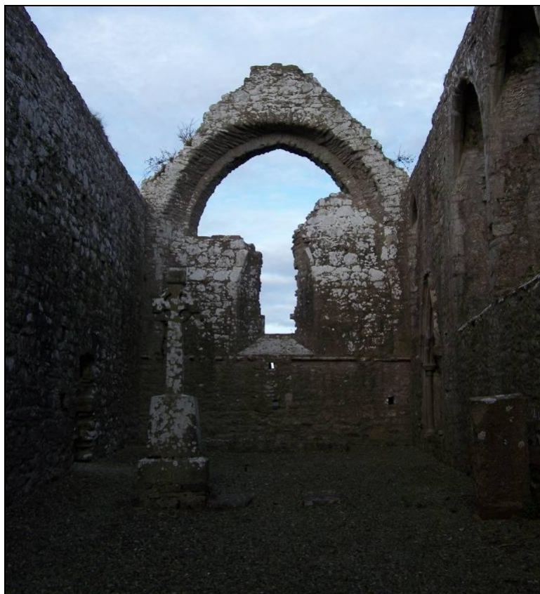
Figure 4: The east window of Burriscarra friary
