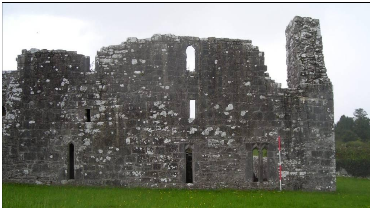
Figure 28: External view of the east range
