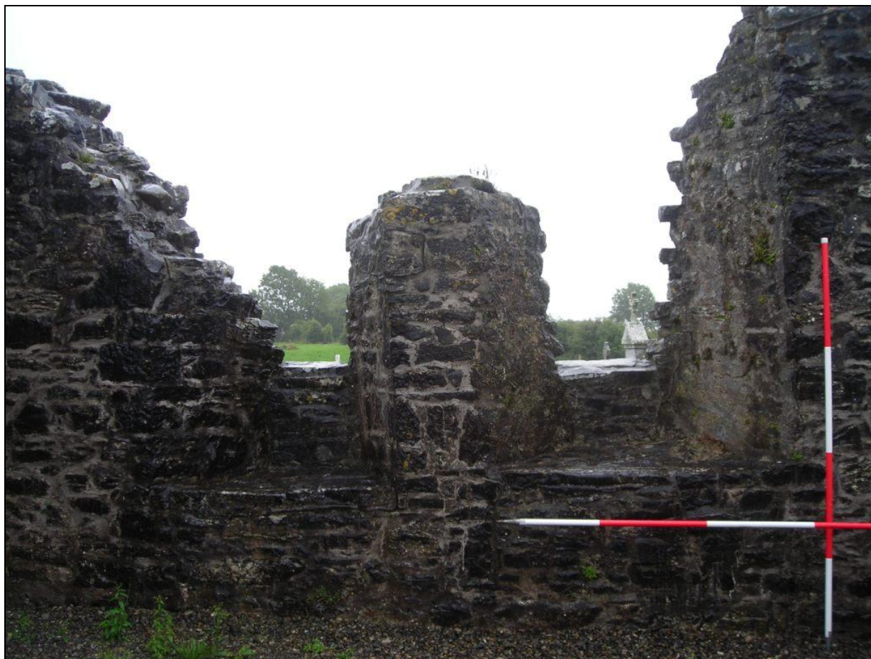
Figure 34: Windows in south wall, towards eastern end of church
