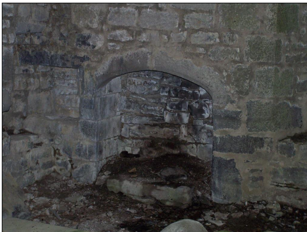
Figure 22: Fireplace in the vaulted room of Burriscarra friary
