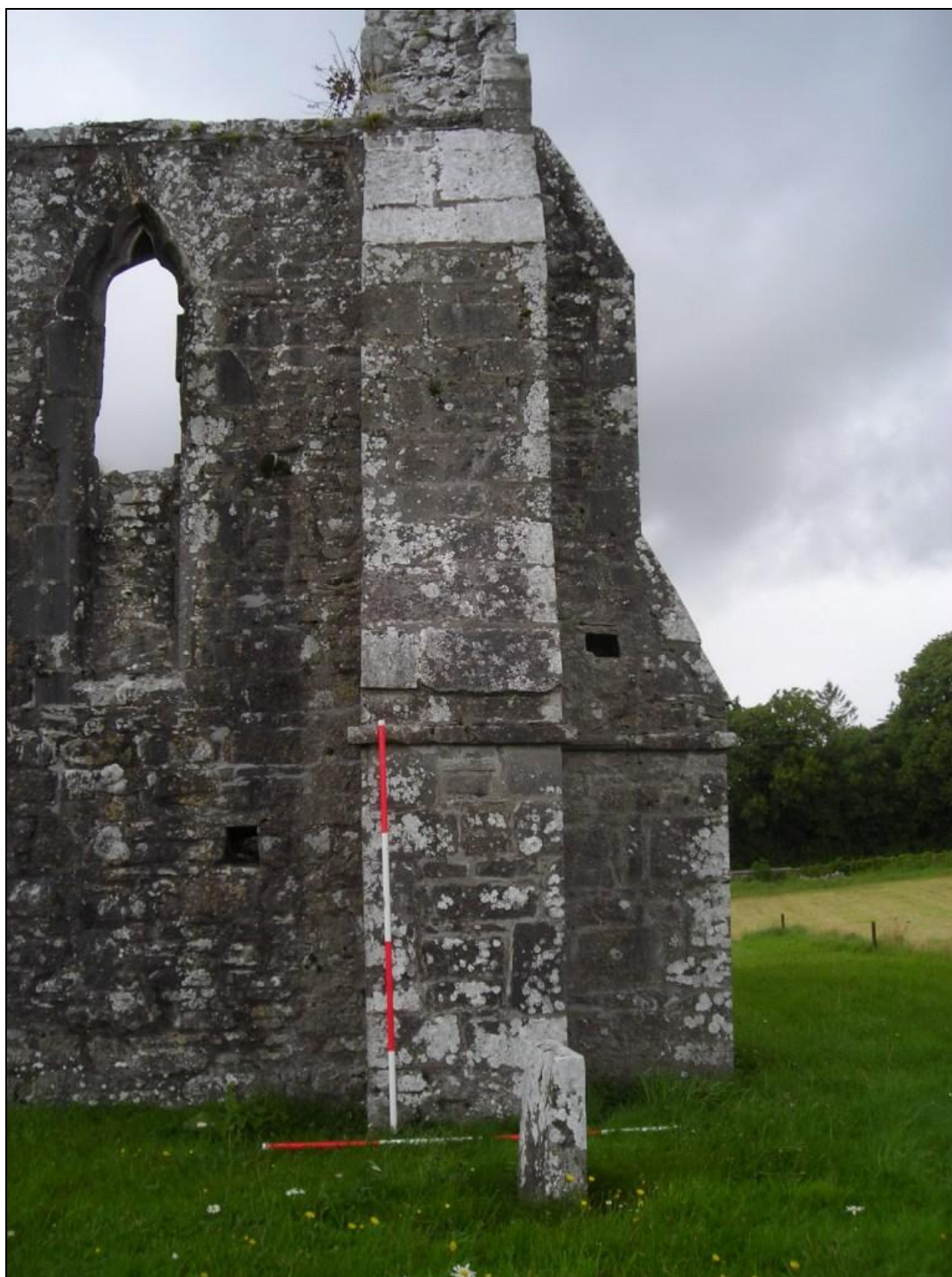
Figure 26: South east corner of friary church
