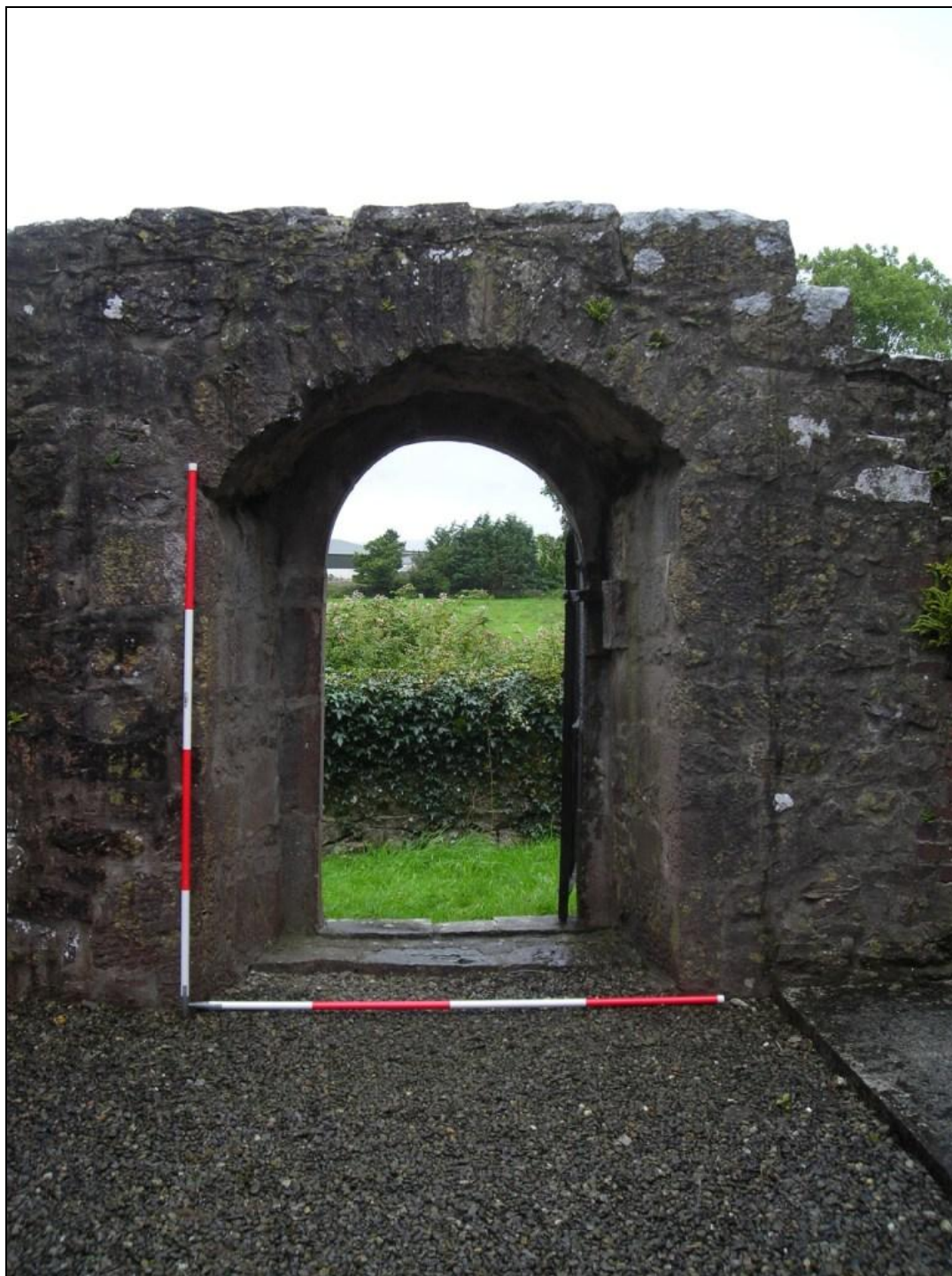
Figure 24: West doorway from the interior
