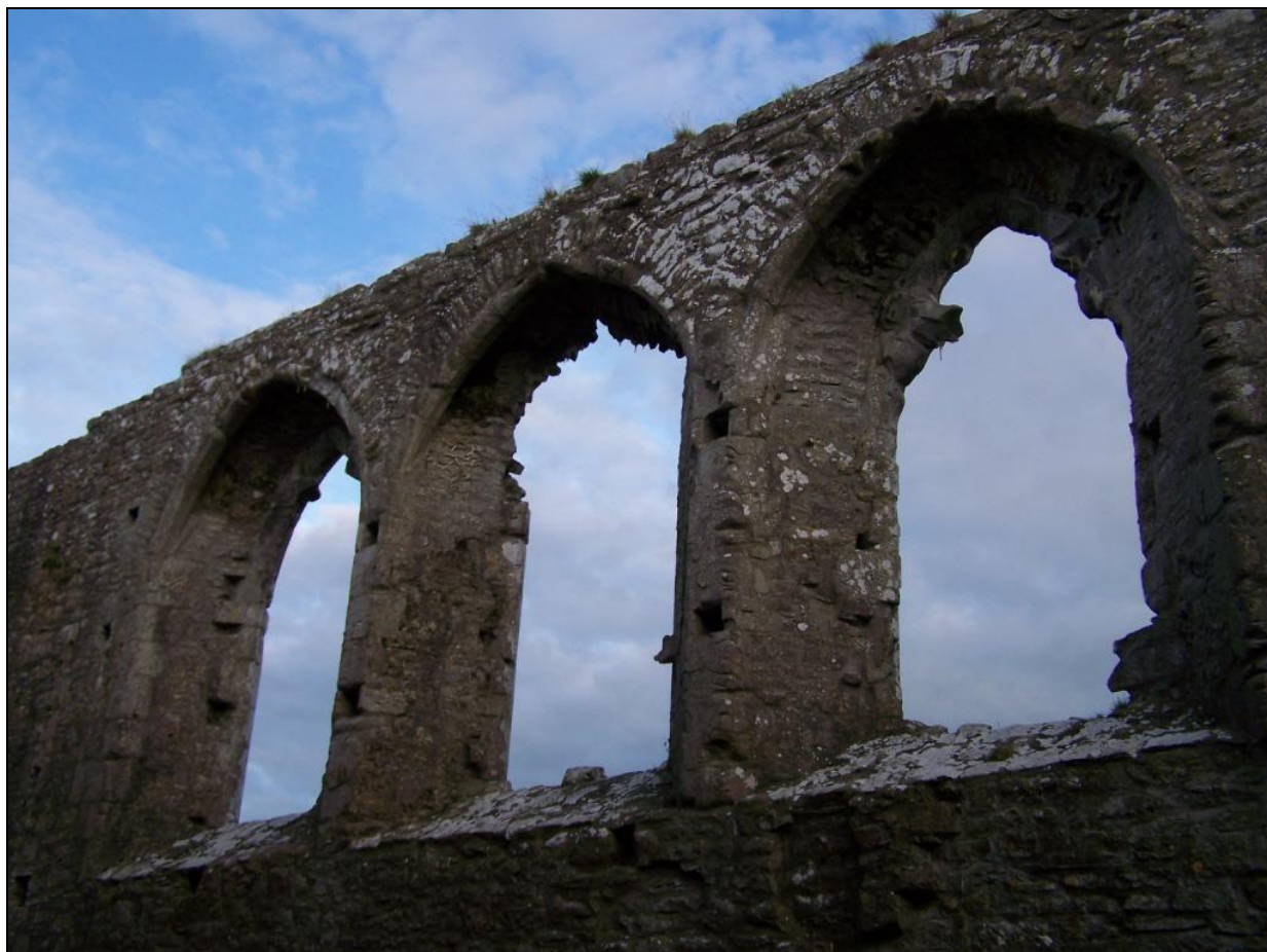
Figure 6: Three windows along the south wall of Burriscarra friary
