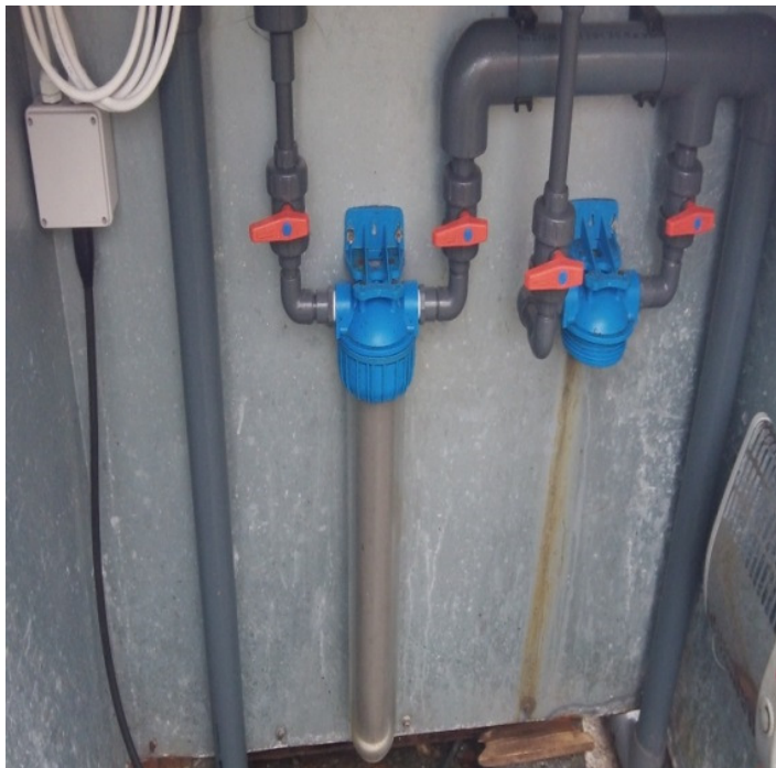
Figure 9. Nest of sieves with outflow pipe releasing filtered water back into water column and Cartridge filter of 80µm
