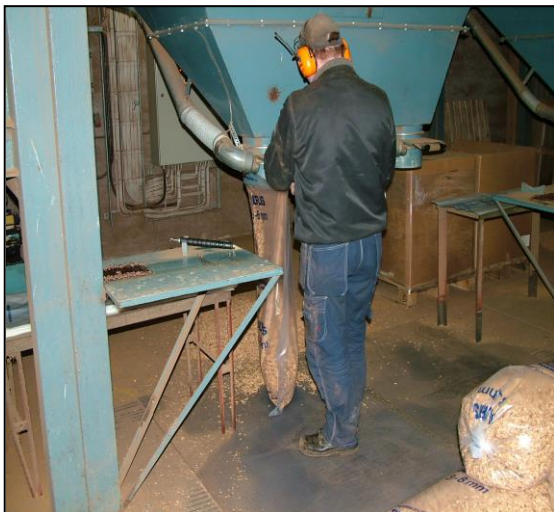
Figure 47: Chip filling station
