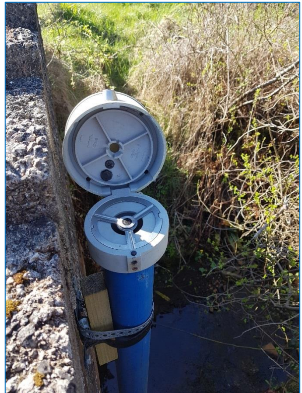
Figure 44: ITC in place (& open) at top of pipe.
