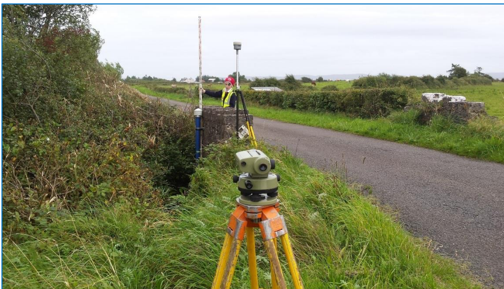
Figure 49: Surveying with a vertical staff along with a dumpy level & tripod to measure the relative height difference between the base of the staff gauge (staff gauge zero) and the TBM.
