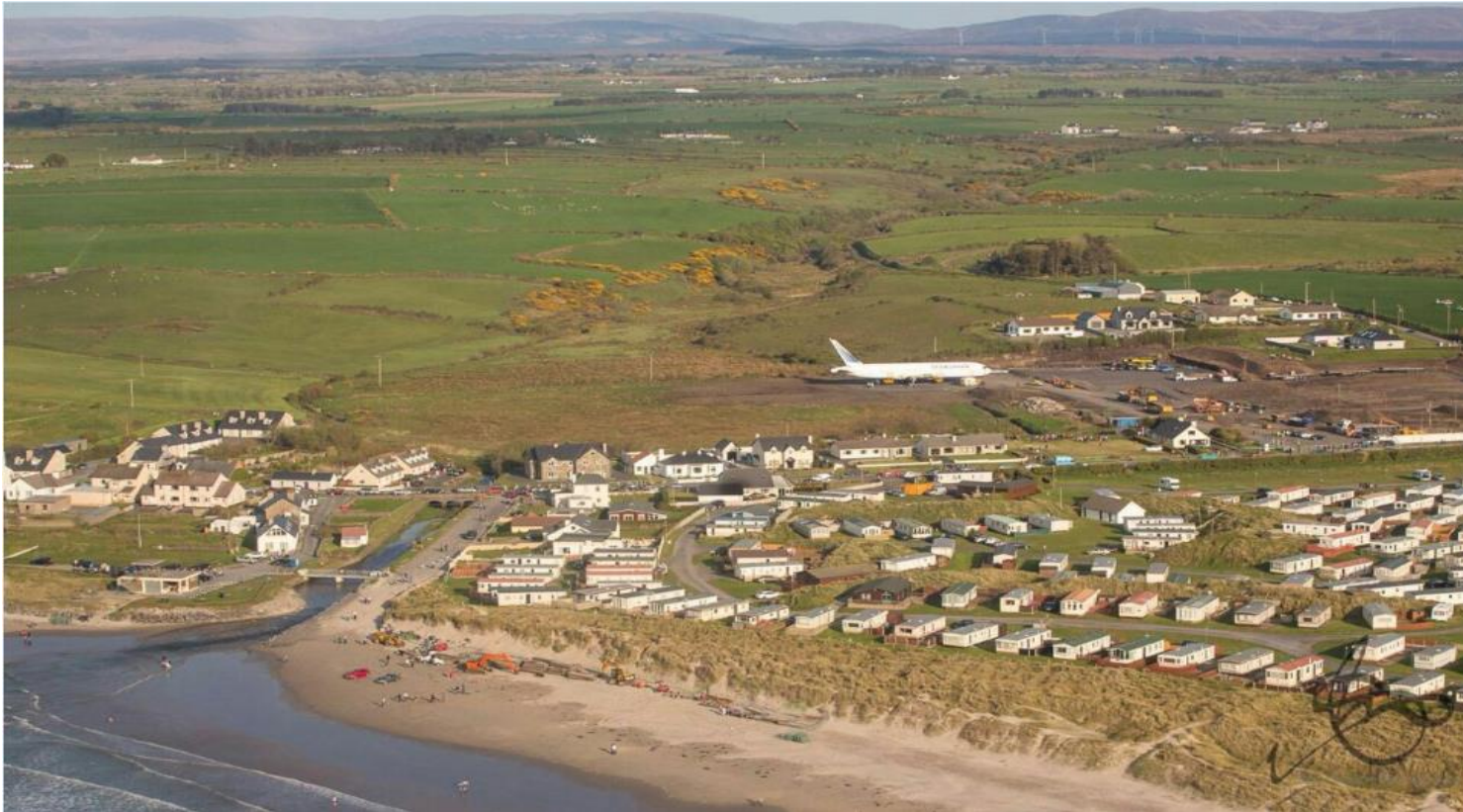
Figure 16: Aerial photograph of beach with river catchment behind.
