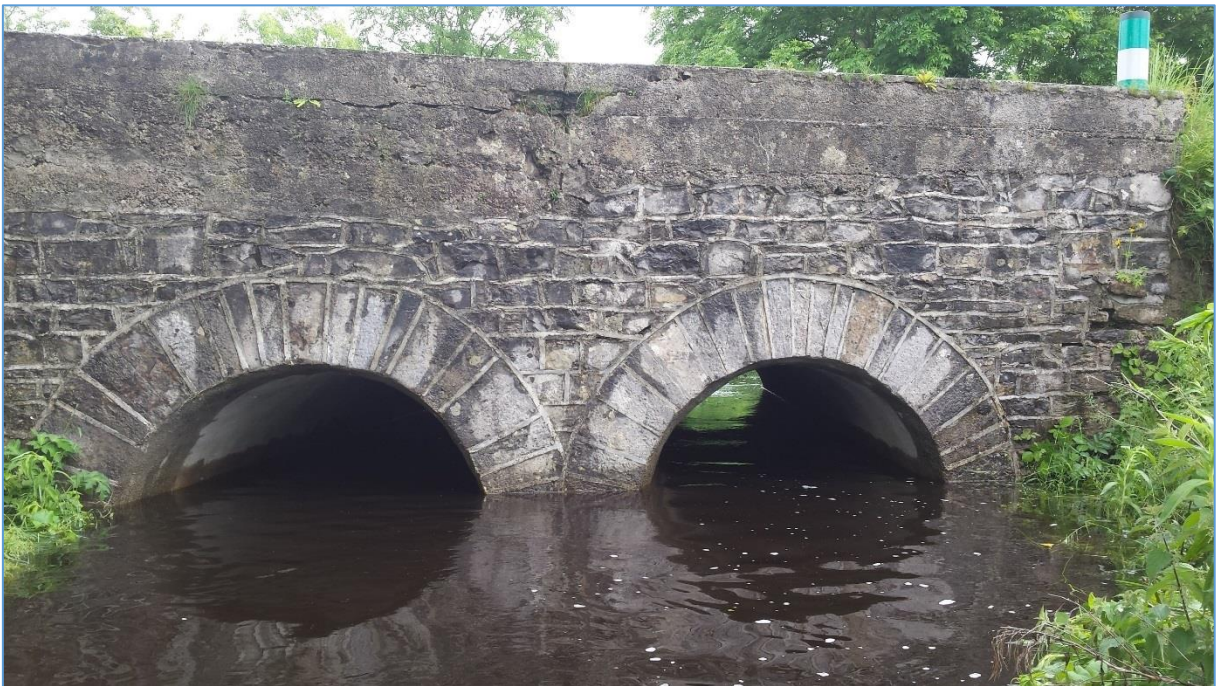
Figure 97: MP5 (Tullylinn Br. – main channel) 14/06/16 after rainfall event
