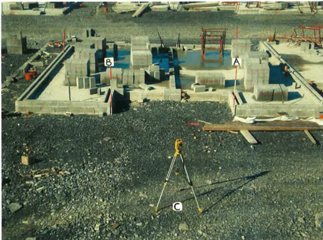
Photograph 4.1 The set up position of the total station.
