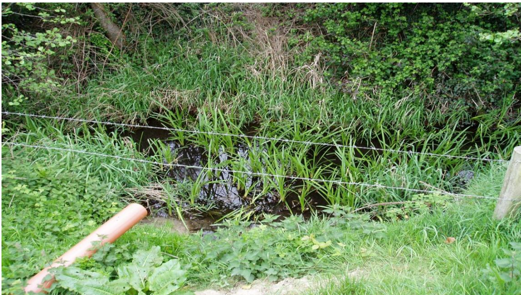
Figure 3.7: The output pipe of pond 12, emptying into the local stream.
