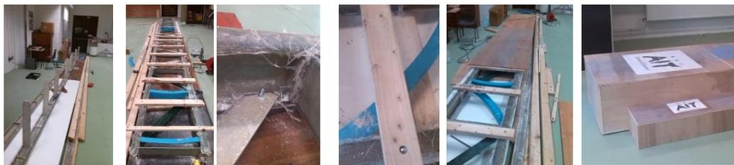
Figure 4: left, lateral bracing construction; 2<sup>nd</sup> left, full bracing near completion; 3<sup>rd</sup> left and centre, GFRP and timber connections; 2<sup>nd</sup> right, decking of bridge; right, 1.5m walk rigid platform.
