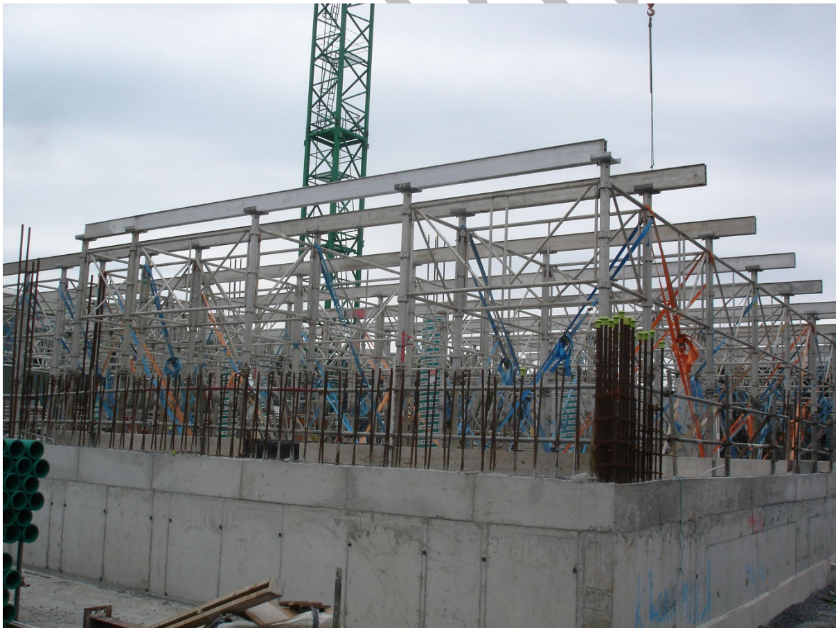
Figure 3 Temporary props prior to erection of lattice girder planks
