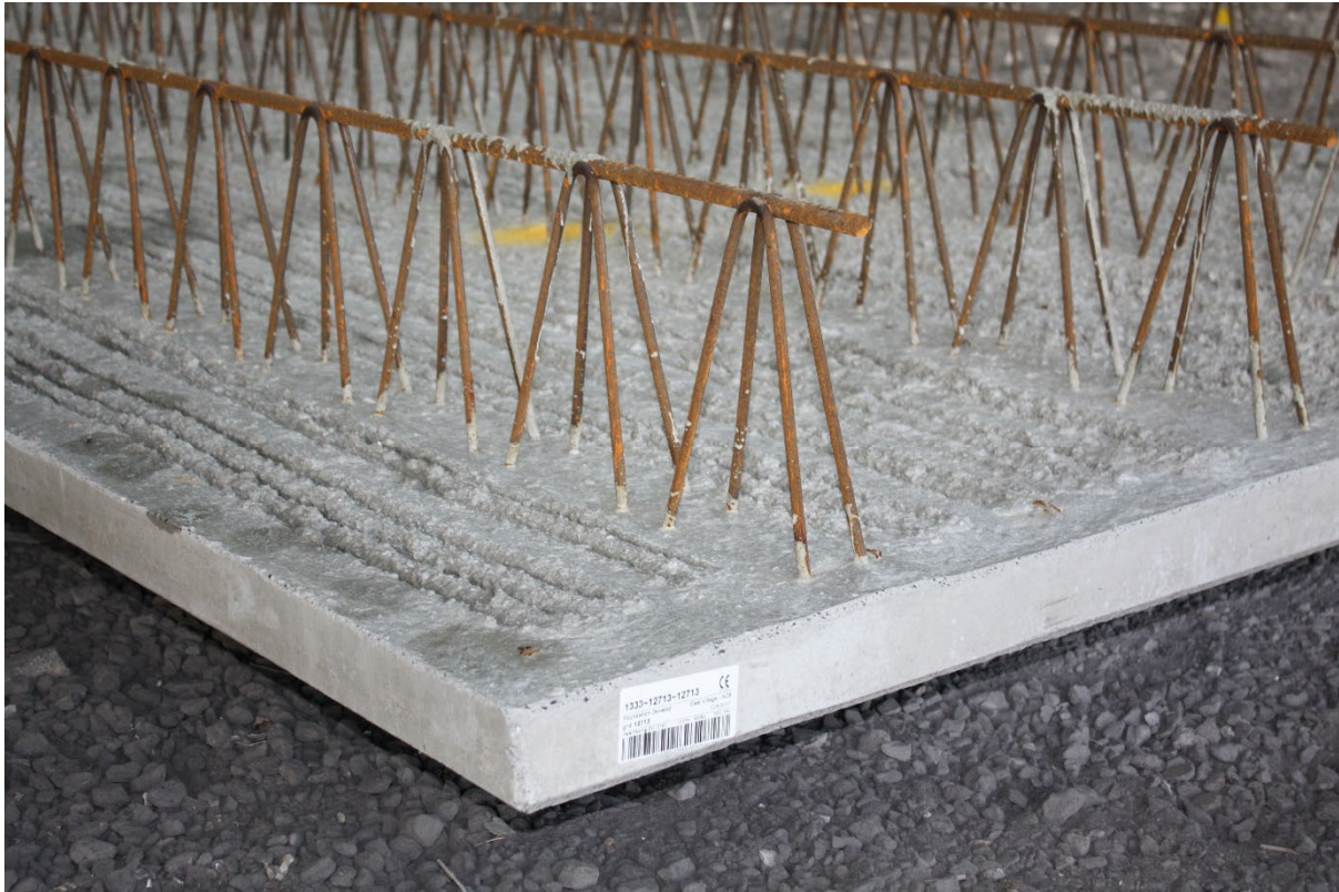
Figure 1 Precast concrete lattice girder plank
