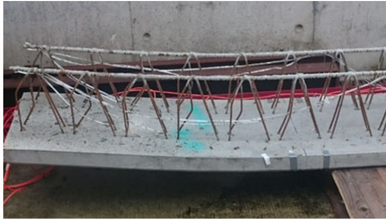
(a) buckling of diagonals (S29-14/07/06_2015)
