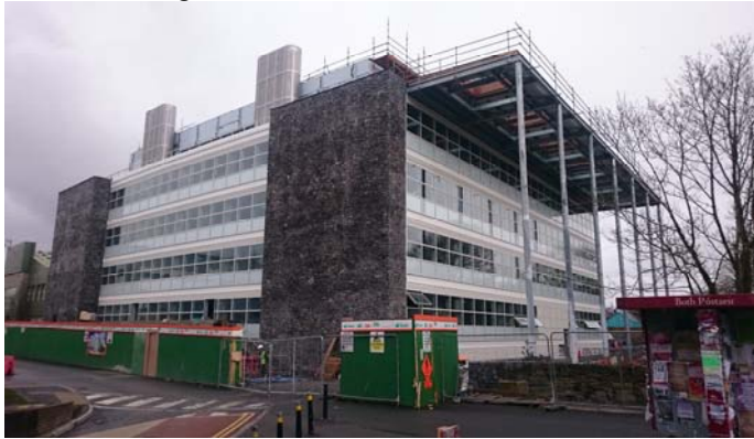
Figure 1. Human Biology Building (under construction)
