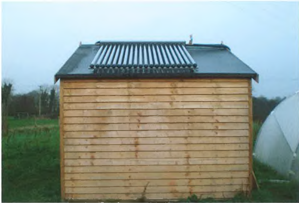
Figure 3.8: Test shed with evacuated tube solar panel attached to south facing roof.
