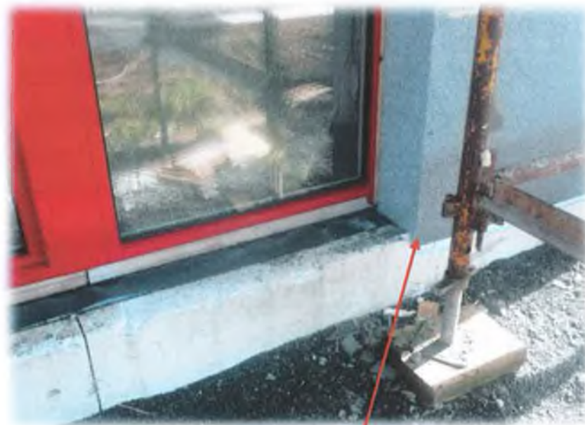
Fig 4.4 Foundation Insulation joins Wall insulation
