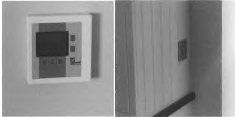
Figure 4.10 Ventilation controls and boost switches
