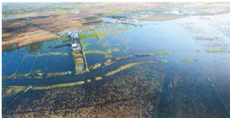
Figure 3.13 – Flooding Along the N84 (Headford Rd), 22/Nov/2009
