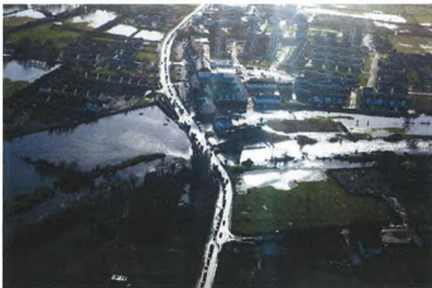
Figure 3.15 – Flooding in Claregalway, 22/Nov/2009
