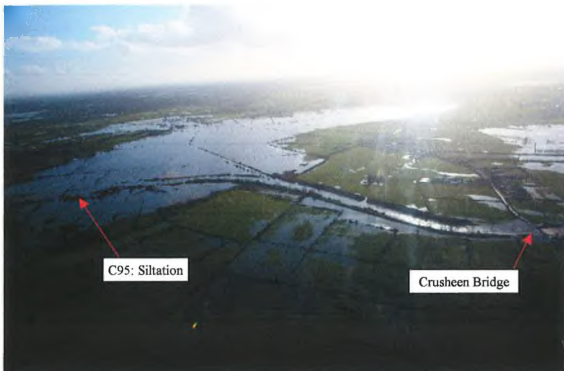
Figure 7.9 – November 2009 Flood Event Upstream of Crusheen Bridge, Looking South
