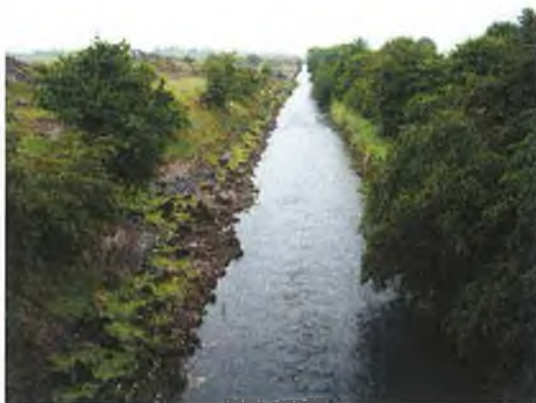
Figure 7.4 – Canalised Channel, Looking d/s from N17 Bridge South of Tuam
