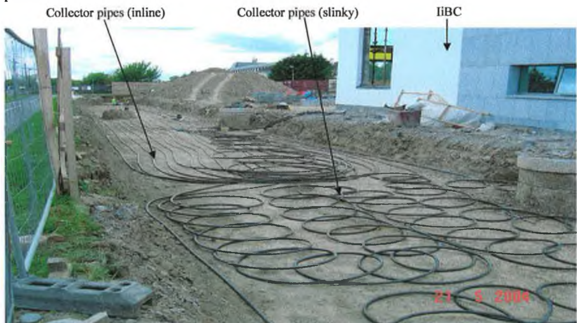
Figure A.12(a) Photograph of the GSHP's collector pipes during installation.
