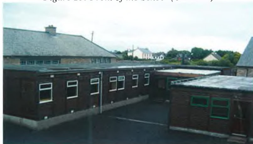
Figure 14: Prefabs in the School
