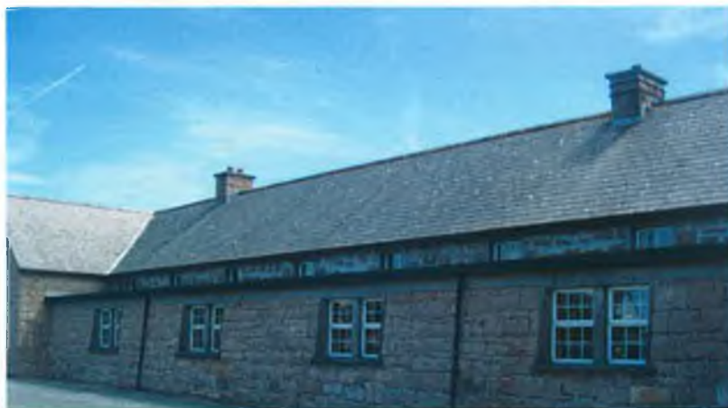
Figure 13: Front of the School (Old Part)
