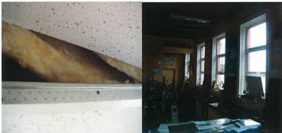
Figure 25: Insulation in Prefabs and Double Glazed Windows in the Main Building
