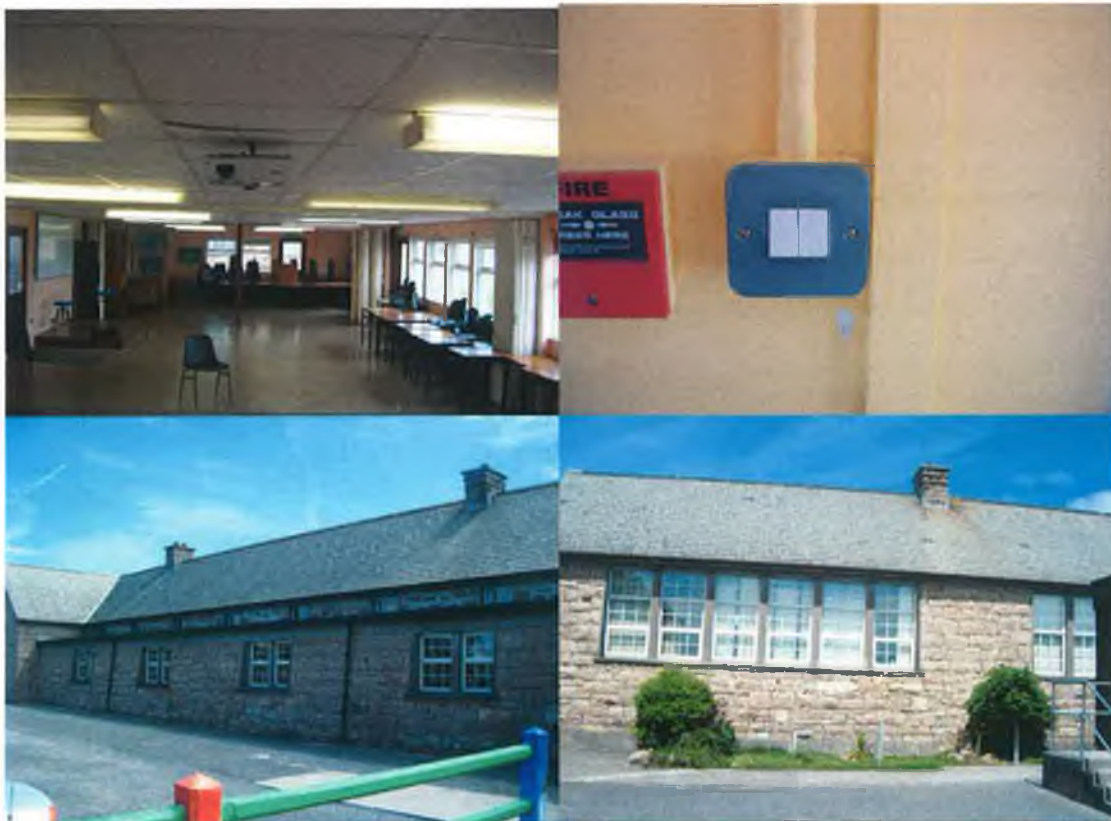
Figure 16: Lighting, Lighting Control and Natural Light Available
