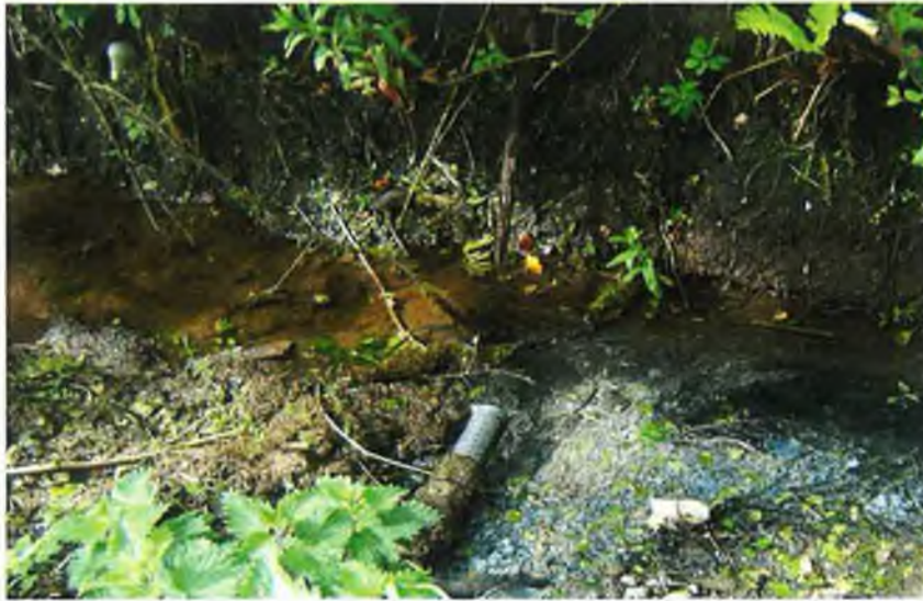
Plate 8.5: Discharge of partially treated effluent into stream (O'Rourke,2012)
