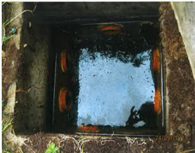
Plate 8.15: Evidence of high water table or blocked percolation (Cooney, 2012)
