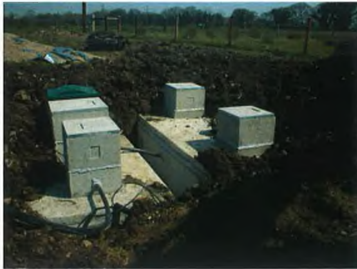
Plate 8.9: Example of risers used to raise the level of the inspection covers to ground level
