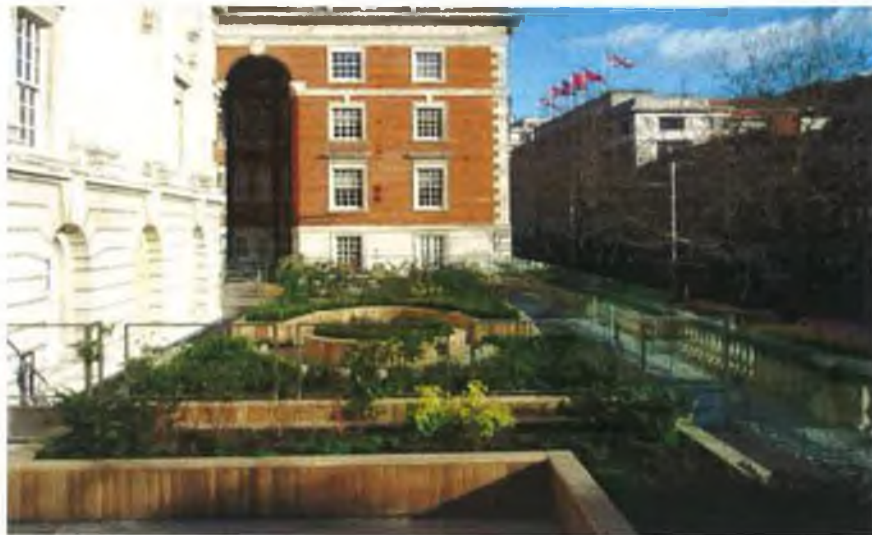
Figure 16: Intensive Green Roof Case Study – Hornton Court, UK ©Bauder
