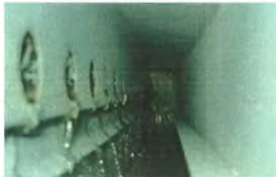
Figure 30: Hidden gutter and parapet ©GoGreenRoof
