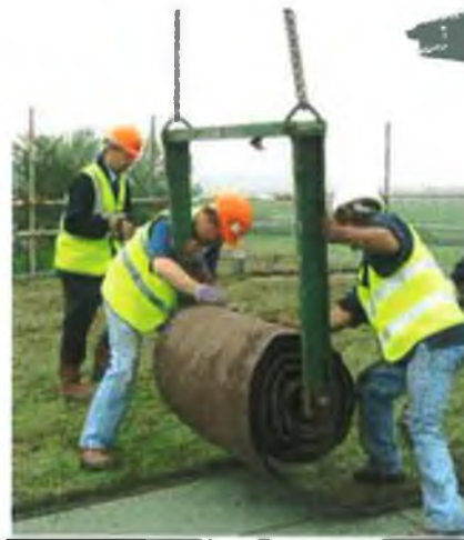
Figure 19: Sedum mat being installed onto roof in large rolls ©Bauder
