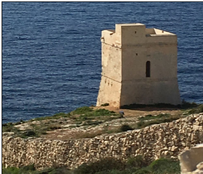
Figure 2.12. Hamrija Tower on the south-west coast of Malta. The de Redin towers are a little stockier than the Lascaris towers. Photograph by James Bonsall.
