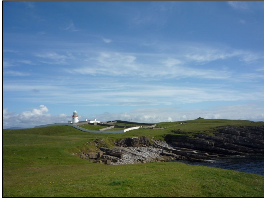
Figure 4.54. St John's Point lighthouse, County Donegal, looking north-east. St John's Point Signal Station was located in the distance, at the right of the shot, in front of the Look Out Post (L.O.P 70) on top of the conical mound.
