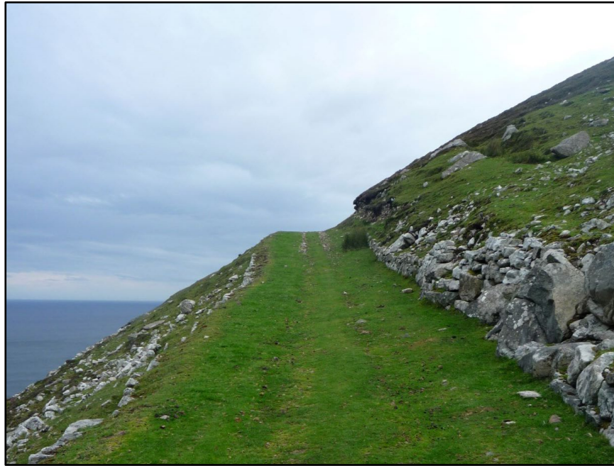
Figure 4.37. A section of the road which leads to Glen Head Signal Station, County Donegal. This track utilises multiple switch backs as it climbs the steep hillside to the north of Glencolumbkille and has clearly been carefully designed and executed.
