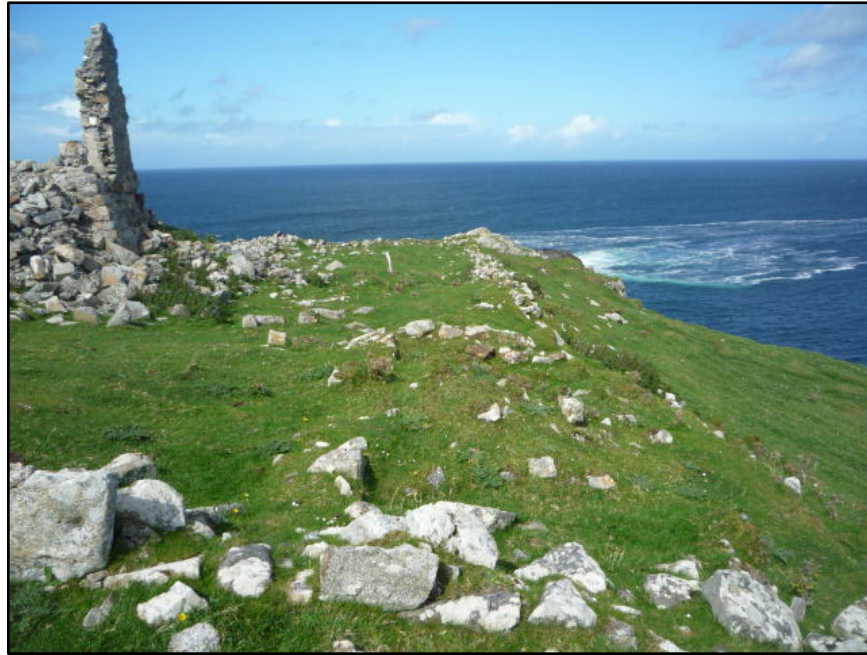
Figure 4.33. The building foundation in the south-east corner of the enclosure at Melmore Head Signal Station, County Donegal, looking north.
