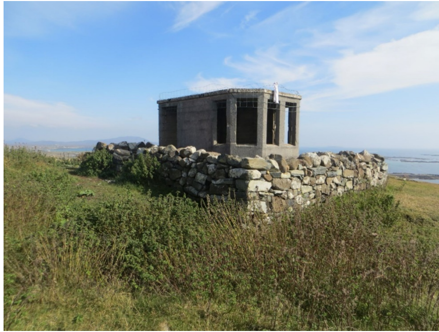
Figure 4.47. The Look Out Post (L.O.P. 53) at the west of Bunowen More Signal Station, County Galway, looking south-east. An encased benchmark is located on the roof of this structure.
