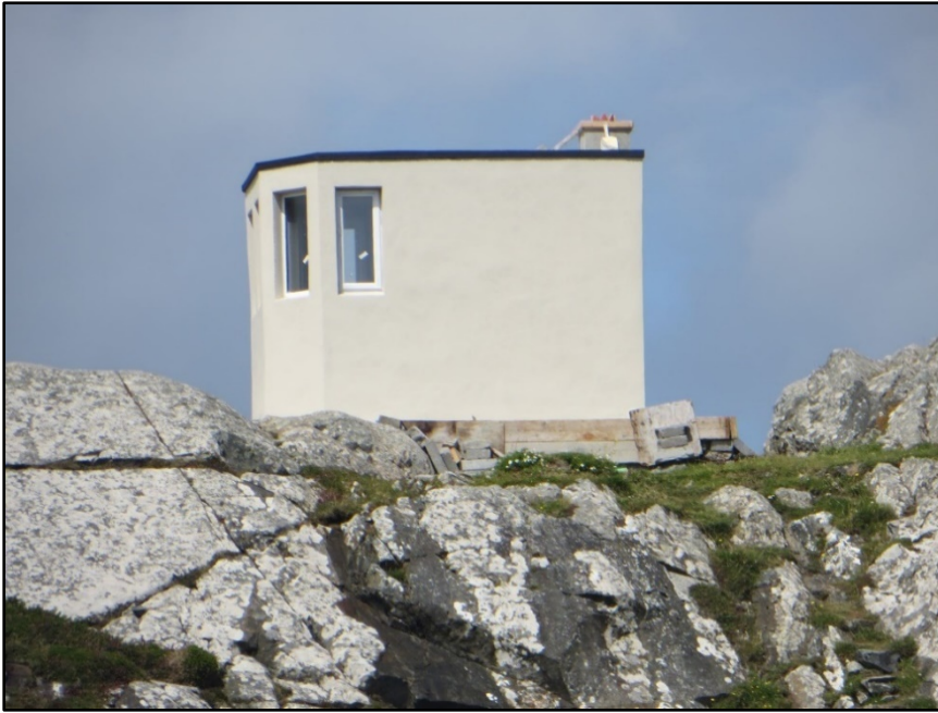
Figure 4.49. The renovated Look Out Post (L.O.P. 51) on Lettertmullan Island, County Galway, overlooking Golam Head Signal Station.
