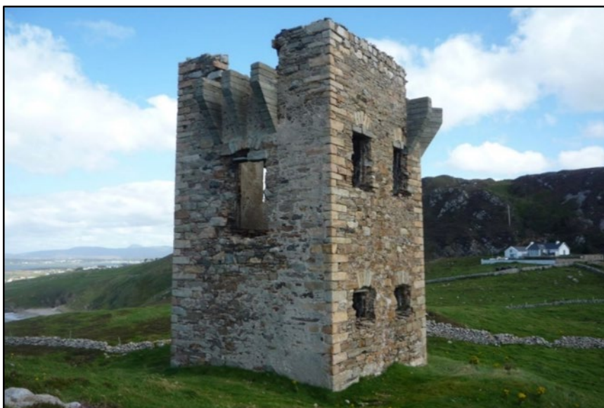
Figure 1.4. Crohy Head signal station, County Donegal, an example of a well-preserved site today. The signal towers were square buildings, measuring around 5.8 m (19') across and had heights of between 10 m (32' 10'') and 12 m (39' 4'').
