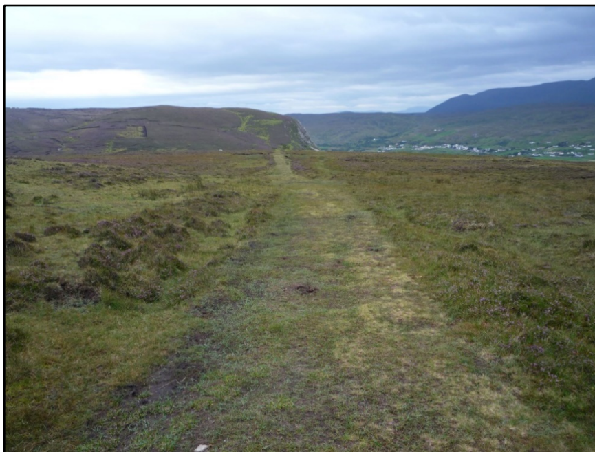
Figure 4.38. The road to Glen Head Signal Station, County Donegal. After climbing the steep hillside, it crosses a flat plateau, shown here. Even in this section the road appears to have been built with a proper roadbed.
