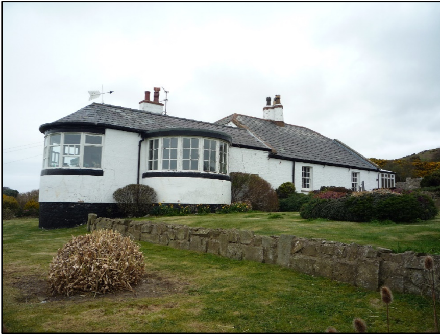
Figure 2.22. Voel Nant Telegraph Station, constructed 1841.
