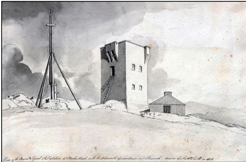
Figure 1.3. A rare contemporary illustration showing Malin Head signal station in County Donegal (TCD MS 942/1: 24). The caption reads 'View of the Naval Signal Port Station at Malin Head with the guardhouse and barrack drawn by Sir Wm Smith in 1808.' Smith was the engineer in charge of constructing several of the signal stations in Northern Donegal. The image shows the signal mast, the signal tower and a smaller barrack building which was used for accommodation whilst the signal tower was being constructed.
