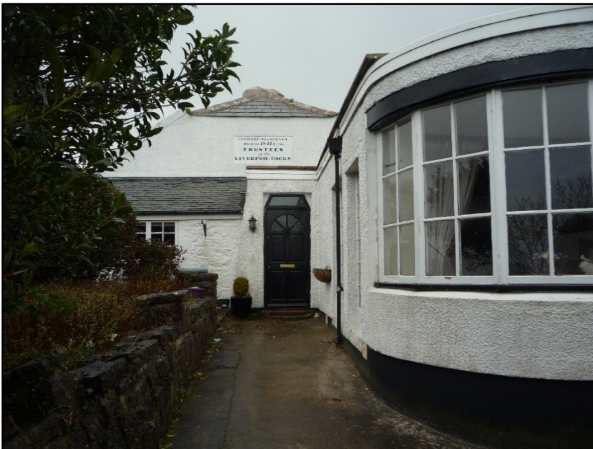
Figure 2.23. Llysfaen Telegraph Station, constructed 1841.
