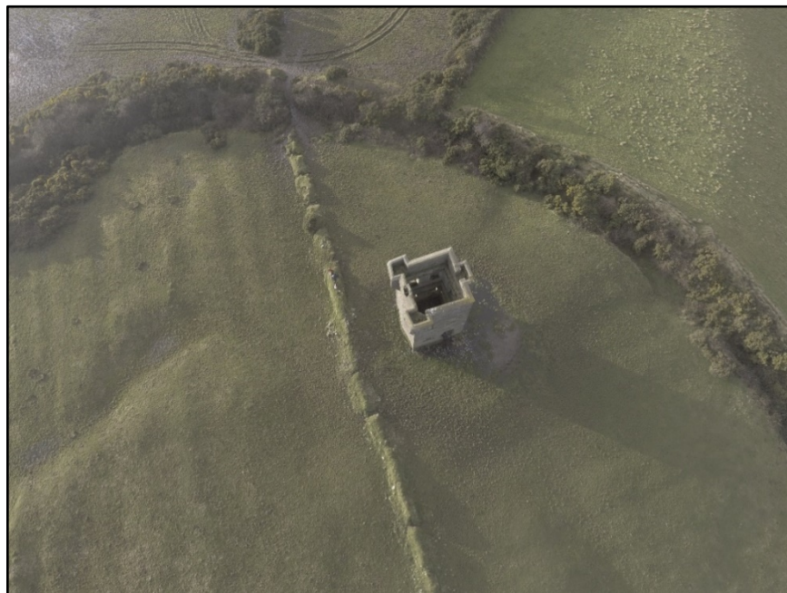
Figure 6.2. Drone photograph of the signal tower at Carrowmably Signal Station, County Sligo, showing details about the upper portion of the tower that would be difficult to observe directly from ground level (Photograph courtesy of Sam Moore).
