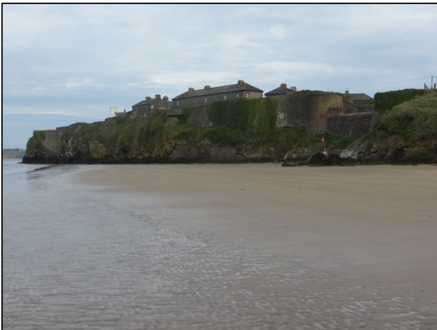
Figure 2.2 Duncannon Fort, County Wexford, from the adjacent beach, looking north.
