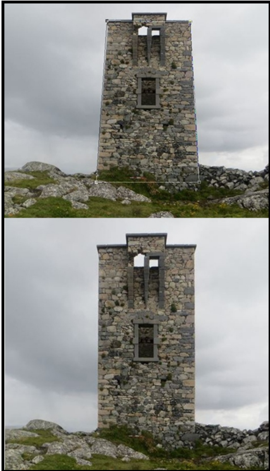
Figure 3.7. Perspective correction south-west wall of the signal tower at Golam Head Signal Station, County Galway, in PaintShop Pro X8 . The corners of the perspective correction tool are dragged over the corners of the building (top), and the software makes the required adjustments (bottom).
