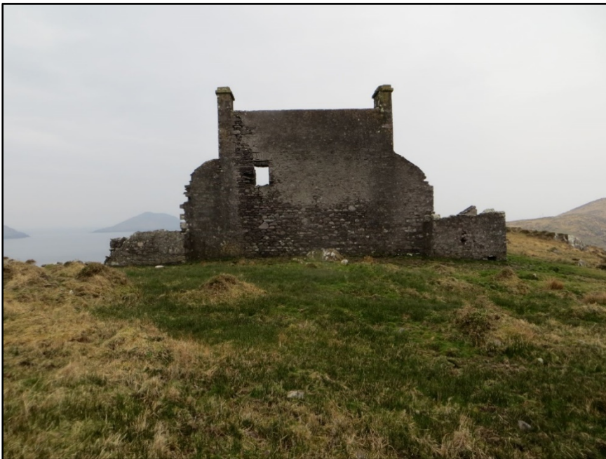
Figure 4.64. The imposing rear wall of the two storey building at Hog's Head Enclosed Barrack, County Kerry, looking west. This wall formed part of the perimeter along the eastern side of the enclosure.
