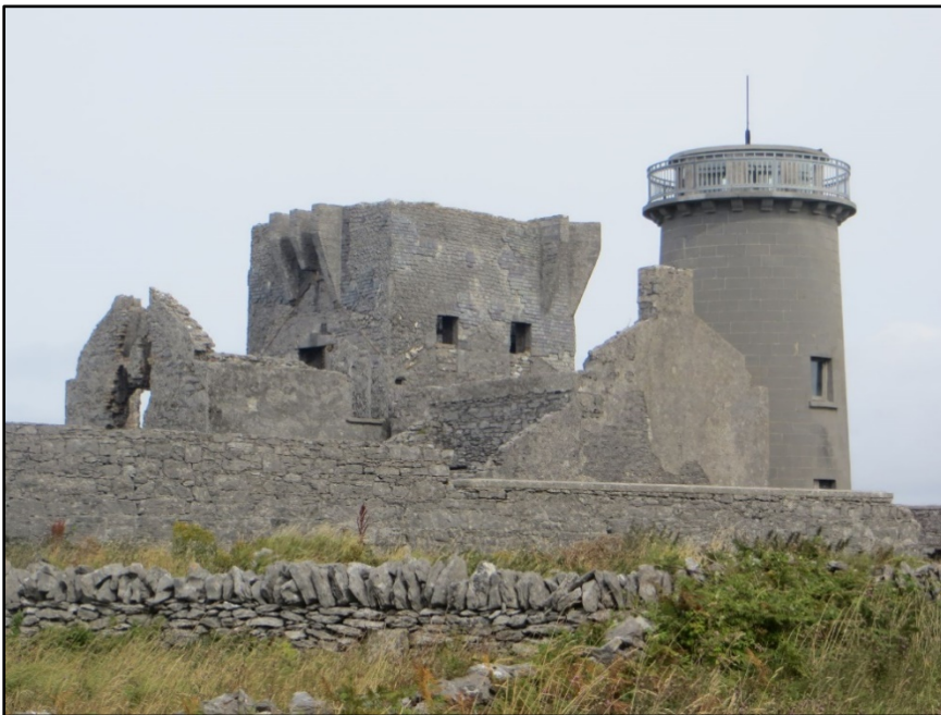
Figure 4.42. Inishmore Signal Station, County Galway, showing the secondary additions to the signal tower and the later lighthouse in the back ground, looking north.
