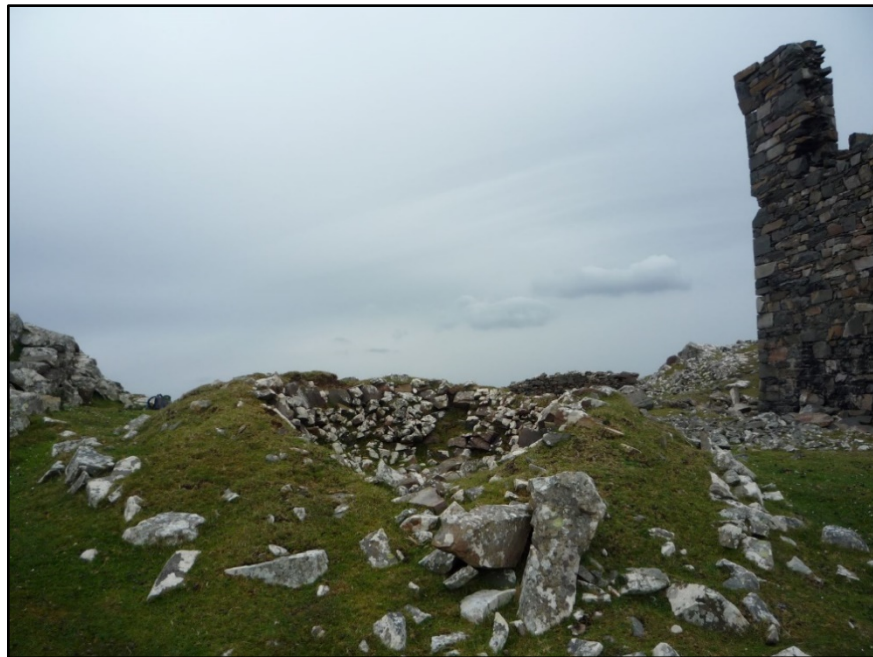
Figure 4.36. The lime kiln at Clare Island, County Mayo, looking north-east with part of western side of the signal tower in the background.
