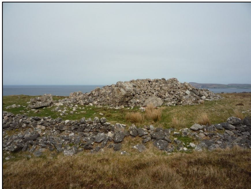
Figure B.69. The south-west side of the signal tower at Tower Hill Signal Station, with the enclosure wall in the foreground and Benwee Head visible in the background. The fallen bartizan is visible in the centre of the photograph.
