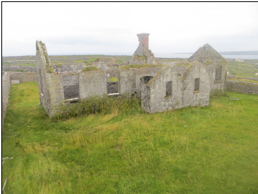
Figure A.12. View of the schoolhouse, looking west. The double entrance is in the foreground, projecting from the front wall of the building, and the brick chimney can be seen extending from the peak of the central gable.
