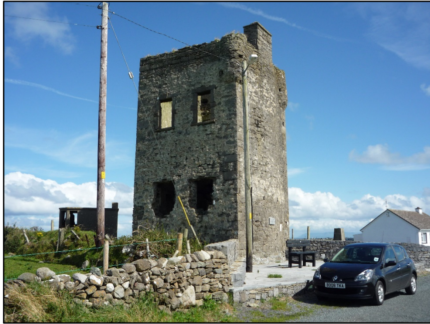
Figure C.18. View of the south-west corner of the signal tower at Rathlee Signal Station.
