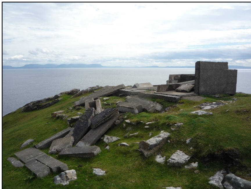
Figure D.14. The badly collapsed remains of L.O.P. 71, located to the south of the signal tower at Carrigan Head Signal Station.
