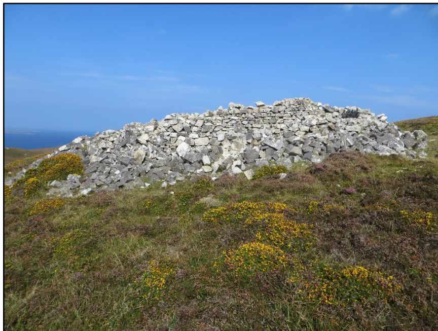
Figure A.96. View of the southern wall of the collapsed adjacent building, looking north.
