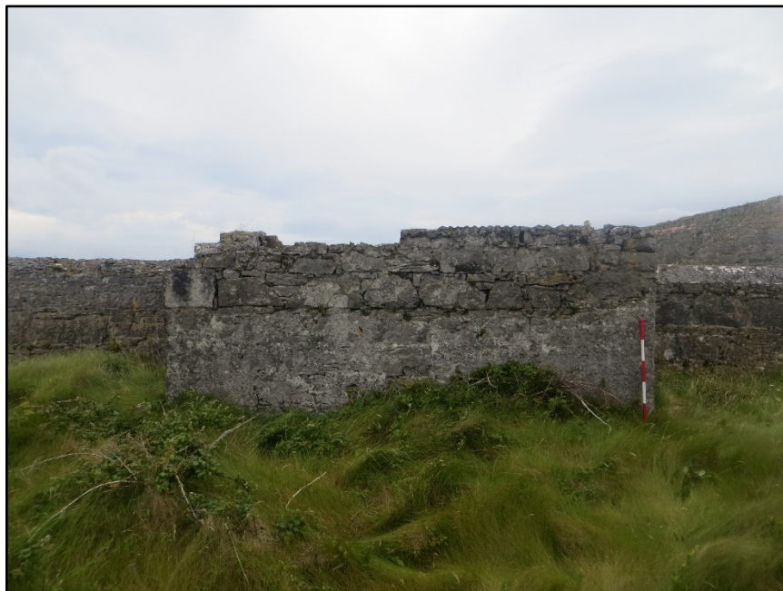
Figure A.14. The north-east front wall of the toilet block.
