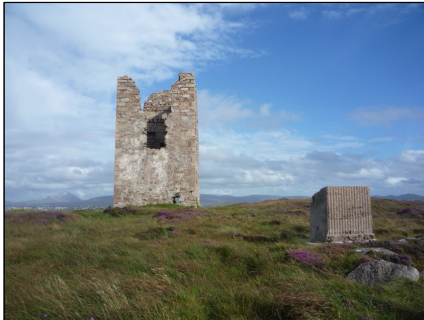
Figure D.72. View of the north-west wall of the signal tower at Mullaghderg Hill Signal Station, with the concrete pillar in the foreground.
