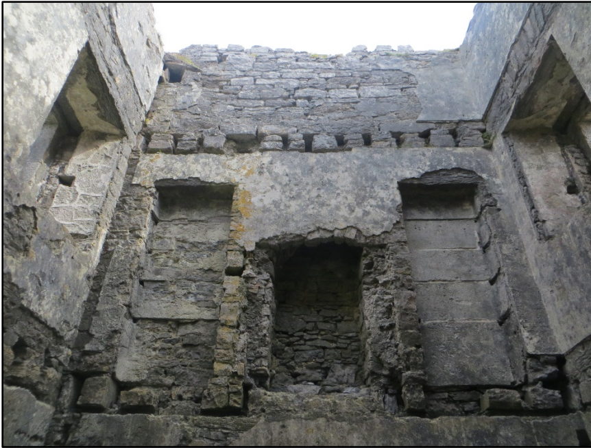
Figure A.30. The upper part of the internal wall face of the north-east wall, showing the central fireplace flanked by alcoves bearing the impressions of shelves. The row of joist holes of the attic level run above the tops of the alcoves. In the top left the edge of the diagonal stone marking the entrance to the north bartizan can be seen.
