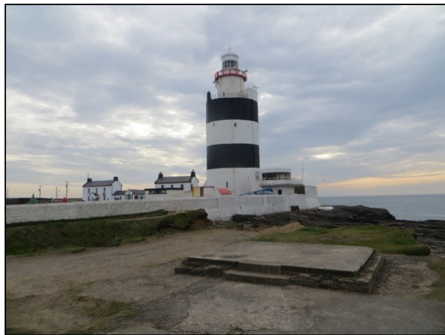
Figure E.11. The concrete slab foundation of Look Out Post 16, located to the south of the enclosure around the lighthouse, looking east.
