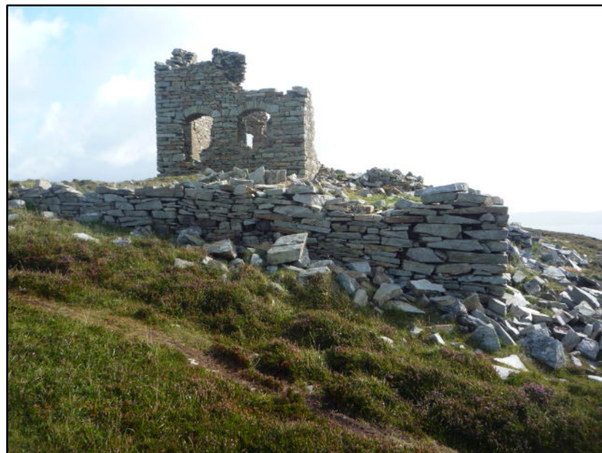
Figure D.90. The external face of the west wall of the signal tower at Horn Head Signal Station, with the south-west corner of the enclosure in the foreground.
