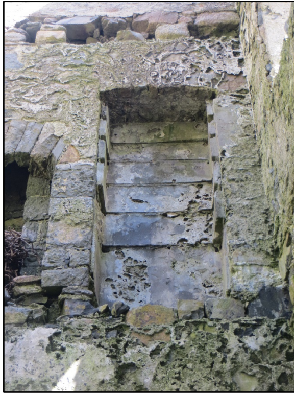
Figure A.61. Detail of the east first floor alcove on the north-east wall, showing the impressions of shelves in the render.
