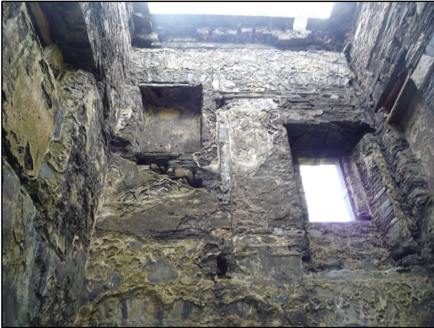
Figure D.29. The upper portion of the internal face of the north-west wall of the signal tower at Carrigan head Signal Station, showing the heavily modified first floor windows.
