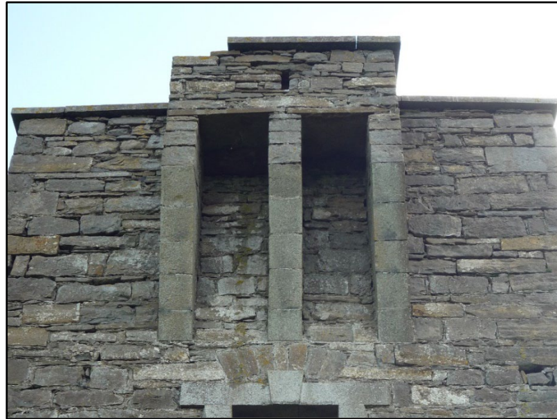
Figure C.49. Detail of the machicolation over the door on the south wall of the signal tower at Carrowmably. Note the gun-loop in the centre of the south wall of the machicolation.
