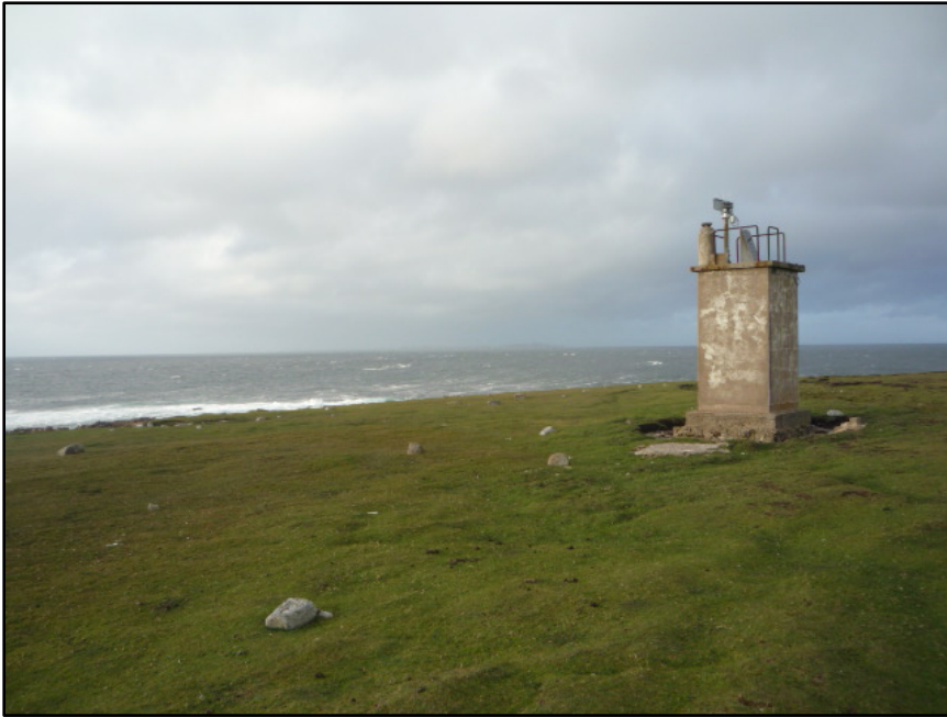
Figure D.84. The automated weather station at Bloody Foreland, to the north of the location of the demolished Bloody Foreland Signal Station.
