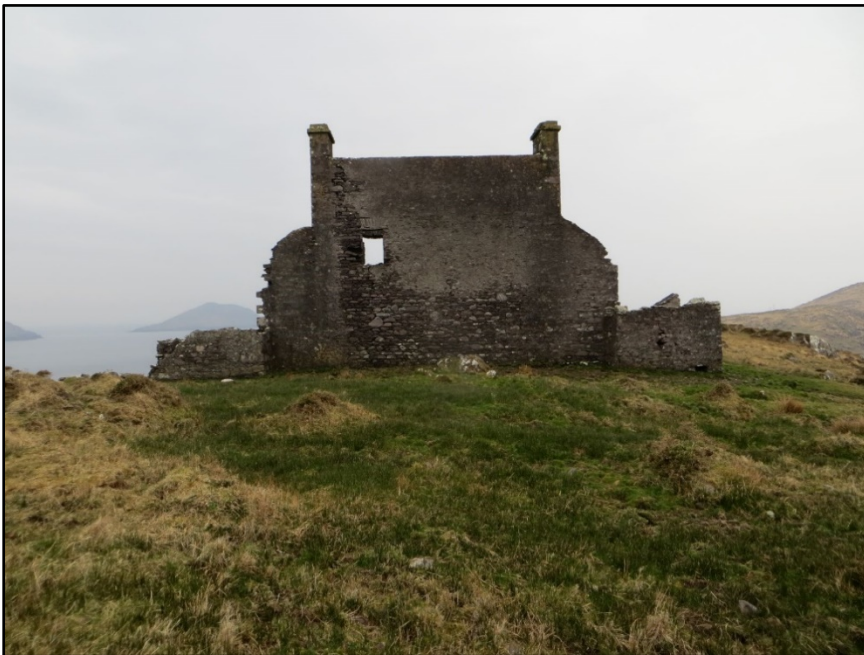
Figure G.3. The imposing rear wall of the two storey building at Hog's Head Enclosed Barrack, County Kerry, looking west. This wall formed part of the perimeter along the eastern side of the enclosure.
