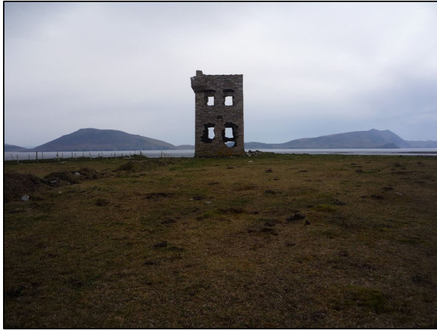
Figure B.53. The north wall of the signal tower at Glash Signal Station. Achill Island can be seen in the background.
