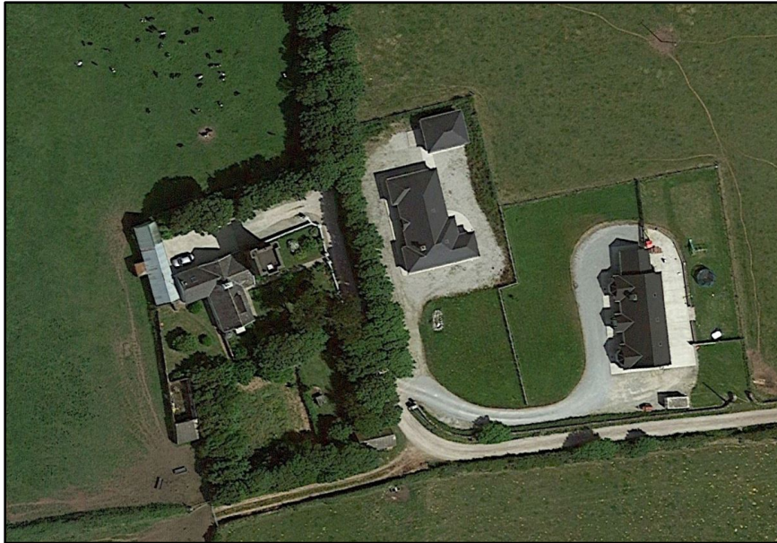
Figure F.5. Aerial view of Ballynacotter signal tower with the large residence attached to its western side. (Photo courtesy of Google Earth).
