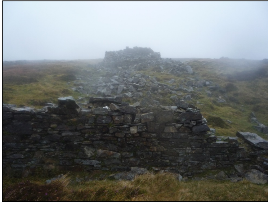
Figure B.84. View of Glinsk Signal Station, looking north, with the wall of the enclosure in the foreground.
