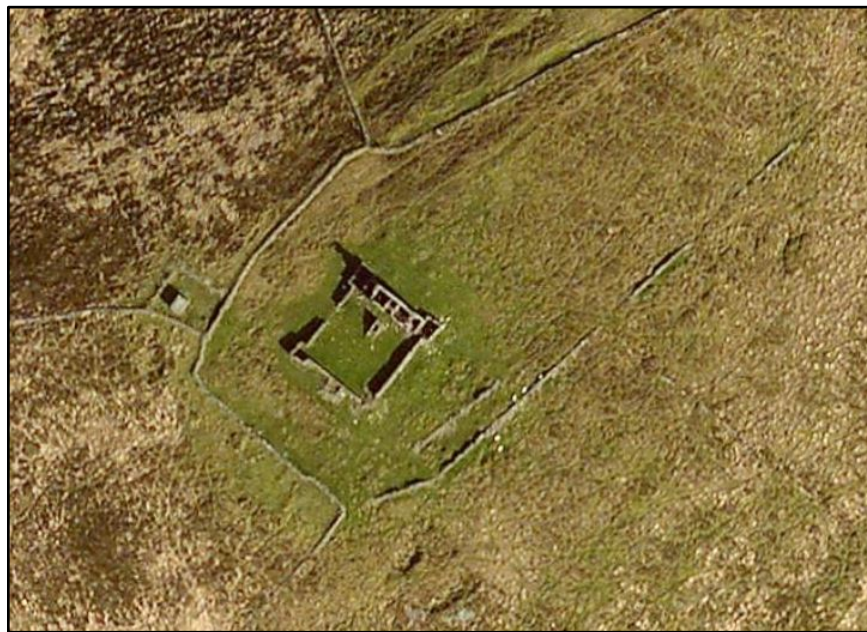
Figure G.9. Aerial photo of Bolus Head Enclosed Barracks, County Kerry (Photo courtesy of Google Earth).
