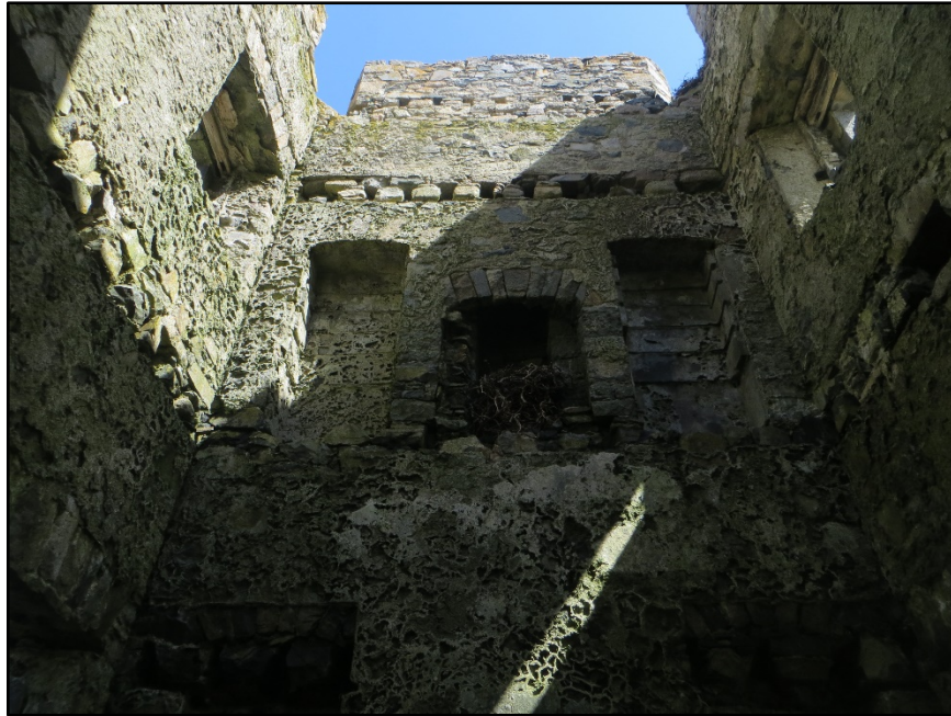
Figure A.57. The upper portion of the internal face of the north-east wall, showing the central fireplace flanked by two alcoves with the impressions of shelves, the joist holes of the attic level, the stepped parapet with joist holes for the roof, and the entrances to the bartizans.
