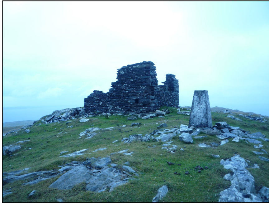
Figure B.8. View of the base of the signal tower at Inishturk Signal Station, looking south-west, with the trigonometry pillar in the foreground.
