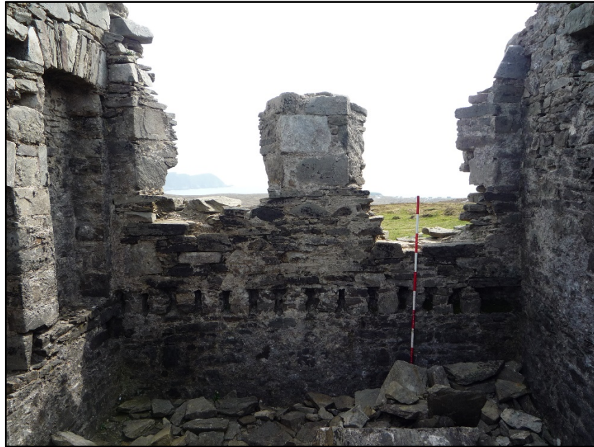
Figure B.38. View of the internal face of the south wall of the signal tower at Saddle Hill Signal Station.
