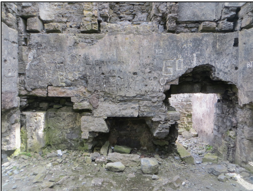
Figure A.31. The lower part of the internal wall face of the north-east wall, showing the top of the central fireplace flanked by alcoves, the right hand alcove having been opened up into a ground level entrance. The extent to which the ground floor level has been infilled is clearly visible.
