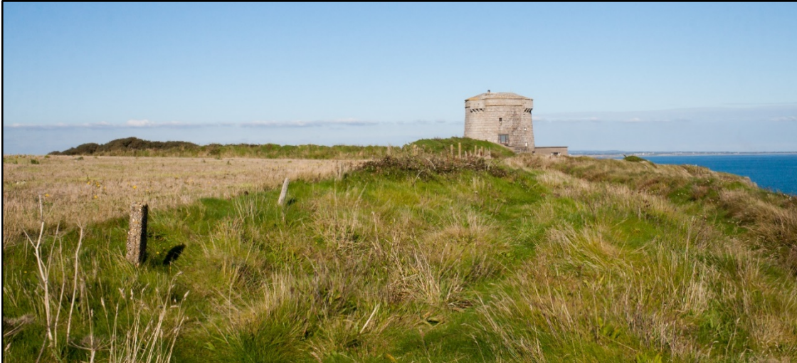
Figure E.8. Baginbun Martello Tower, County Wexford. (Photograph by Andreas F. Borchert used under Creative Commons License 2.0).
