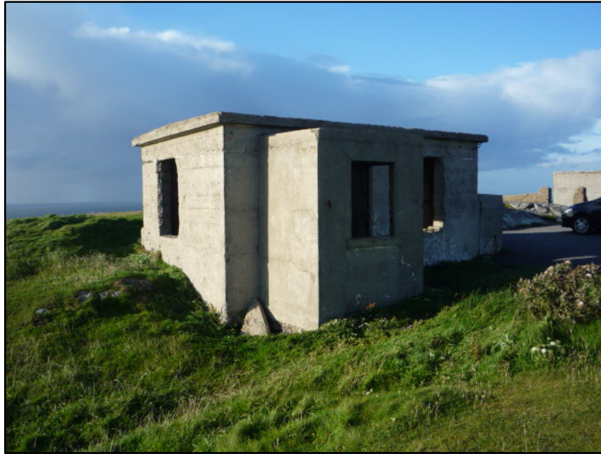
Figure D.121. The 'semaphore watch house' located to the west of the signal tower at Malin Head Signal Station, looking north-west.
