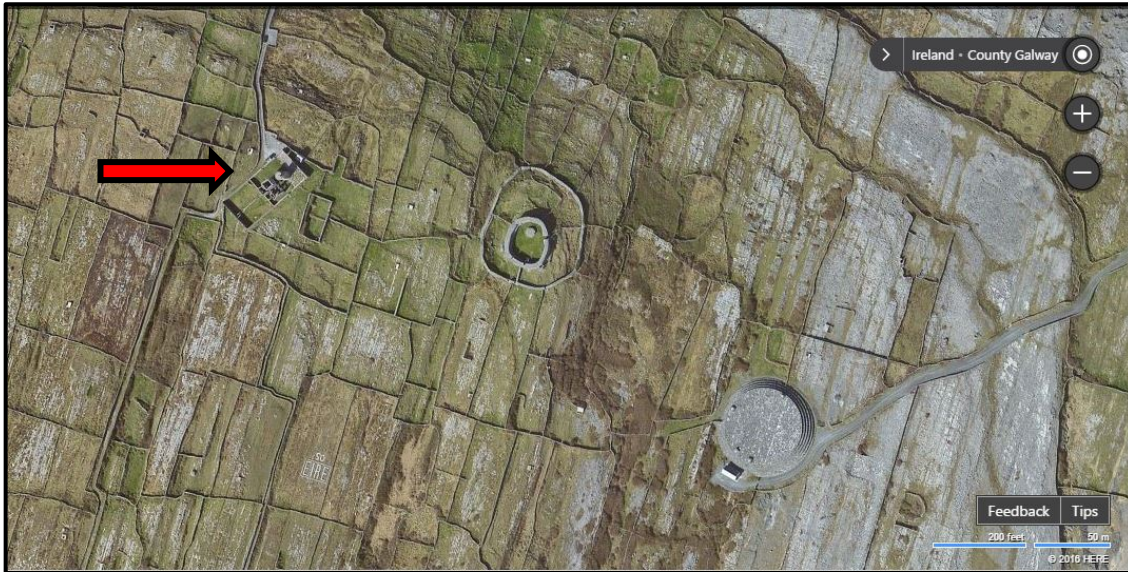
Figure A.23. Aerial photograph showing Inishmore signal station in the top left of the image (Bing Maps).
