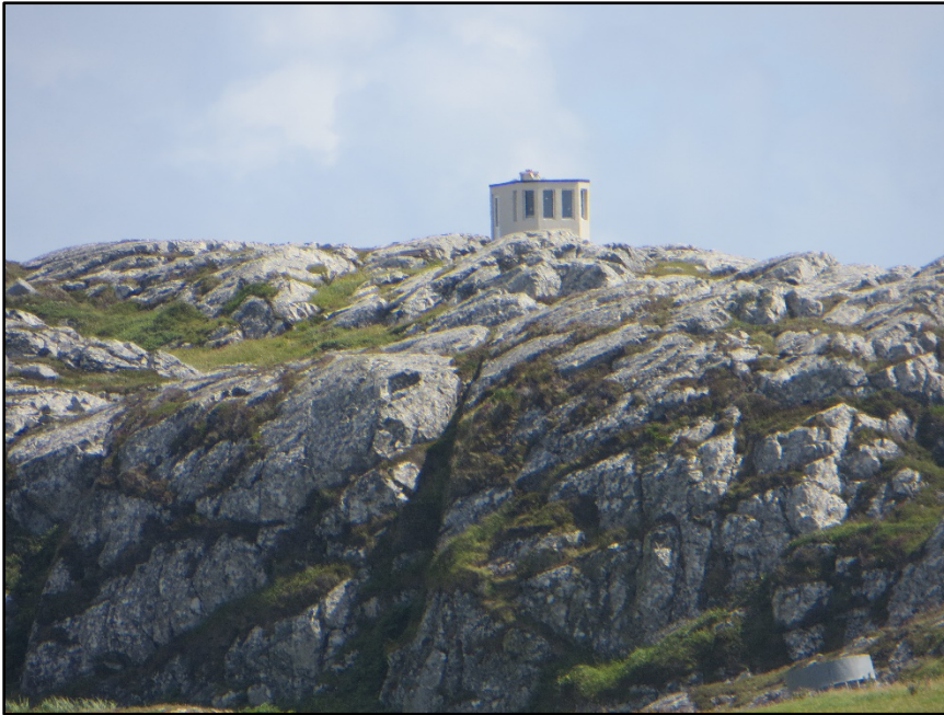
Figure A.63. View of the restored Look Out Post (L.O.P 51) on Lettermullan Island.
