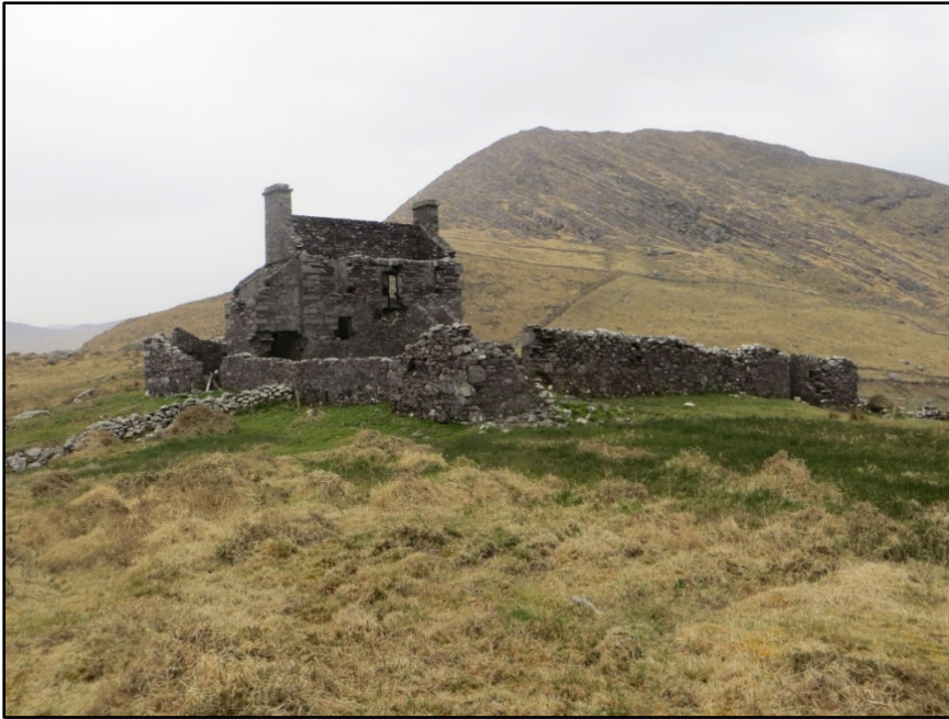
Figure G.2. Hog's Head Enclosed Barrack, looking west, with the western bastion in the foreground.
