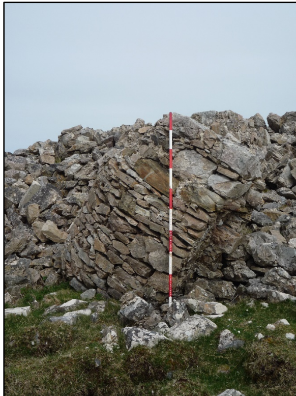
Figure B.70. Detail of the fallen bartizan in the rubble spread surrounding the collapsed signal tower.
