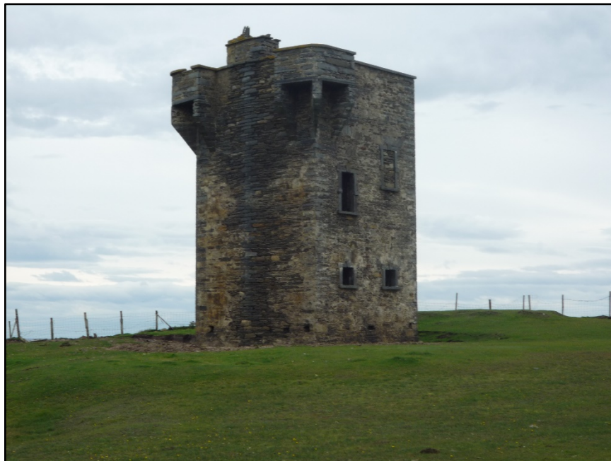
Figure D.24. The north-east corner of the signal tower at Malin Beg Signal Station.
