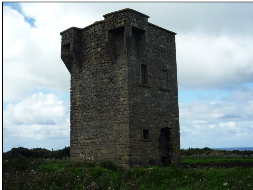
Figure C.38. The south-east corner of the signal tower at Carrowmably Signal Station.
