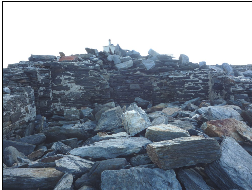
Figure D.51. The internal face of the south-east wall of the collapsed signal tower at Dawros Head Signal Station, with the lower portions of the ground floor central fireplace and flanking alcoves visible.
