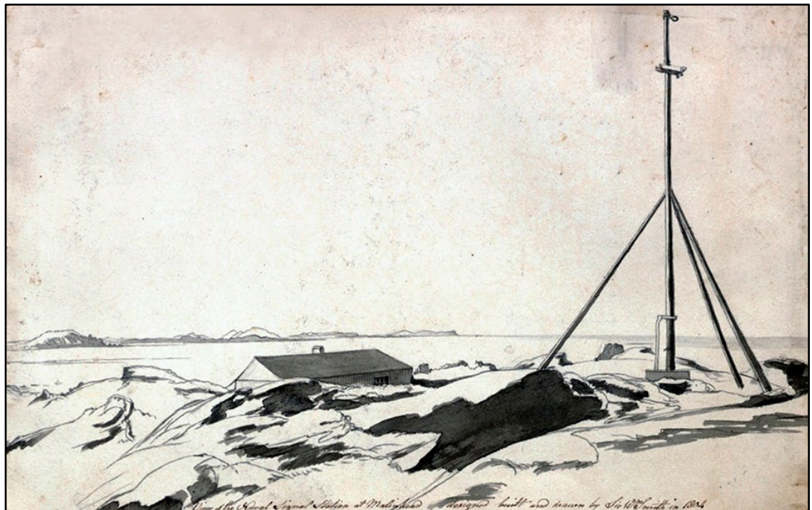
Figure D.130. View of the Naval Signal Station at Malin Head seen looking the way of Malin Well erected by Sir Wm Smith in 1804 & also drawn by him. (TCD MS 942/1: 16).
