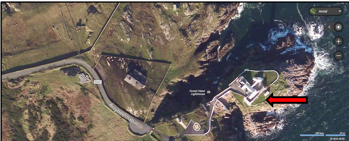
Figure D.103. Aerial photograph showing the Fanad Head lighthouse which overlay the position of Fanad Head Signal Station towards the right of the image. Fanad Head coast guard station is shown in the centre of the image (Bing Maps).
