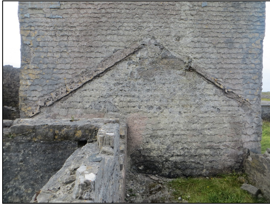
Figure A.36. The impression of the roof of the single storey addition on the north-east wall.
