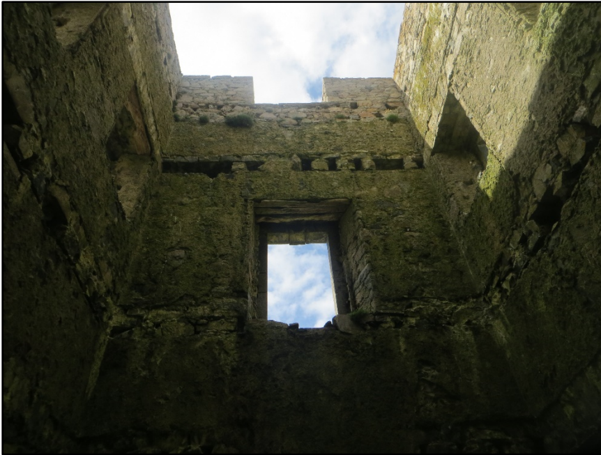
Figure A.59. The upper portion of the internal face of the south-west wall, showing the joist holes of the first floor, the doorway with traces of its timber framing, the joist holes of the attic level, the instep of the parapet and the entrance to the machicolation.
