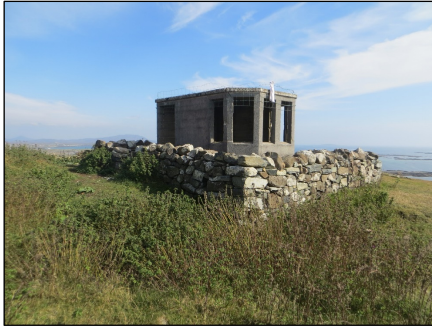
Figure A.83. The well-preserved Look Out Post close to the site of Bunowen Hill Signal Station.
