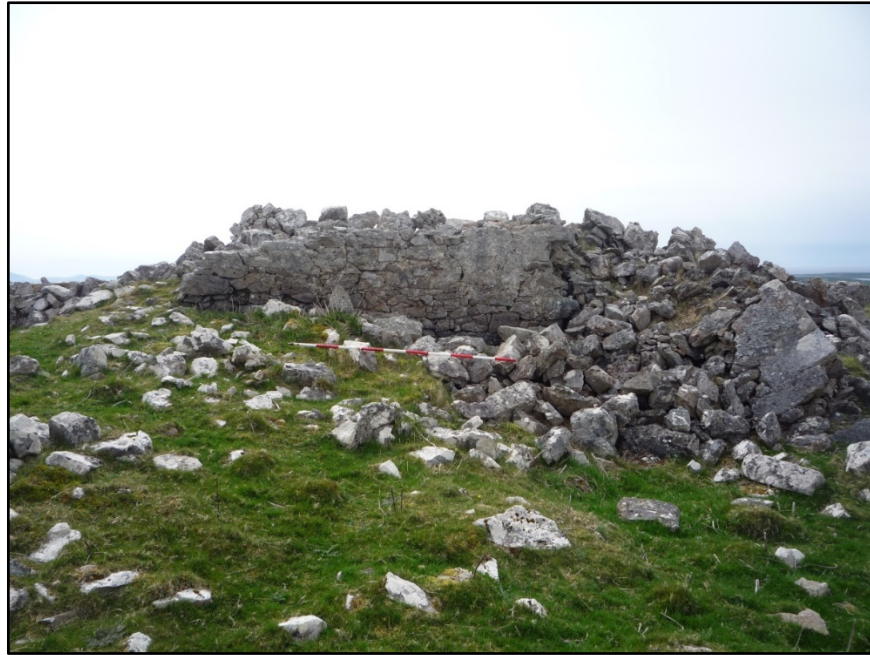
Figure B.68. The north-east side of the signal tower at Tower Hill Signal Station.
