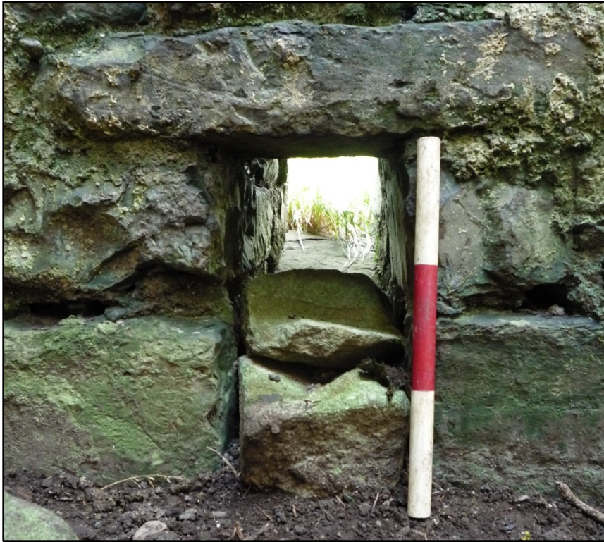
Figure C.47. Detail of the chute passing through the south wall into the semi-basement level.
