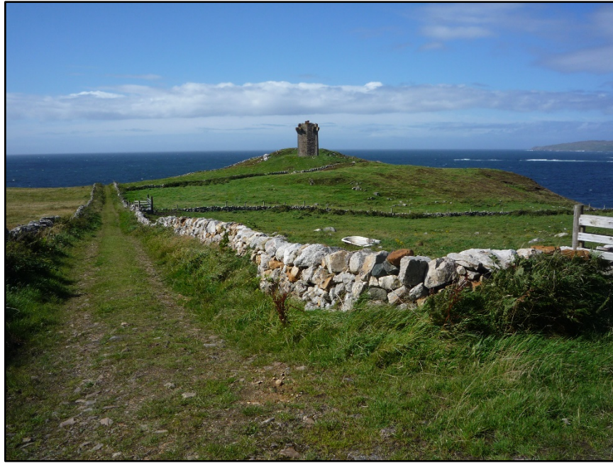
Figure D.57. View of Crohy Head Signal Station, looking west.
