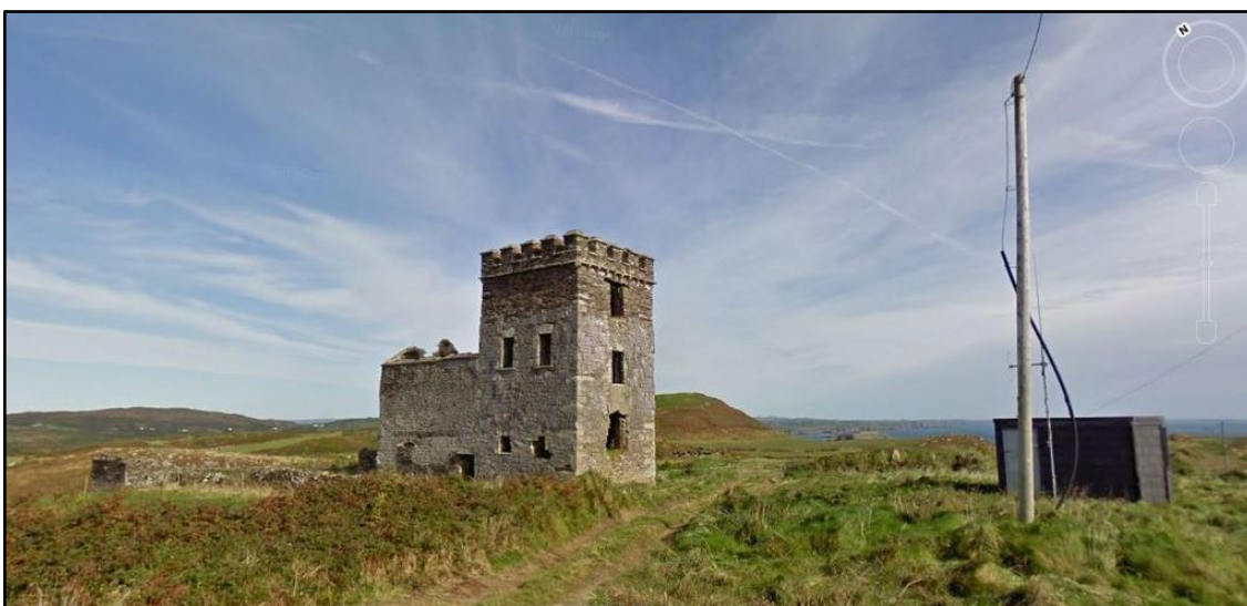
Figure F.14. Toe Head Signal Station, County Cork, looking north-east. (Photo courtesy of Google Earth).
