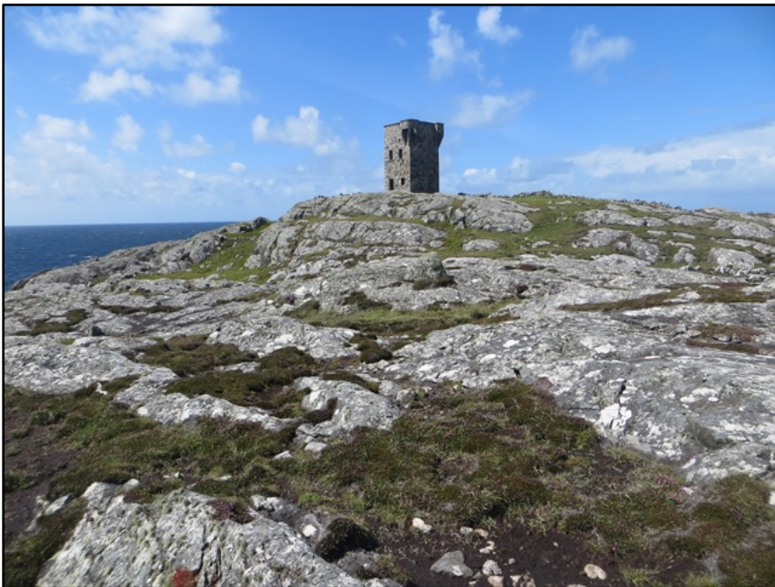
Figure A.52. A view of the signal tower at Golam Head Signal Station, set on the low hill towards the western end of Golam.
