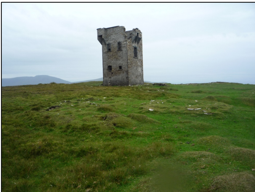
Figure D.40. The north corner of the signal tower of Glen Head Signal Station.
