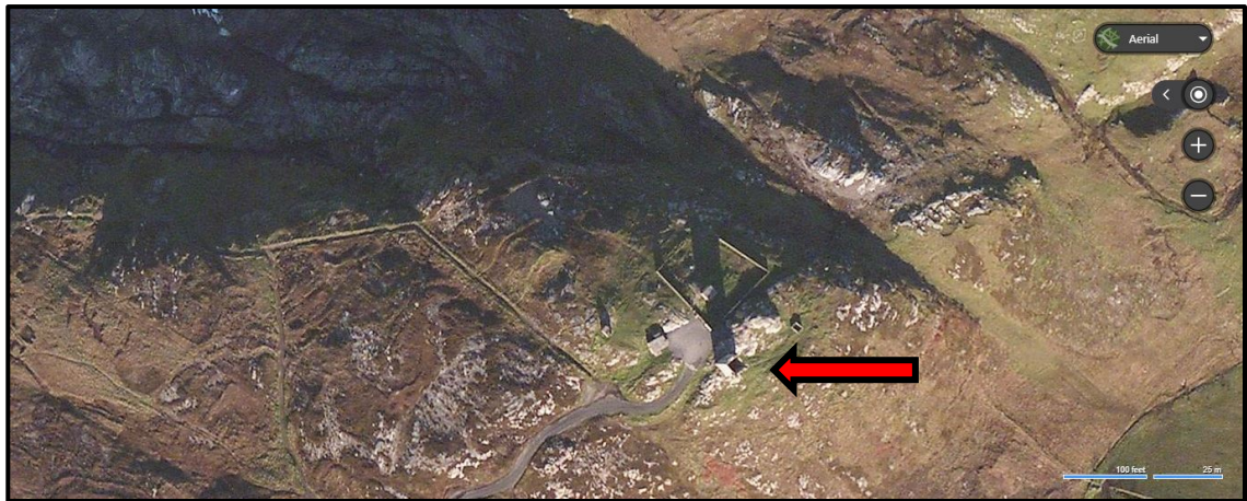
Figure D.116. Aerial photograph showing the complex of different communications building at Malin Head. The signal tower is shown below the centre of the image (Bing Maps).
