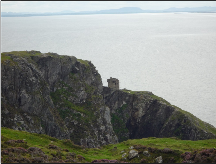
Figure D.11. View of Carrigan Head Signal Station, looking south-east towards the north-west corner of the signal tower.
