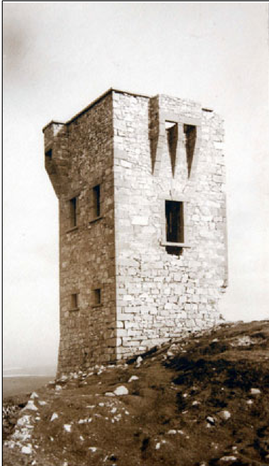
Figure A.88. Historic photograph of Cleggan Hill Signal Tower, looking south-east. The signal tower is clearly of the standard design and closely resembles the signal tower at Lettermullan Signal Station (A.52). Note the suggestion of a collapsed enclosure wall at the bottom left of the image, which would be north-west of the signal tower (The Signal Towers of Ireland 2006).
