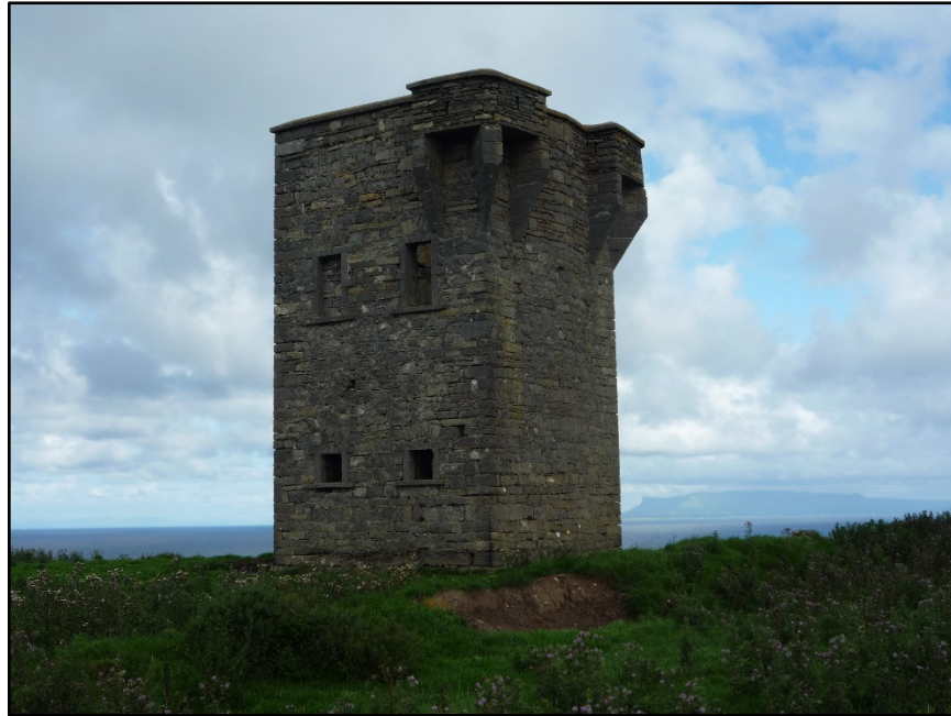
Figure C.37. The south-west corner of the signal tower at Carrowmably Signal Station.
