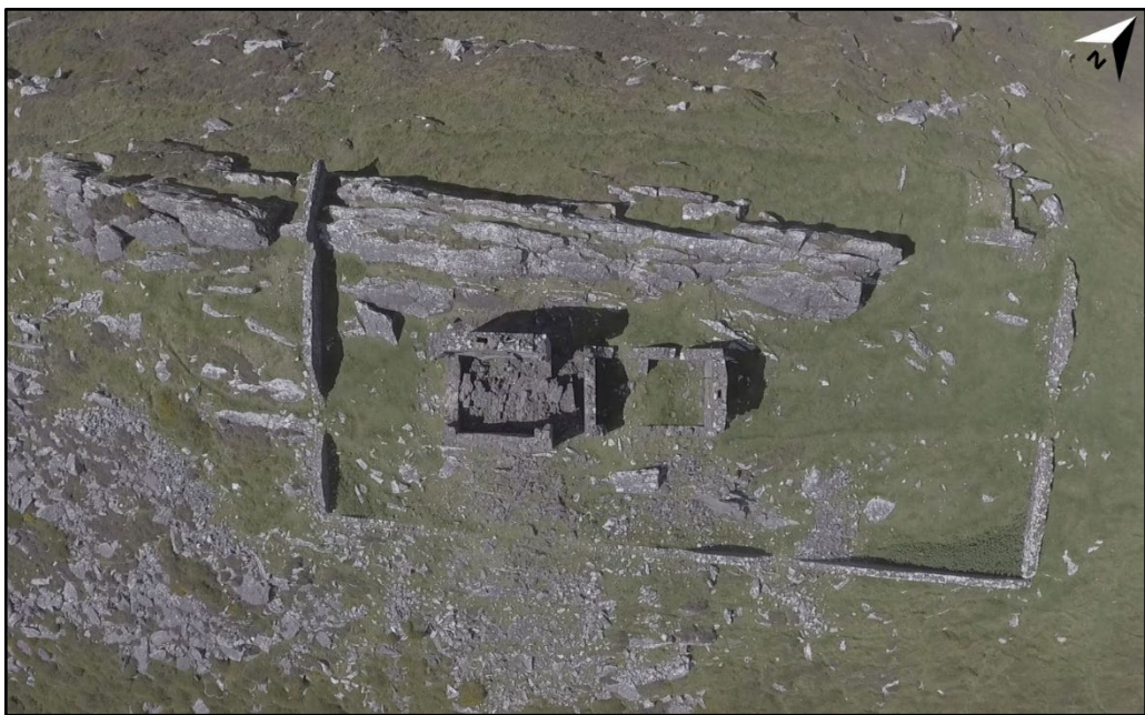
Figure F.36. Drone photograph of Ballydavid Head Signal Station showing the enclosure with traces of an entrance at the north-east and the small building at the north corner. The signal tower is towards the south-west end of the enclosure and the gabled building is located to the north-east of the tower. (Photograph courtesy of Dr James Bonsall).
