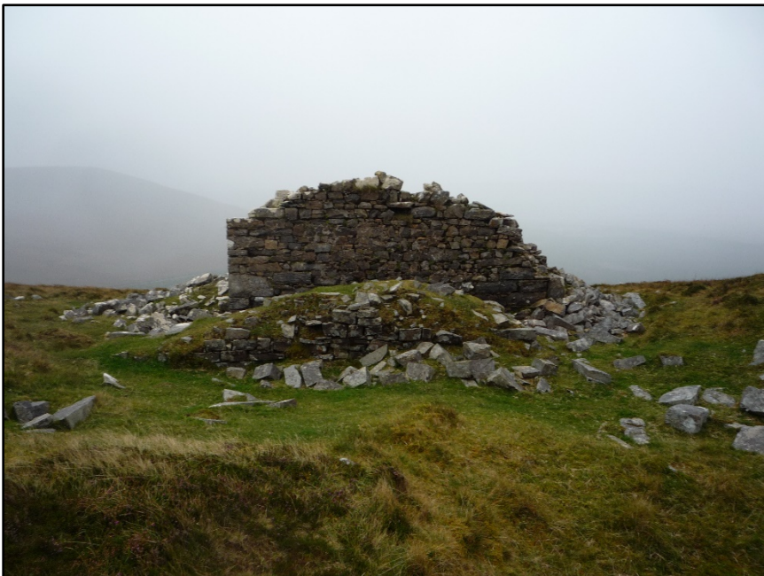
Figure B.83. The external face of the north wall of the collapsed signal tower at Glinsk Signal Station. The wide section of wall that may belong to a second building is visible in front of the tower.
