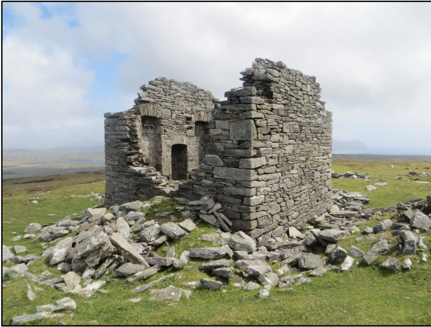
Figure B.36. View of north-west corner of the signal tower at Saddle Hill Signal Station.
