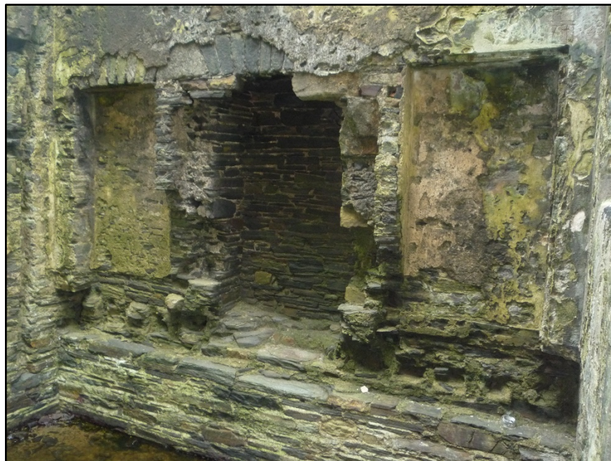
Figure D.28. The lower portion of the north-east internal wall face of the signal tower at Carrigan Head Signal Station. The upper part of the semi-basement level, the ground floor slot, the central fireplace and the flanking alcoves are visible.
