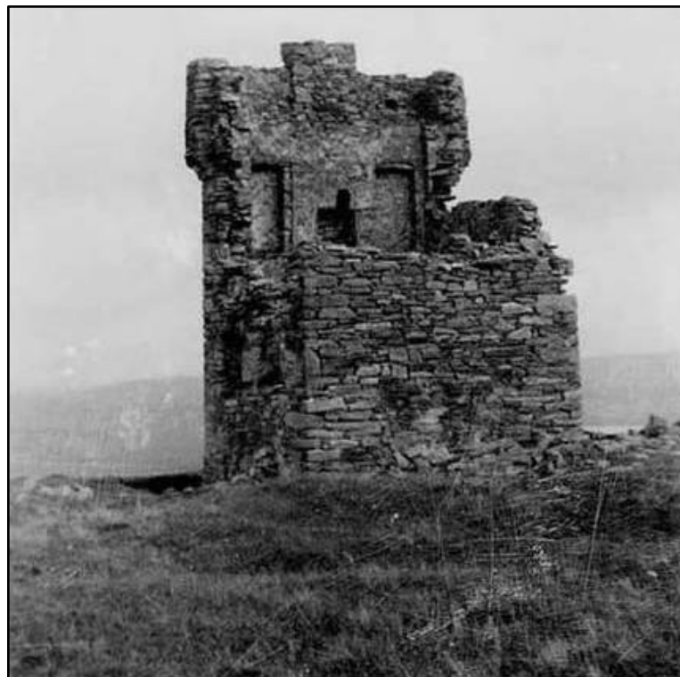
Figure B.35. A second undated photograph of Saddle Hill Signal Tower. The collapsed western walls allow the presence of first floor alcoves and fireplace on the eastern interior wall to be confirmed (From the personal collection of Michael O' Connor).
