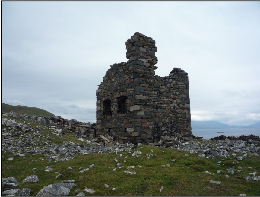
Figure B.19. View of the north-west corner of the signal tower at Clare Island Signal Station.
