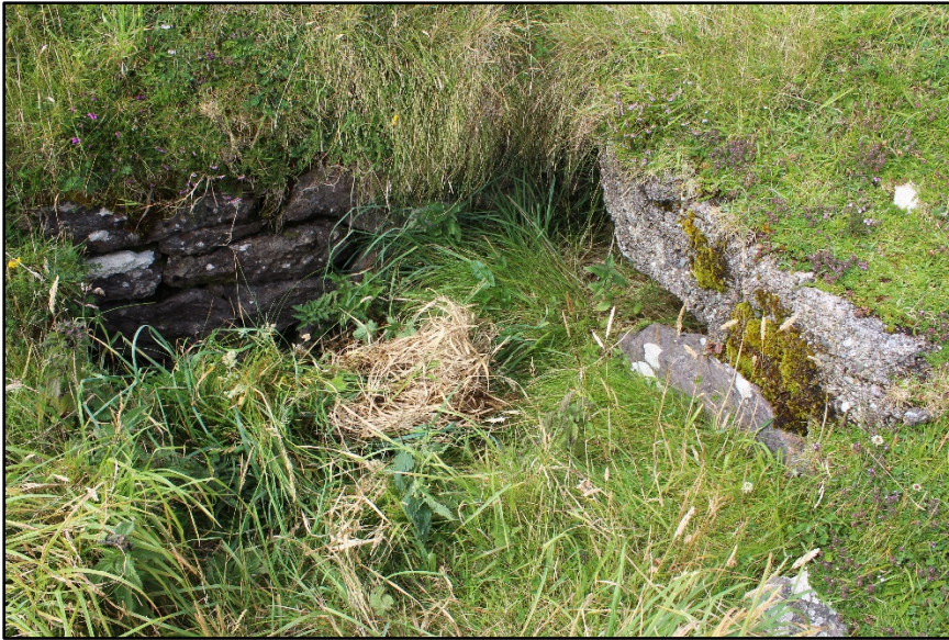
Figure F.34. detail of possible signal mast mount to the south-west of the two storey building at Sybil Head Signal Station, County Kerry, looking north-east. (Photograph courtesy of Dr James Bonsall).
