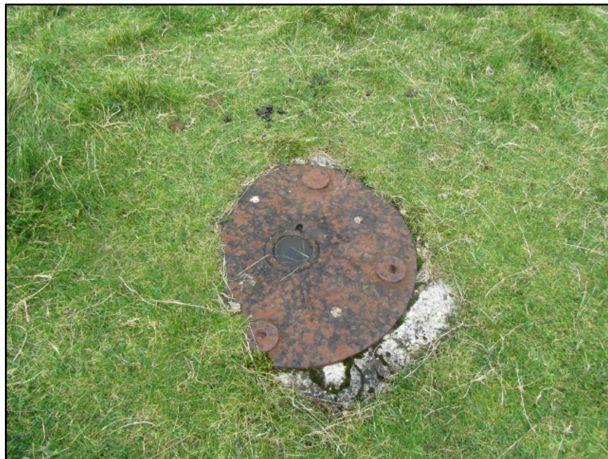
Figure F.33. Detail of metal mounting plate located to the north-west of the two storey building at Sybil Head Signal Station, County Kerry, looking north-east. (Photograph courtesy of Dr James Bonsall).
