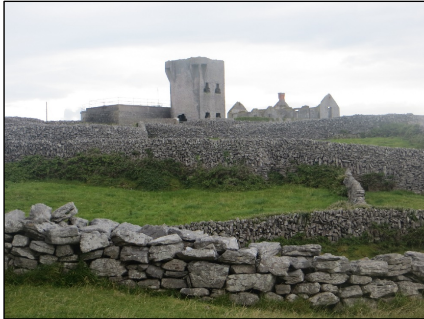
Figure A.5. View of Inisheer Signal Station from the north, showing the dense stone walled landscape in the foreground, the signal tower in the centre, the schoolhouse to the right of the signal tower and the rectangular water tank to the left of the signal tower.
