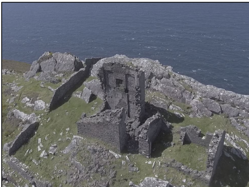
Figure F.38. Drone photograph of Ballydavid Signal Station, showing details of the signal tower and the adjacent gabled building, looking west. (Photograph courtesy of Dr James Bonsall).
