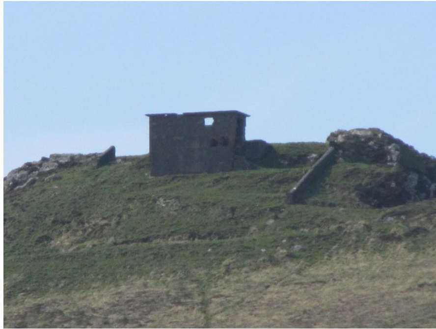
Figure F.25. Sybil Head Signal Station, County Kerry, looking north-west. The unusual two storey building and the enclosure wall can be seen. (Photograph courtesy of Isabelle Bennett).
