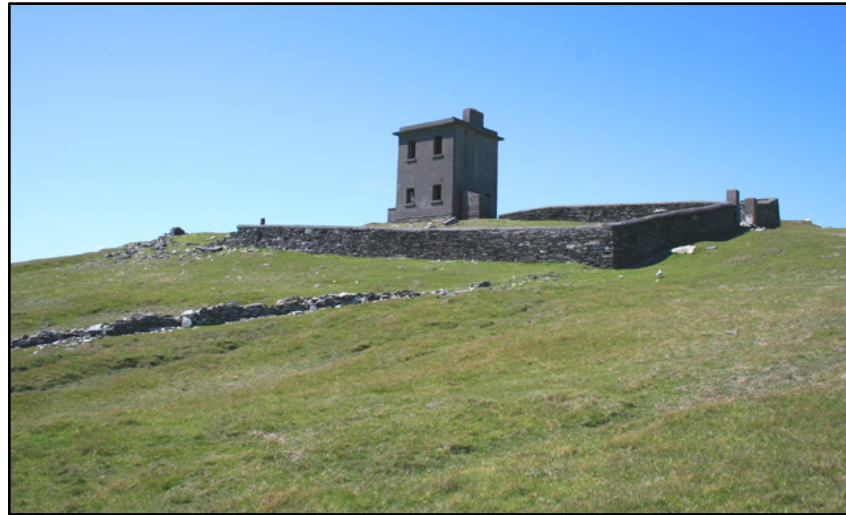
Figure F.22. Bray Head Signal Station, Valencia Island, County Kerry. (Photograph by Espresso Addict used under Creative Commons License 2.0).
