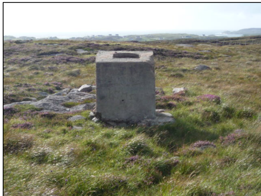
Figure D.73. Detail of the concrete structure adjacent to the signal tower at Mullaghderg Hill Signal Station, looking west.
