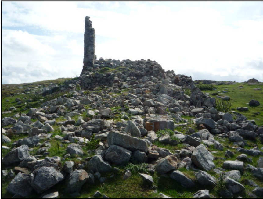
Figure D.99. The north side of the collapsed signal tower at Melmore Head Signal Station, looking south, with the extensive rubble spread in the foreground.
