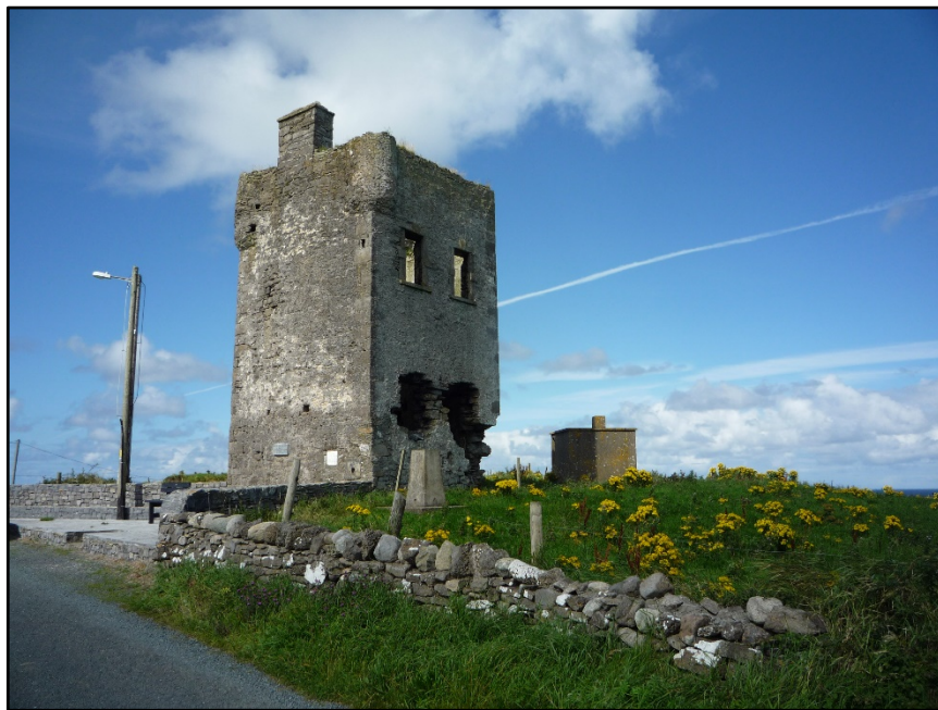
Figure C.19. View of the south-east corner of the signal tower at Rathlee Signal Station, with the trigonometry pillar in the foreground and L.O.P. 65 in the background, to the right of the signal tower.
