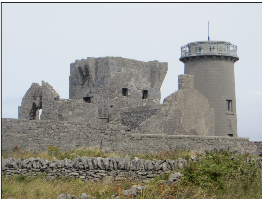
Figure A.27. Detail of the signal tower showing the south-west addition to the left, the south-east addition to the right and the cylindrical lighthouse in the background.
