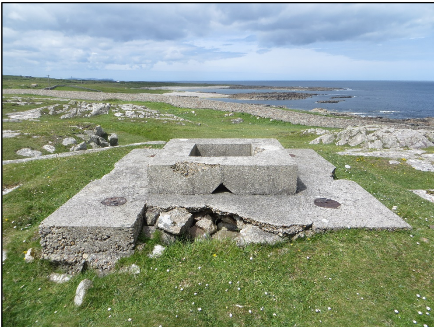
Figure D.108. One of several metal and concrete equipment mounts located in the vicinity of the early 20th Century watch house associated with Fanad Head Coast Guard Station.
