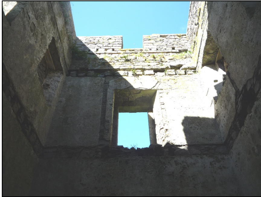
Figure C.41. The upper portion of the internal wall face of the north wall of the signal tower at Carrowmably Signal Station. The position of the first floor, the first floor door, the slot west of the door, the attic level slot, the instep at the parapet level, the parapet joists, and the entrance to the machicolation can all be seen.
