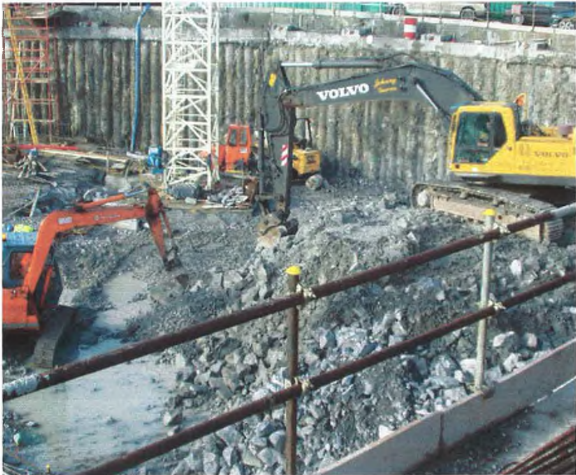
Photo 5.9 Rock and Subsoil Excavation.
