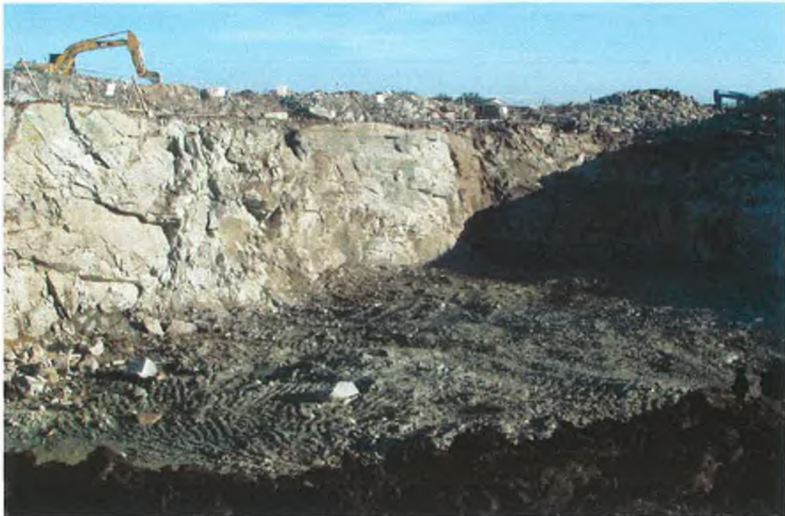
Photo 5.4 Natural Rock Excavation.
