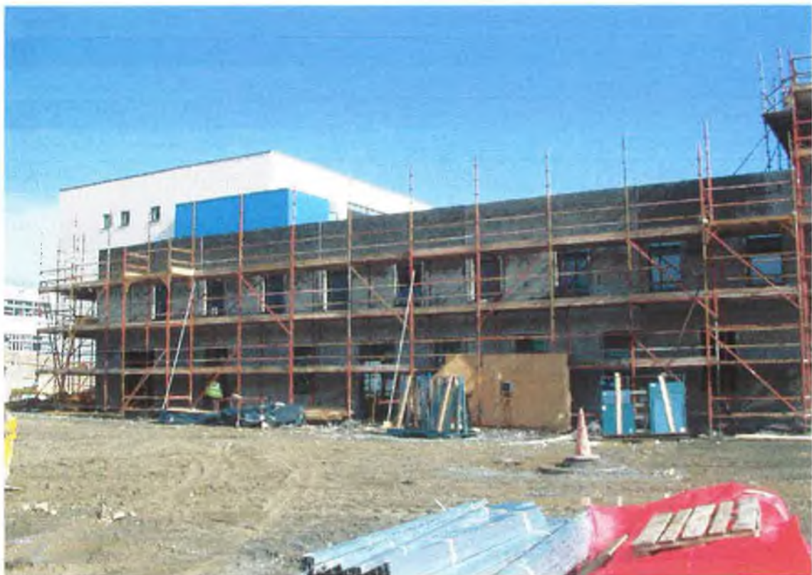
Photo 5.10 Construction in Progress.
