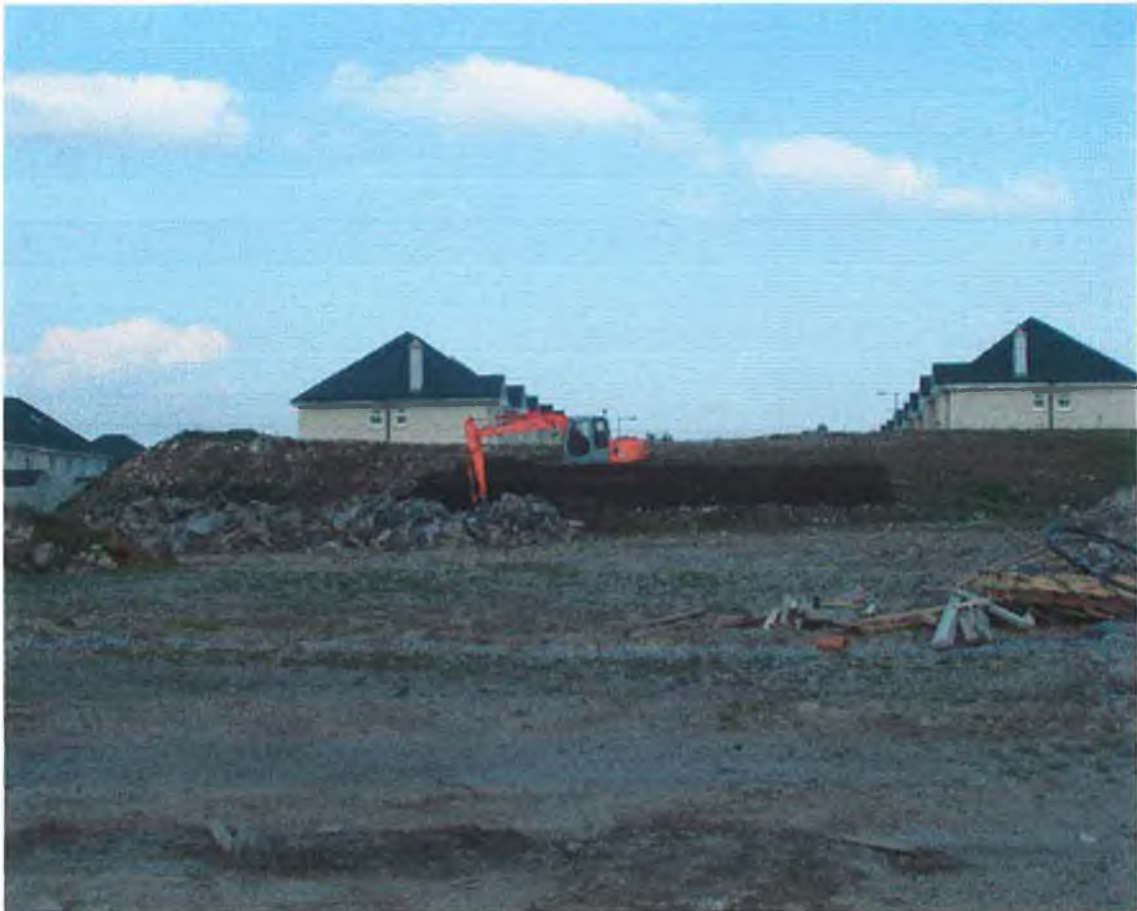
Photo 5.1 Topsoil Stockpile (15000m 3 ).
