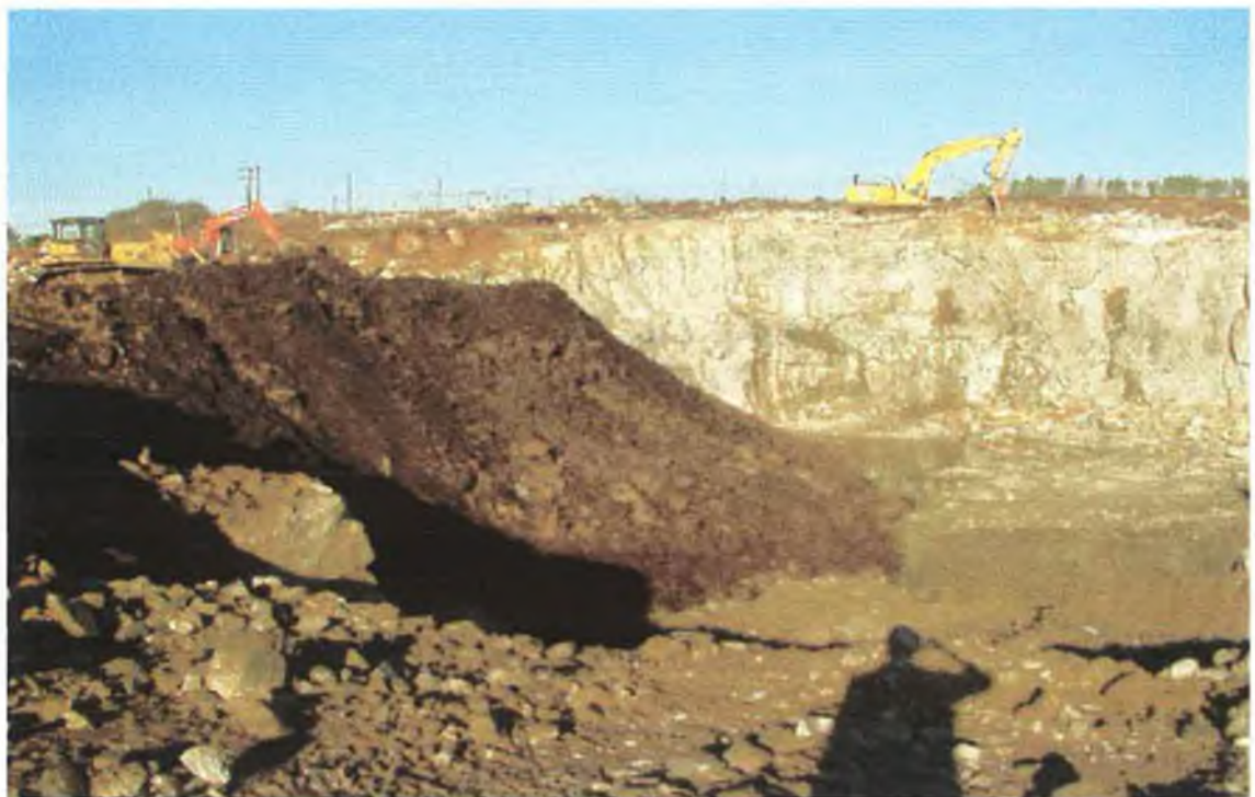
Photo 5.5 Backfilling with Waste Soils.
