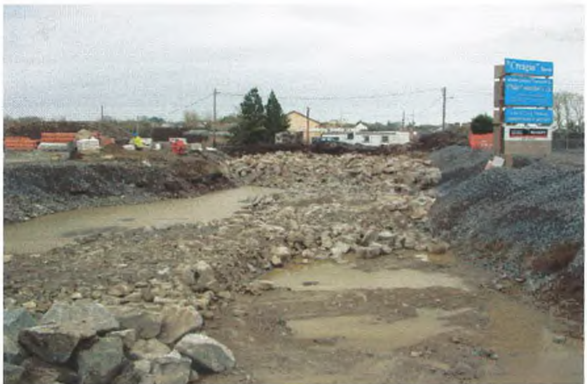
Photo 5.6 Reusing Crushed Rock.
