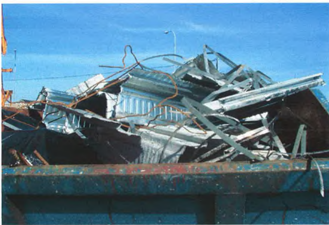
Photo 6.4 Metal Waste Disposal
