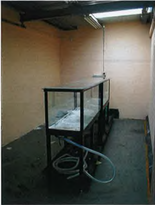
Figure D-5: Simulation tank after the build is completed
