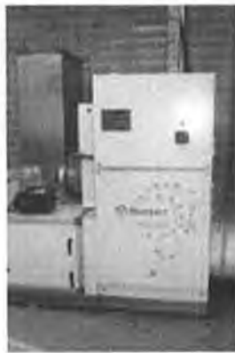
Figure F.4 Dehumidifier used to maintain dry air in the ambient room.
