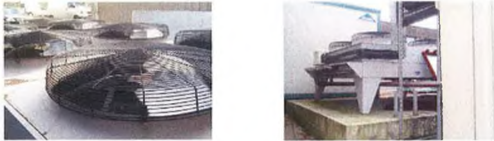
Figure F.2 Air Cooled Condenser Pack.
