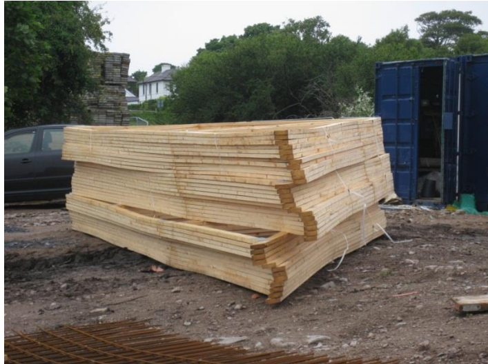
Picture 6.7 Timber roof trusses
