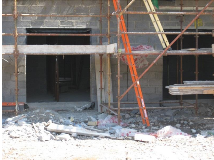
Picture 6.71 Cleaning out waste 1
