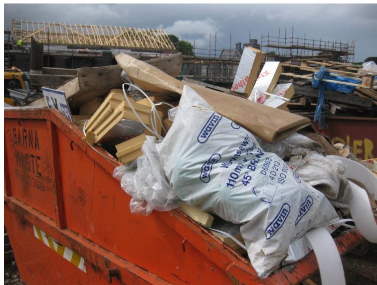
Picture 7.1 Mixed waste skip on site
