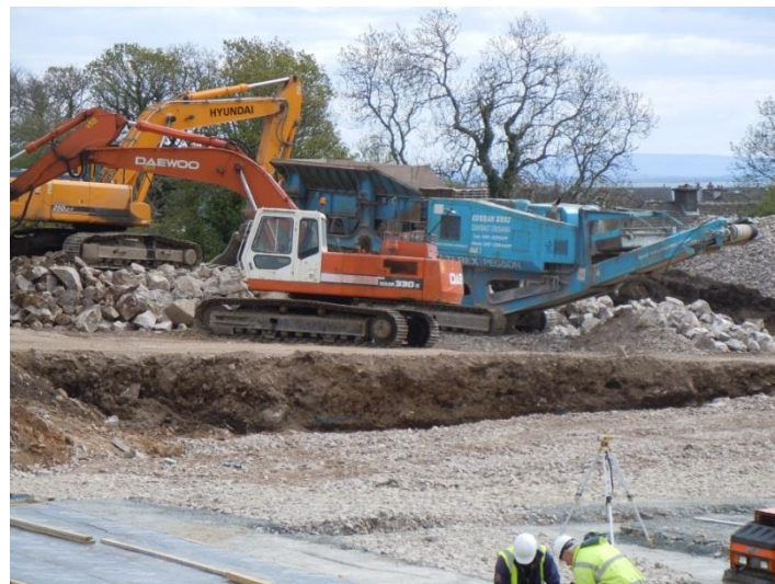
Picture 6.2 On-site crusher
