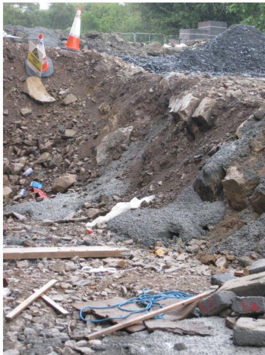
Picture 6.45 Concrete waste after delivery 3
