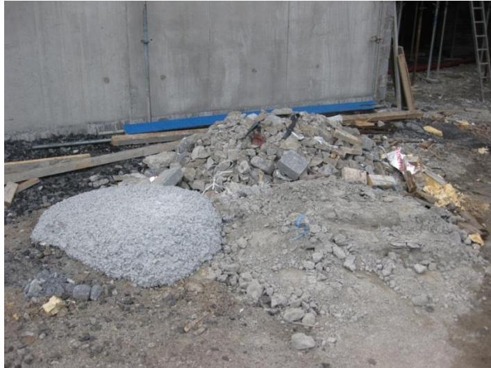
Picture 6.44 Concrete waste after delivery 2
