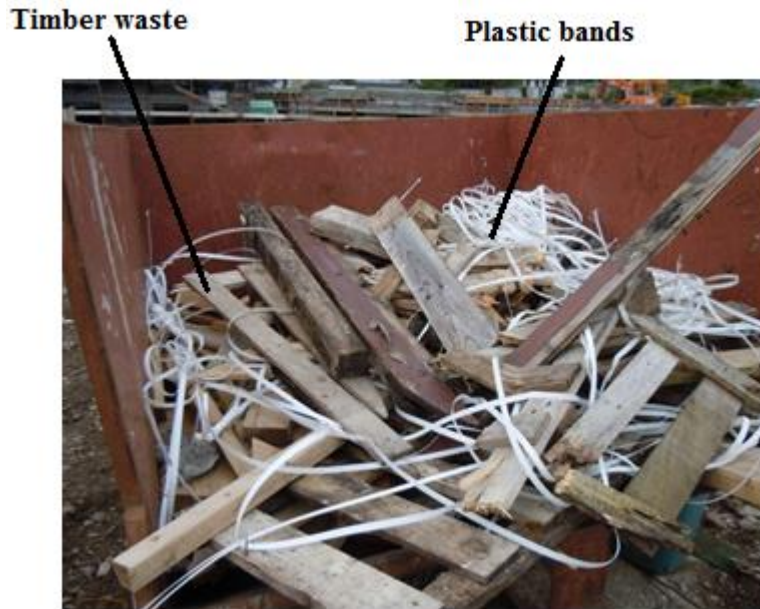
Picture 6.85 Mini skip with timber waste 22 nd of May
