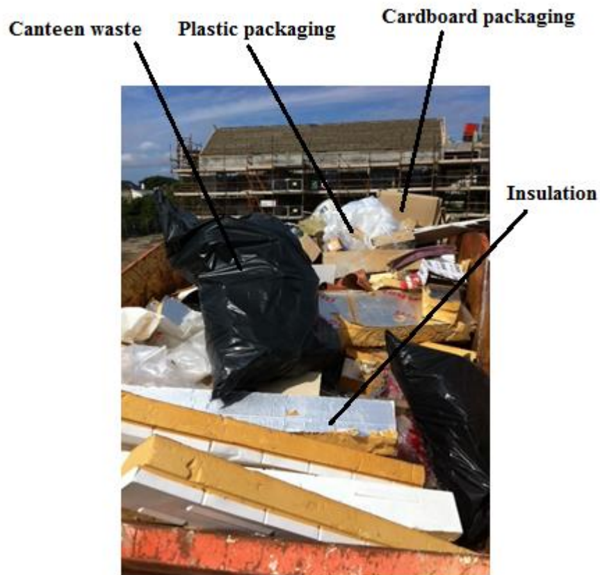
Picture 6.101 General waste skip 26 th of July
