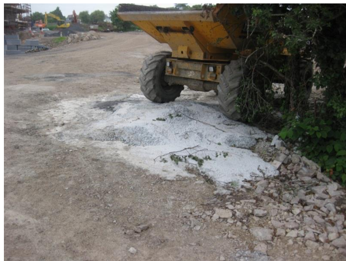
Picture 6.43 Concrete waste after delivery 1
