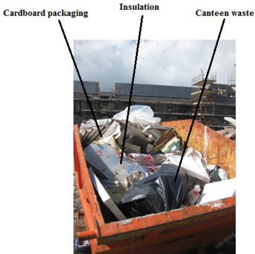
Picture 6.104 General waste skip 22 nd of August
