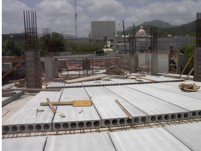
Picture 3.5 Hollowcore flooring
