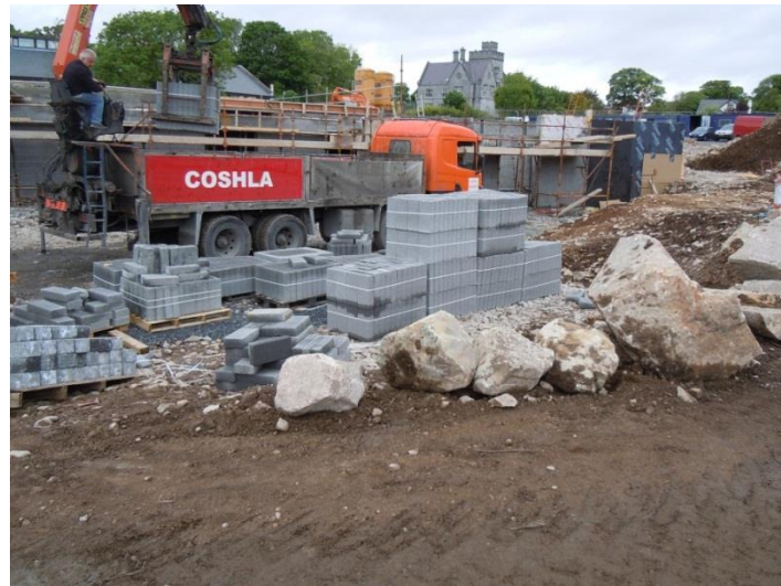
Picture 6.3 Delivery of blocks
