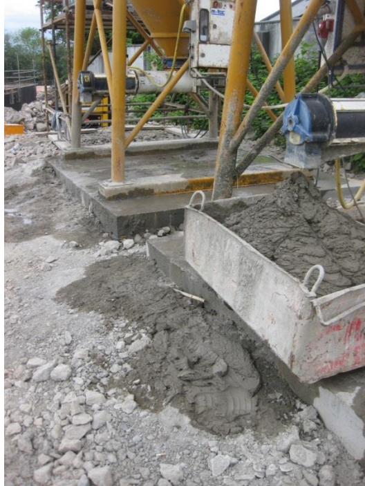
Picture 6.37 Overfilling mortar bins 1
