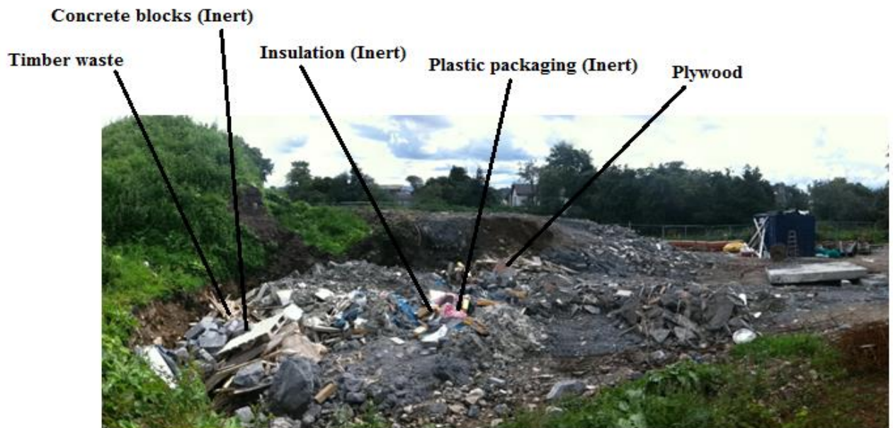
Picture 6.53 Fly tipping of waste on site
