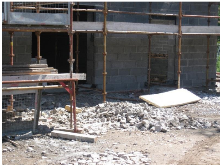
Picture 6.72 Cleaning out waste 2
