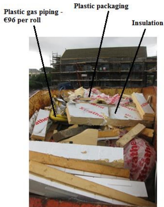
Picture 6.100 General waste skip 18 th of July
