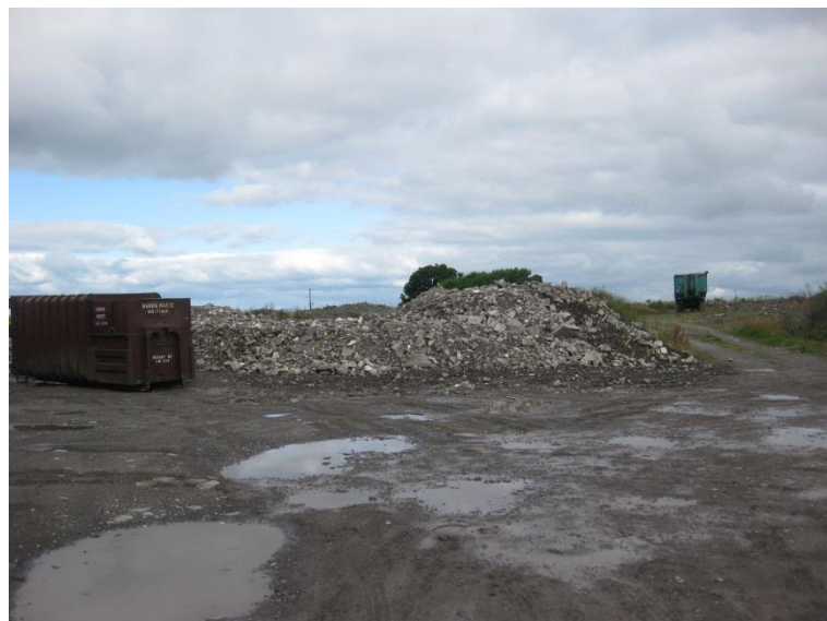
Picture 7.15 Concrete/ rubble used as fill
