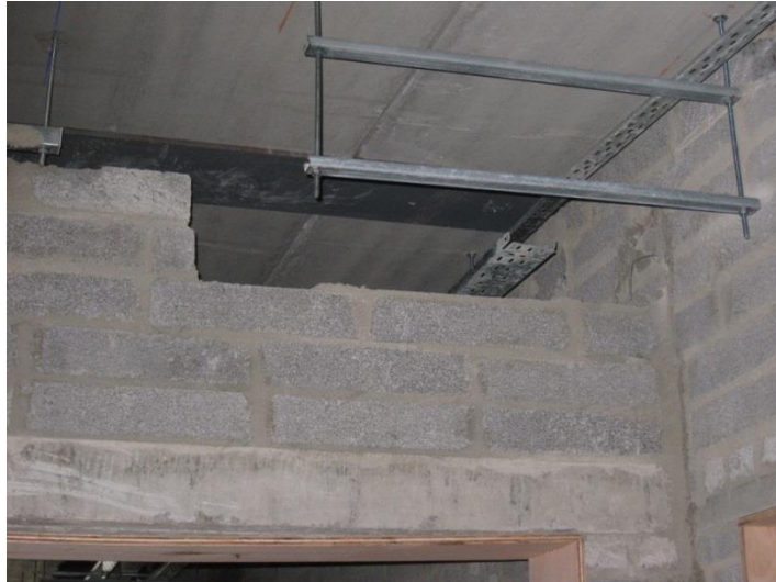
Picture 6.59 Breaking out for services
