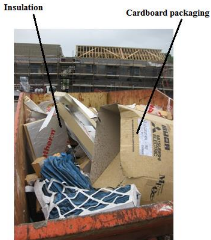
Picture 6.99 General waste skip 12 th of July
