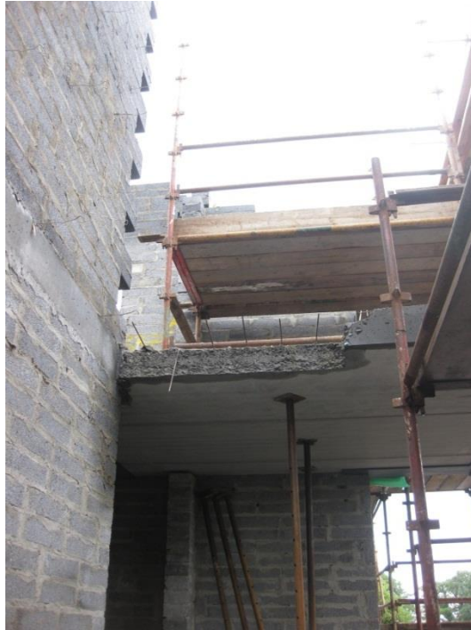
Picture 6.58 Breaking out to accommodate future work
