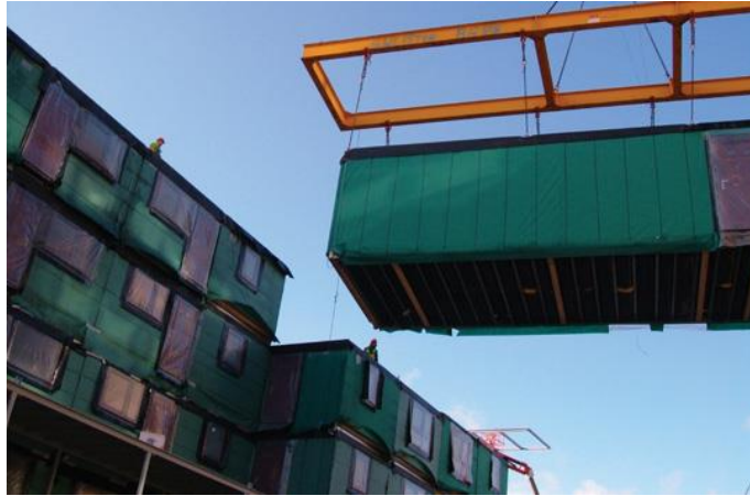
Picture 3.1 Volumetric modular construction
