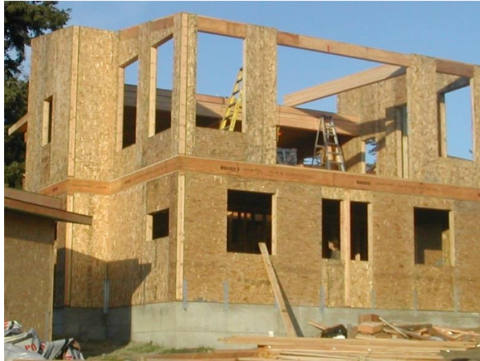
Picture 3.2 Timber frame construction using SIPs
