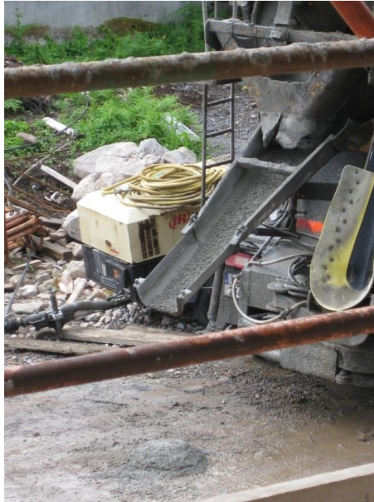
Picture 6.42 Wastage of concrete during delivery 2
