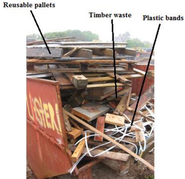
Picture 6.90 Mini skip with timber waste 5 th of June
