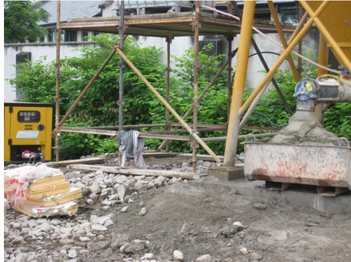
Picture 6.38 Overfilling mortar bins 2
