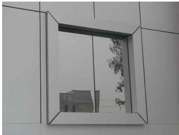
Picture 3.4 Composite panel cladding
