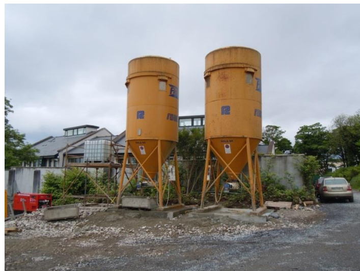
Picture 6.4 Mortar mixing silos
