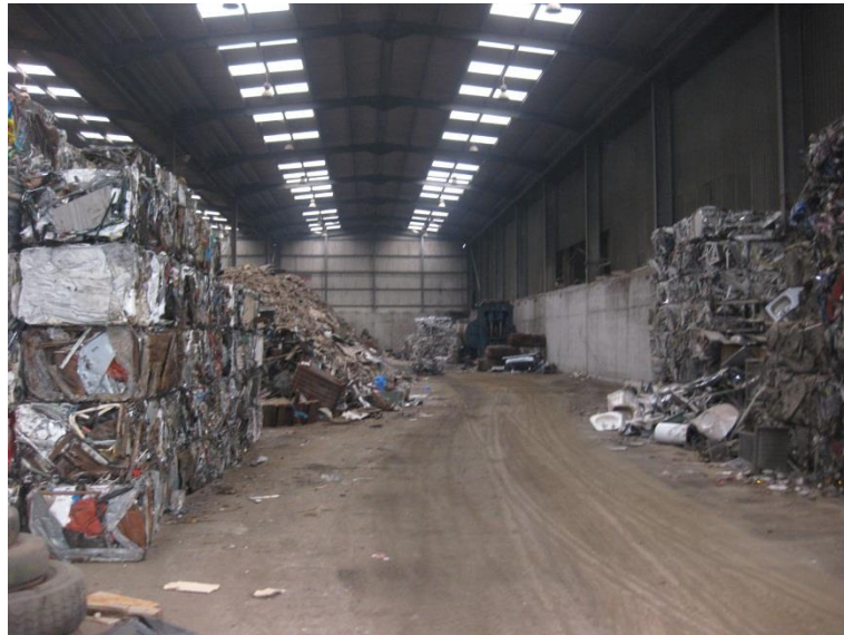
Picture 7.12 Metal waste holding bay
