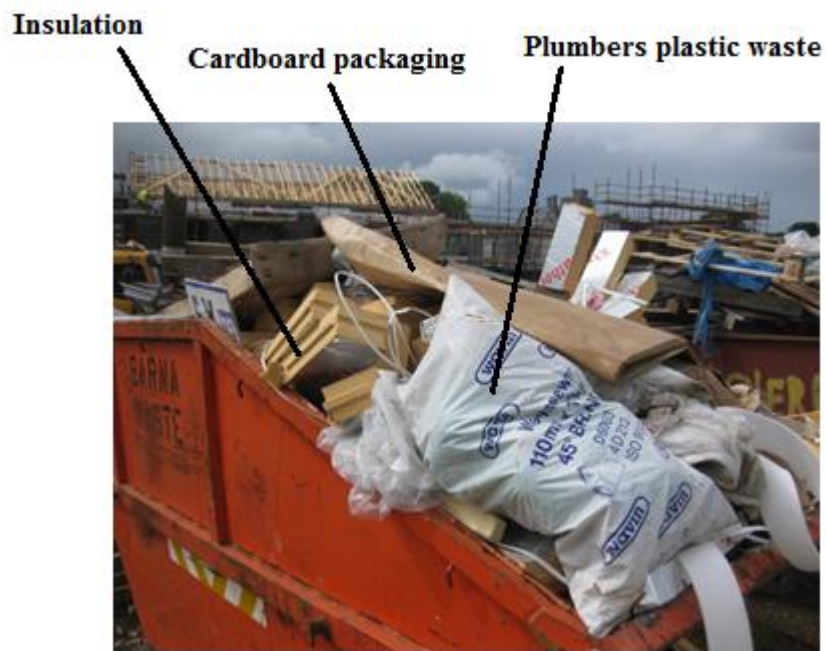
Picture 6.96 General waste skip 4 th of July
