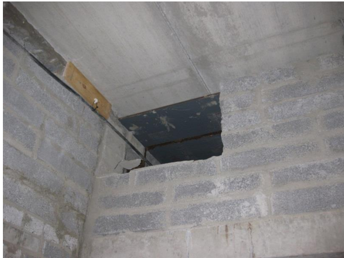
Picture 6.60 Breaking out for services
