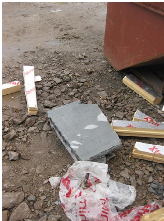
Picture 6.47 Hollowcore waste 2
