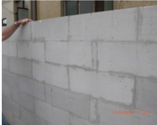
Picture 3.6 AAC blocks with thin joint mortar
