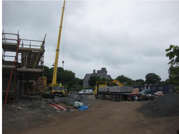
Picture 6.9 Hollowcore installation
