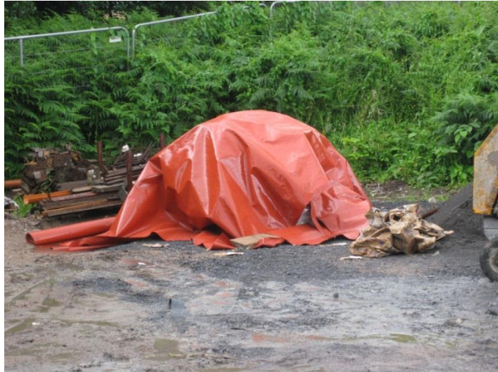
Picture 6.31 Incorrect use of materials 1
