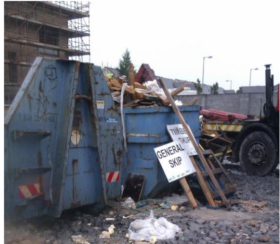
Photograph 5.24: Day 3. Skip signage
