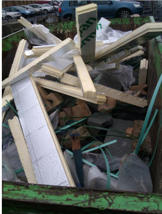
Photograph 5.27: Day 3. Mixed skip containing recyclable materials - approximately 4% non-compliance
