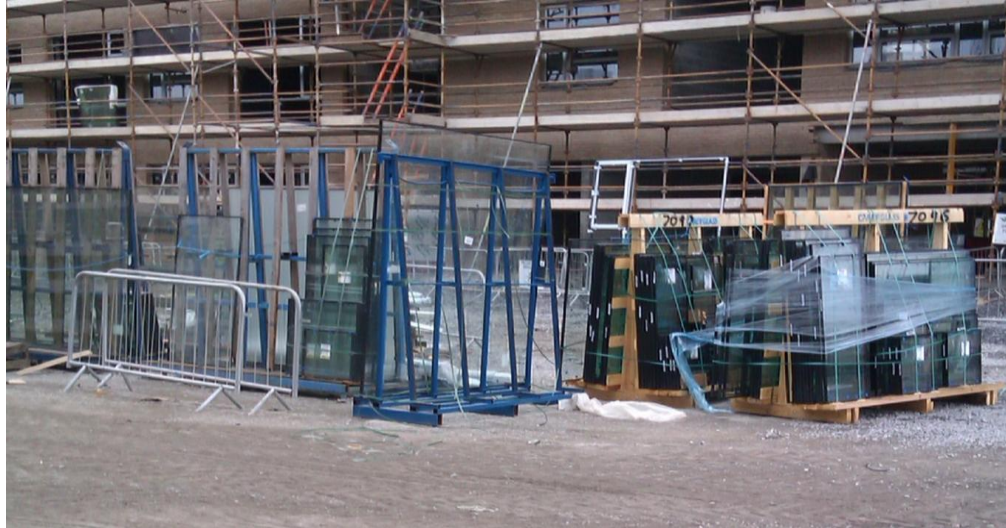
Photograph 5.21: Day 2. Glass and windows storage
