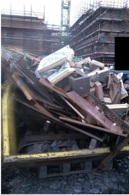
Photograph 5.25: Day 3. Timber skip A containing mixed waste – approximately 50% non-compliance. Site worker omitted for purposes of privacy.
