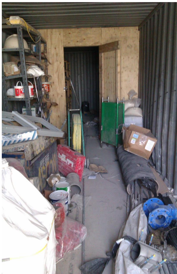
Photograph 5.12: Day 1. Indoor storage area with materials piled in the walkways
