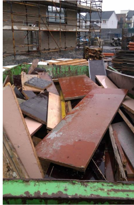
Photograph 5.26: Day 3. Timber skip B containing some metals – approximately 4% non-compliance
