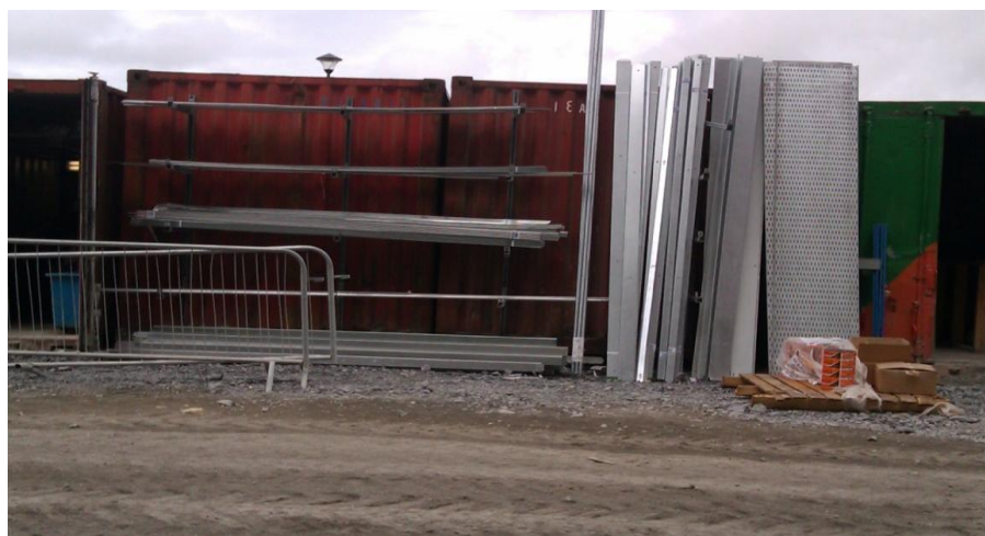
Photograph 5.22: Day 2. Aluminium roofing materials
