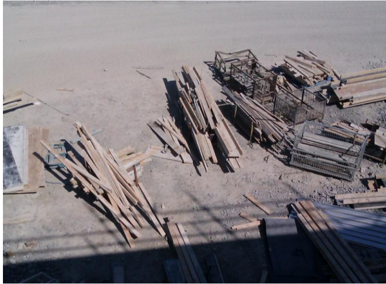
Photograph 5.7: Day 1. Storage of reusable timber A
