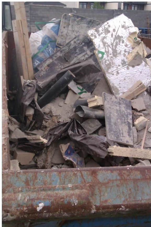
Photograph 5.39: Day 5. Skip intended for timber but containing mixed waste - 95% non-compliance
