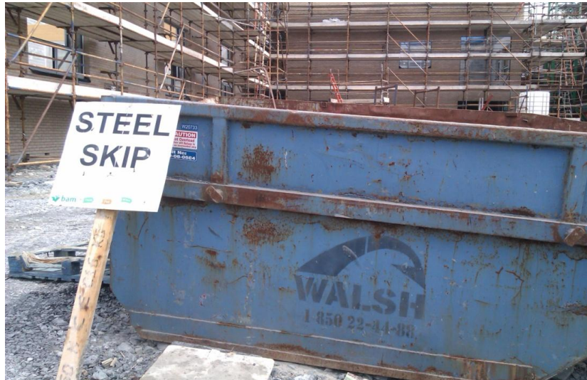
Photograph 5.17: Day 2. Metal skip signage
