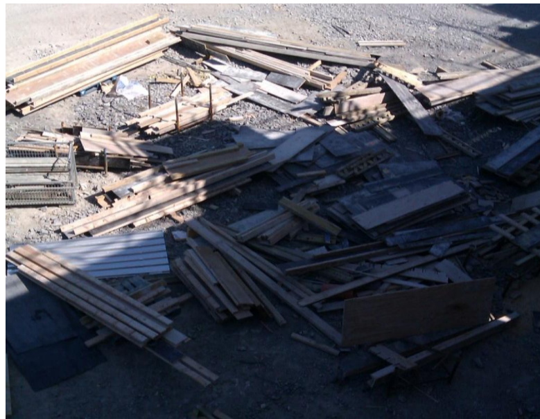
Photograph 5.8: Day 1. Storage of reusable timber B
