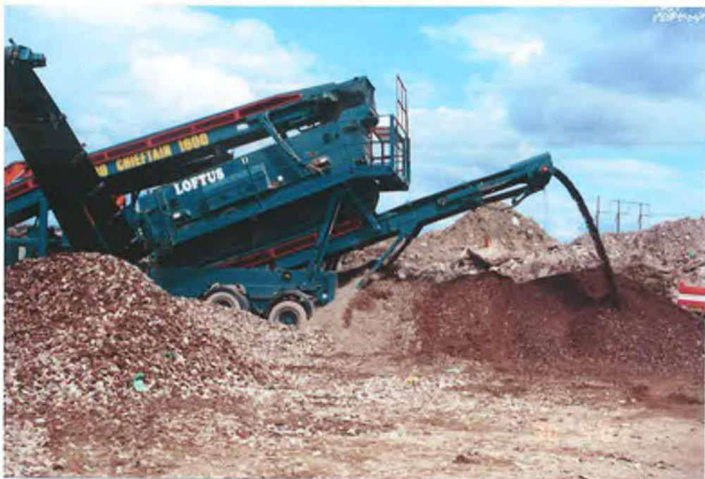
Photograph 6.3 Screening of material into three separate fractions on the DemCon 20/20 project
