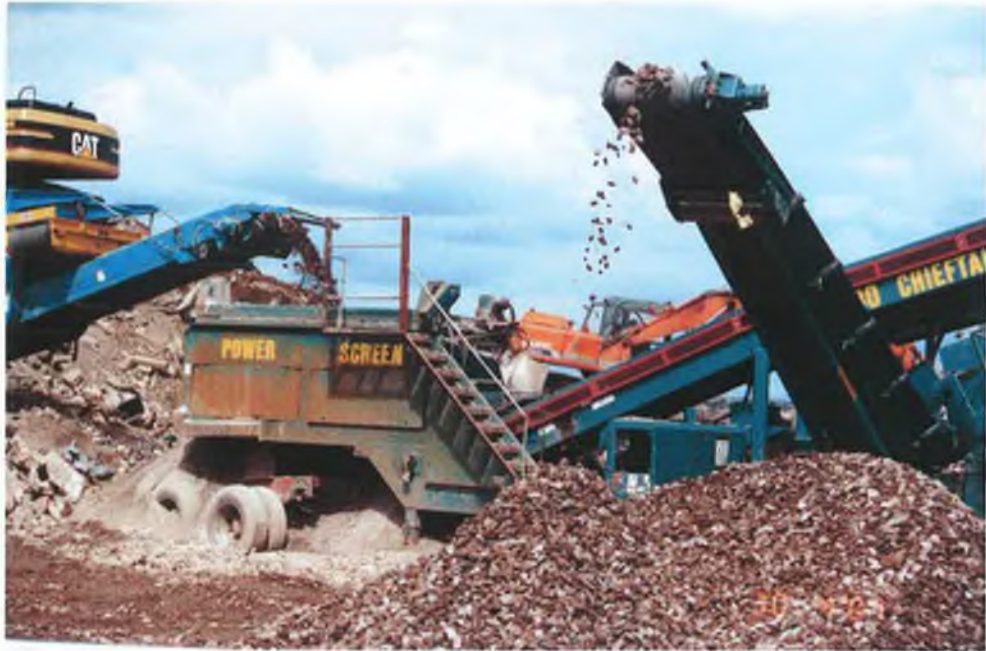
Photograph 6.2 Screening of construction and demolition waste materials on the DemCon 20/20 project
