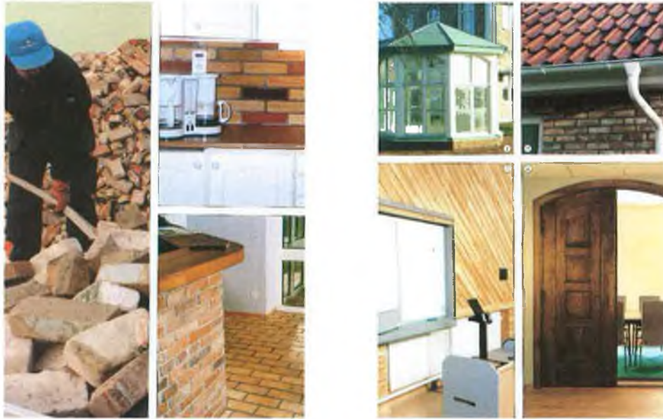
Photograph 6.21 Use of recycling building material at Sysav's head office
