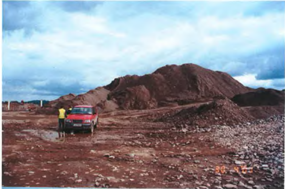
Photograph 6.4 Stockpiles of construction and demolition waste on the DemCon 20/20 project
