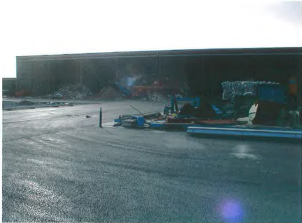
Photograph 8.2 View of waste transfer building on the Barna Waste site
