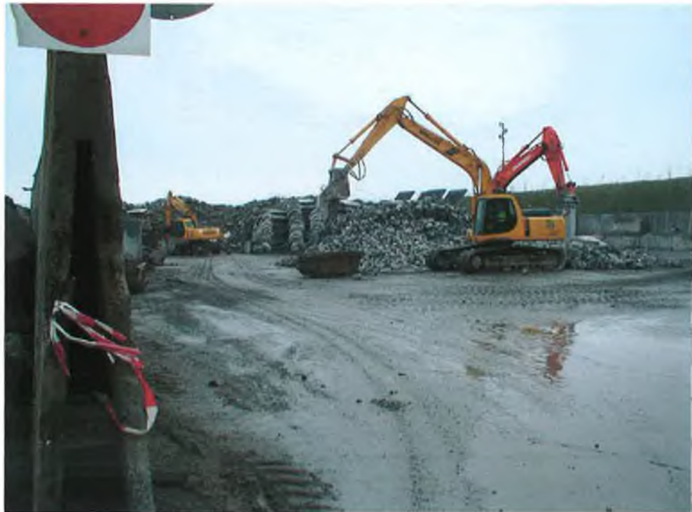
Photograph 6.10 Size reduction methods at the Copenhagen Recycling Centre
