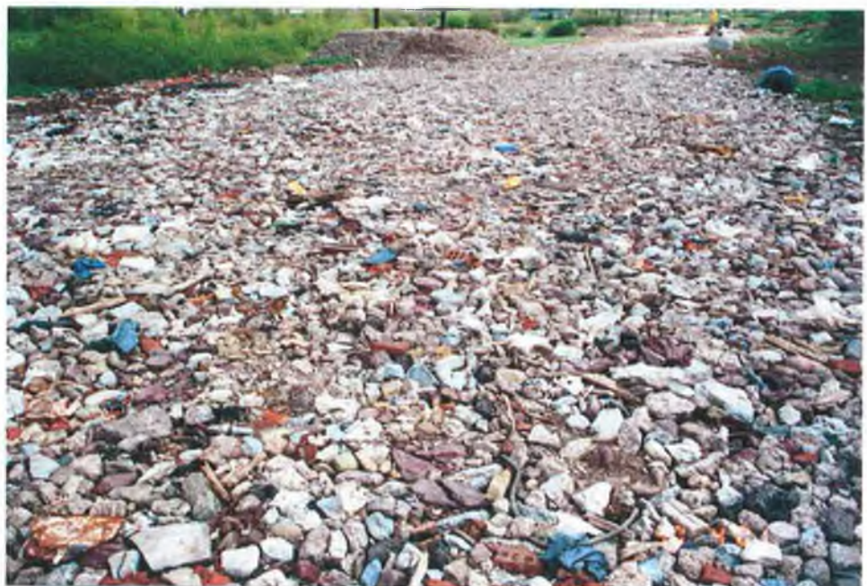
Photograph 6.5 Use of processed materials in the construction of landfill access roads
