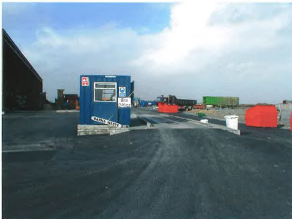
Photograph 8.4 View of weighbridge and associated office on the Barna Waste site
