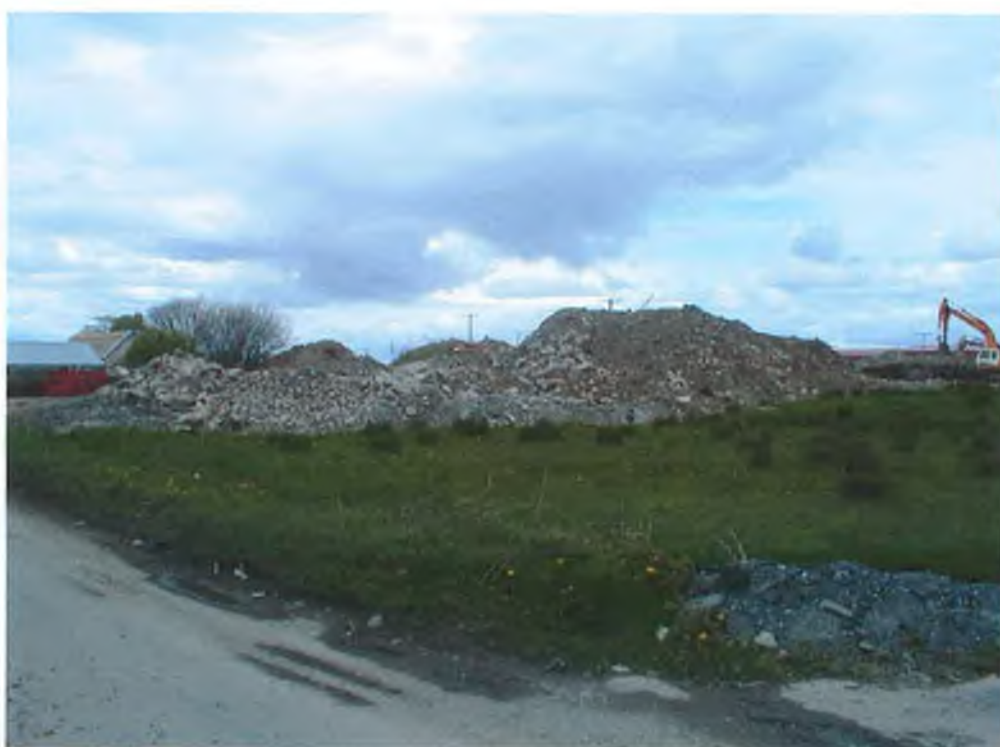
Photograph 8.8 Permitted adjacent site being filled with inert material
