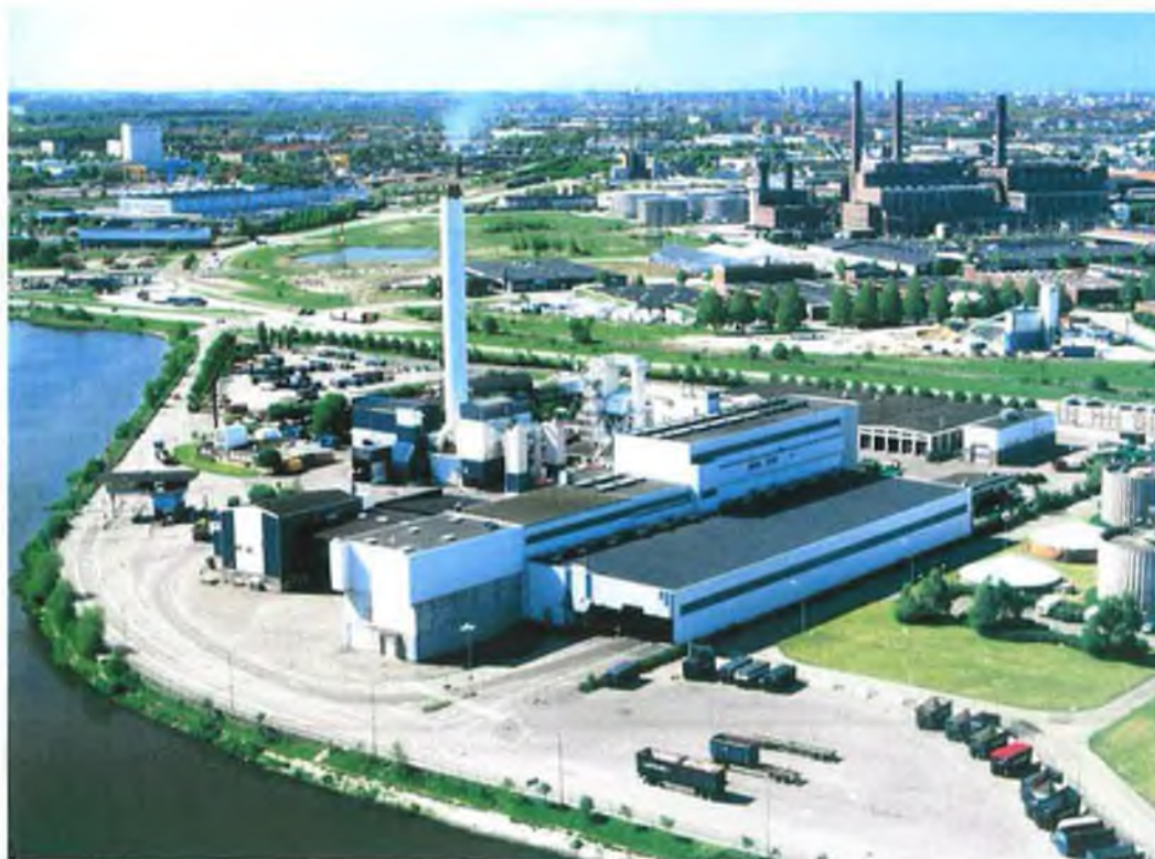
Photograph 6.14 Aerial view of the Sysav Facility in Malmo
