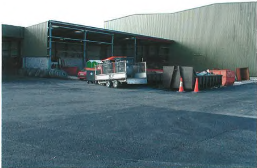
Photograph 8.3 View of maintenance building and yard on the Barna Waste site
