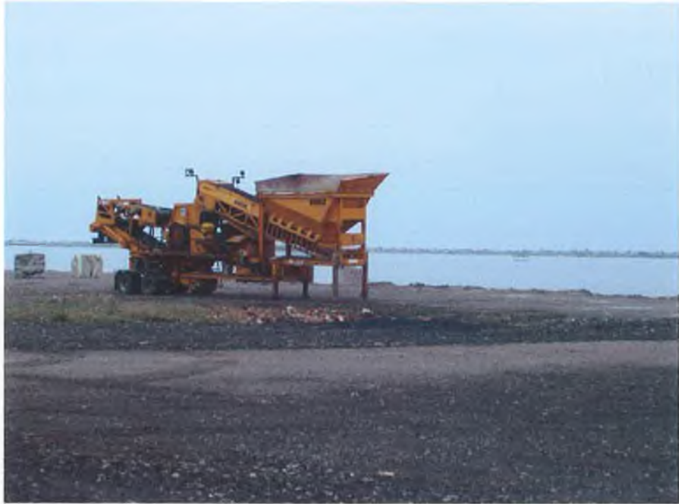
Photograph 5.3 Impact crusher on the Spillepeng Landfill site in Malmo, Sweden
