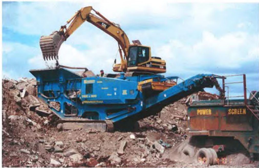
Photograph 5.2 'Jaw' crusher' in operation (DemCon 20/20 Project, Cork)
