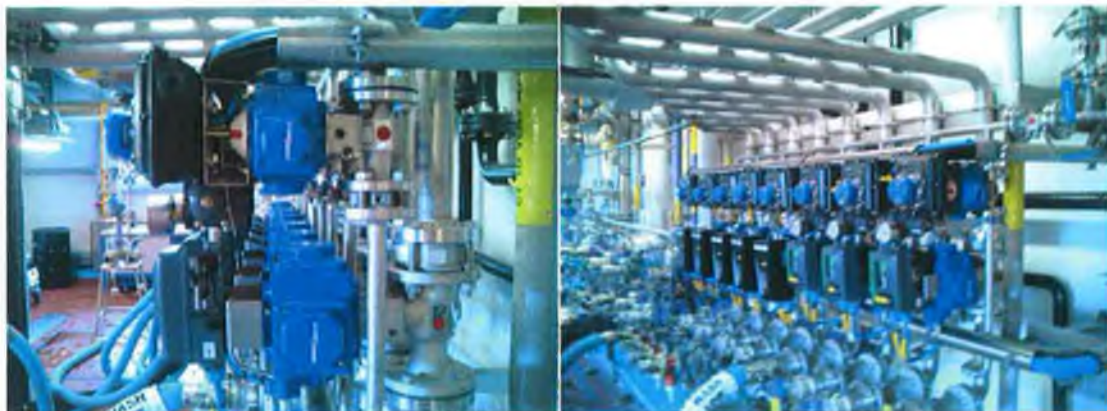
Automated Valve Manifold Side End View and Front View (Compressed Air Users)
