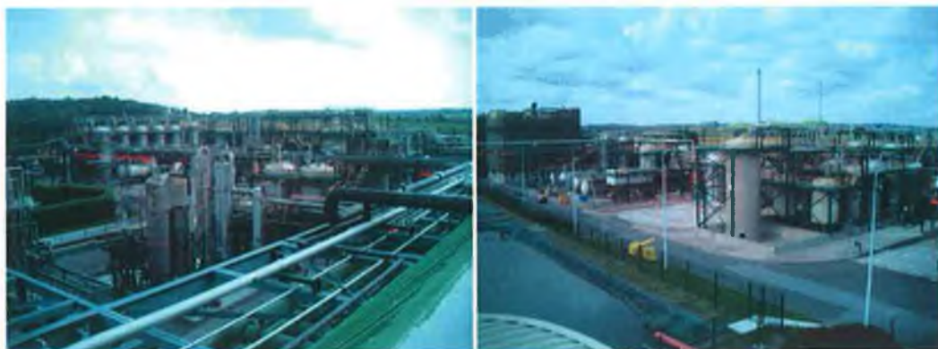
GSK East Side Tank Farm
