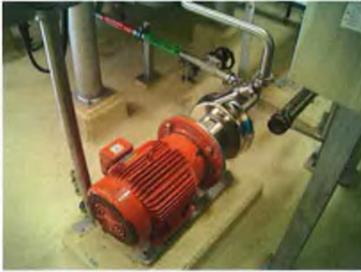
Purified Water Pump with High Purity Piping & Site Retention Ponds, Pipe Rack and Production Buildings
