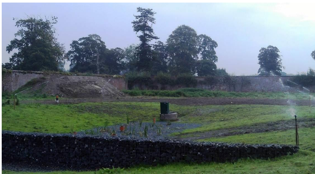
Figure 1.3: Novel Bioswale located at Teagasc Research Centre Oak Park Carlow. showing irrigation system working on the bioswale. What may be seen in the photo is the Gabion stone wall, wetland plants, number 57 stone and the sprinklers. Not seen in the photo is the 5000-litre storage tank for holding the FYDW. Also not seen as it is underground is layers of engineered soil, willow wood chips, pea gravel perforated pipe, outflow concrete sump and three large underground interconnected cisterns.
