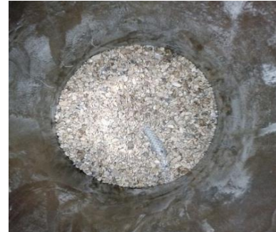
Fig. 2.4: Inside of pipe prior to addition of willow bark.
