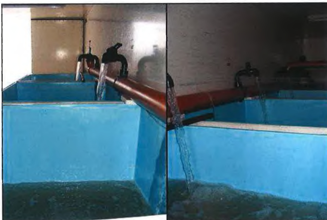
Figure 5. Natural seawater recirculation tanks used for holding live brown crab during the trial. Clarinbridge, Co. Galway.
