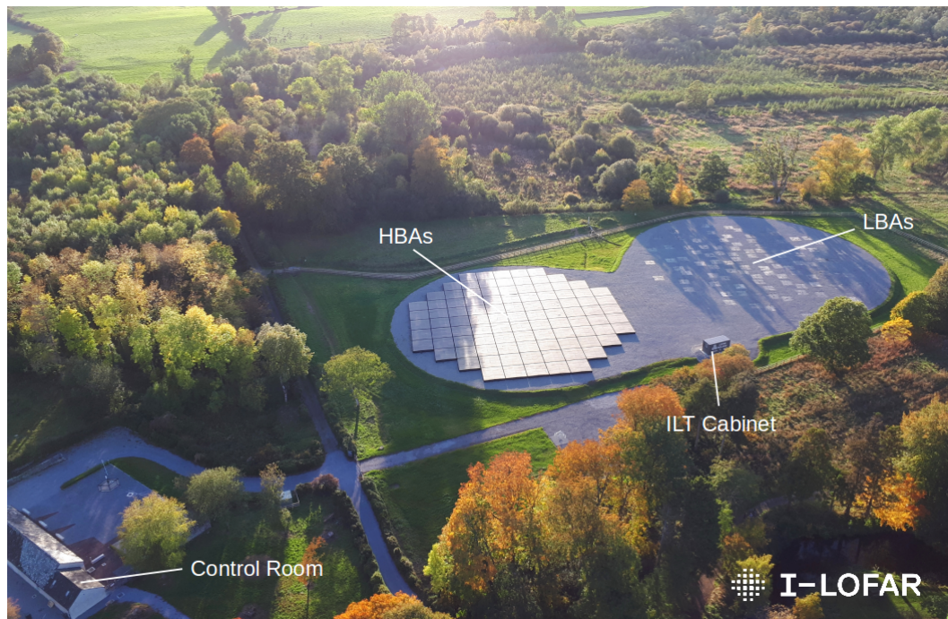
Fig. 2.3 The Irish Low-Frequency Array station IE613 (I-LOFAR) at Birr Castle, County Offaly. Coaxial cables are used to transport data from the Low Band Antennas (LBAs) (10-90 MHz) and High Band Antennas (HBAs) (100-240 MHz) to the ILT Cabinet, where they are amplified, filtered and digitised. Data is sent in international mode at a speed of \sim 3.2 Gbps to Groningen, Netherlands. In the I-LOFAR Control Room, data is processed using REALTA in local mode (Murphy et al. 2021).
