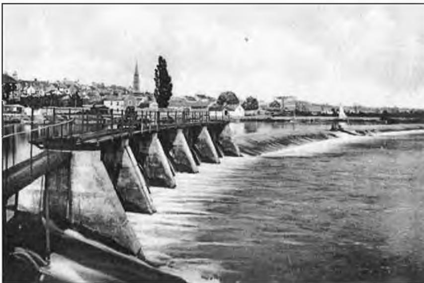
III.21 The impressive structure pictured left is the salmon weir at Athlone, which was constructed towards the end of the 19 th century. At times during the summer when the river is low it is possible to walk across the weir.
