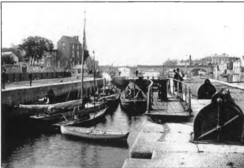
III.17: A number of sail boats and row boats waiting for the water level to equalise in the Victorian lock built by the Shannon Commissioners at Athlone
