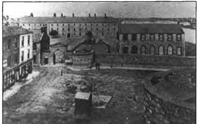
Ill.35: Main entrance to Victoria Barracks
