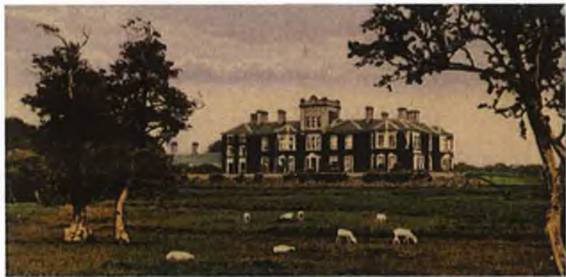
Fig. 175. Back of Creagh House as it was c 1899 overlooking the Deer Park. This house was built by Colonel Charles Knox in 1875. It later became the nurse's home for a tuberculosis sanatorium called St. Teresa's and was very badly damaged by fire. The Agricultural Institute later took it over as a Research Institute after which it was purchased by Mr. O'Malley. James Cuff originally owned the estate.
