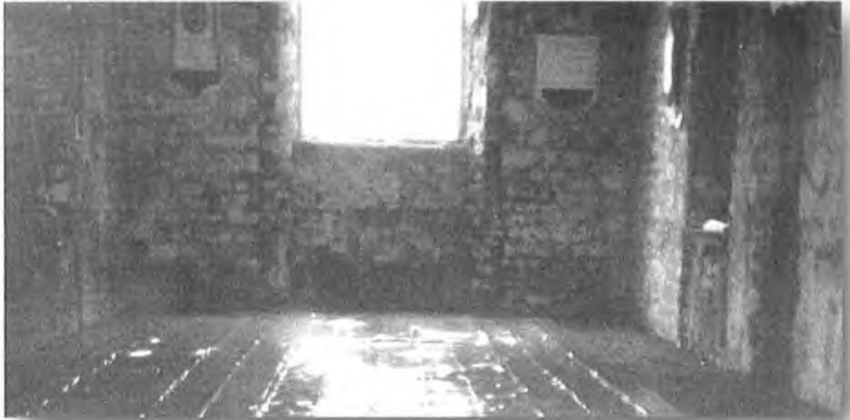
Fig. 126. (A) Interior facing east. On left side; arched recess or doorway see detail below and right side; two openings both blocked up, one being the site of a memorial window now. Note original placement of memorial plaques. Note masonry size.
