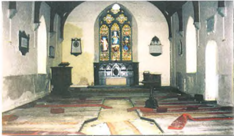
Fig. 129. Church interior prior to renovations in 1990. The raised timber seating areas can be seen together with the Chancel layout and the original location of the memorial plaques, the readers desk, pulpit and the outline for wainscoting. The 1890 Reardos can clearly be seen under stained-glass main window. Dampness is extensive at the east end.
