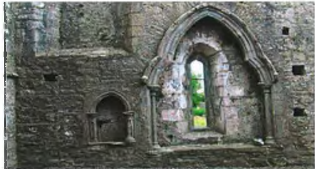
Fig.35. An example of Burriscarra's piscina located beside a sedilia in the Abbey or Priory of the Carmelites which was founded in 1298 probably by Adam de Staunton of Castlecarra. This piscina is beside a trefoil-headed sedilia whose back wall is pierced by a small lancet. This is the lower of the two churches at Burriscarra which occupies the site of a Carmelite Priory which became Augustinian in 1413.
