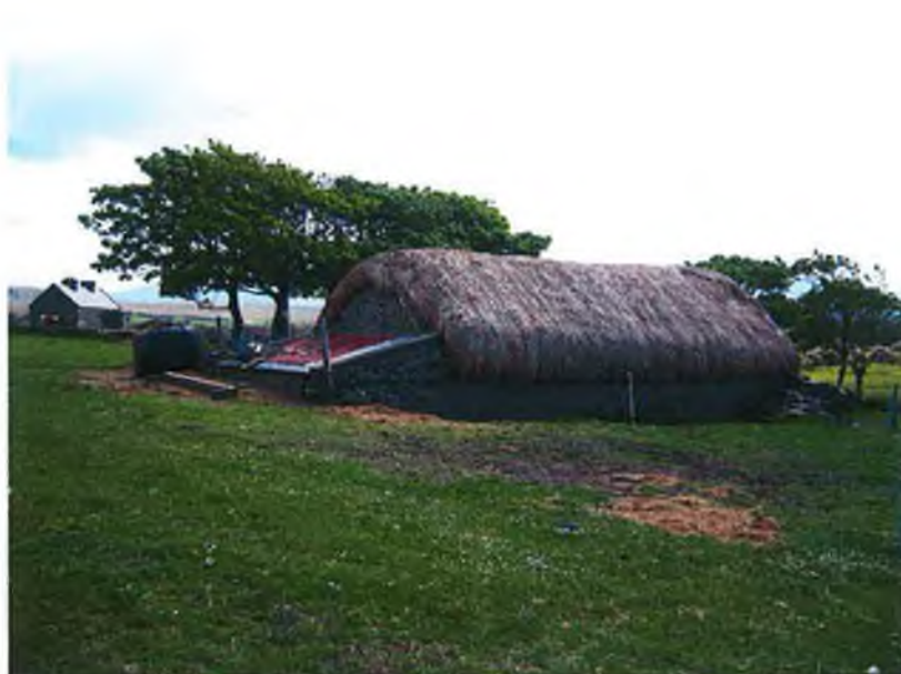
Plate 112 – Thatched byre stone cottage with modified corrugated iron sheets on north gable.
