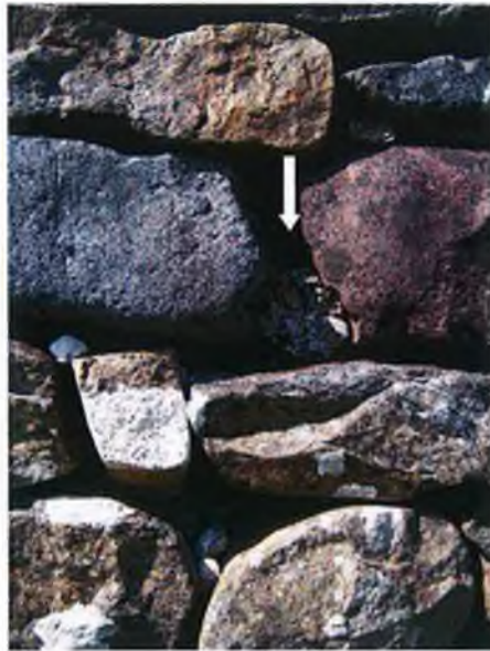
Plate 85 – Shell mortar in the stone walls of the stone cottages (Figure 31).
