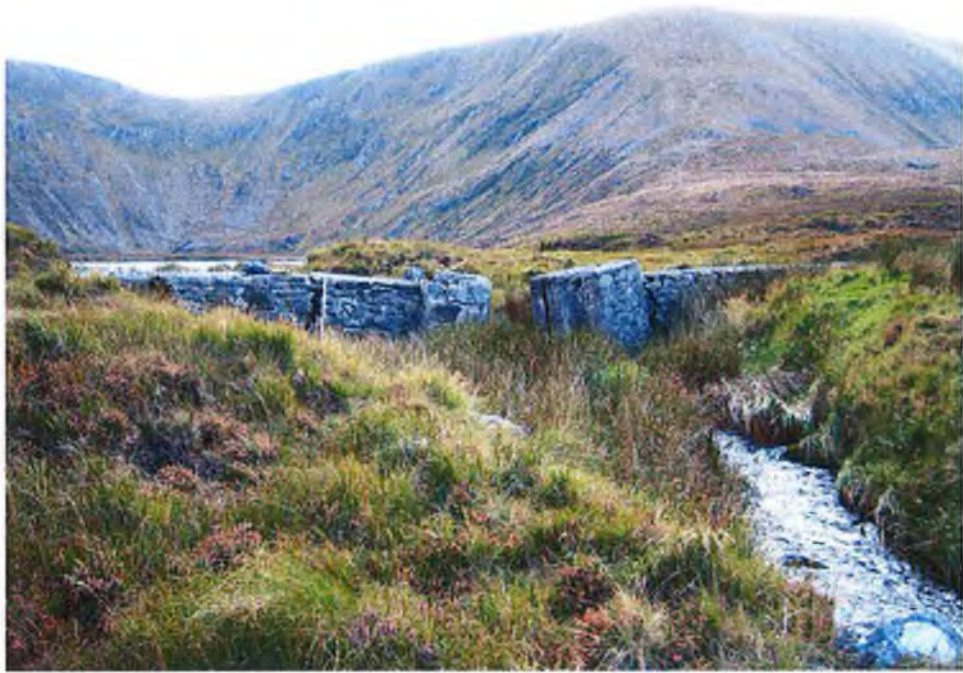
Plate 102 – Dam at Corryloughaphuill Lake.
