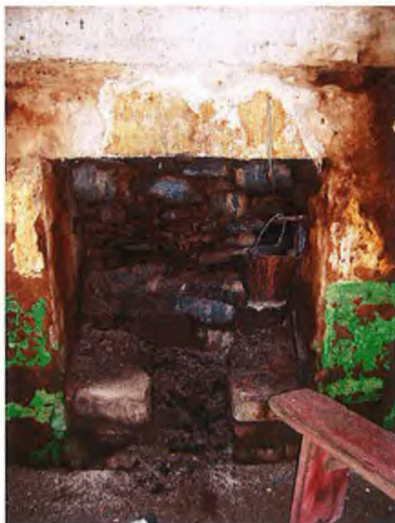
Plate 84 - Iron crane in kitchen or central hearth at Croaghaun townland (Figure 32).
