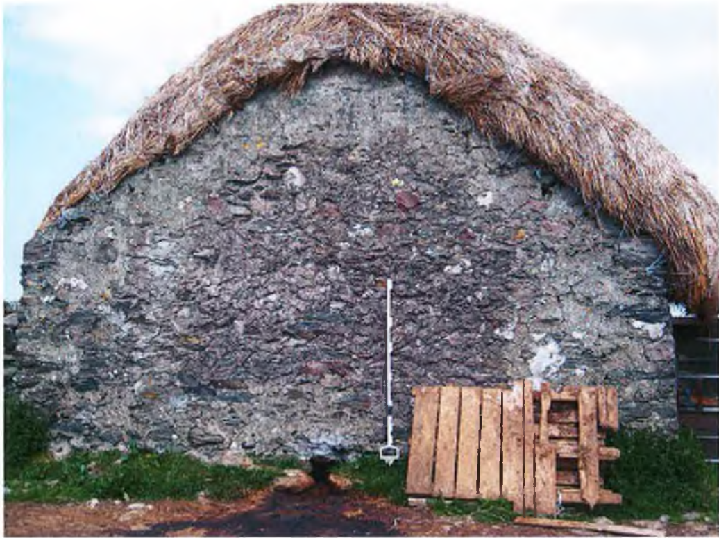
Plate 107 – Figure 37 in section 4.4.1.2 of chapter four. Tie-beam thatching. Note the scraws and rope on the thatch of this byre-dwelling near Ballycroy village. The stone cottages and stone outhouses recorded in this study (Figures 29-42) would have been thatched in the same way. There are only one or two traditional thatchers left in the locality.
