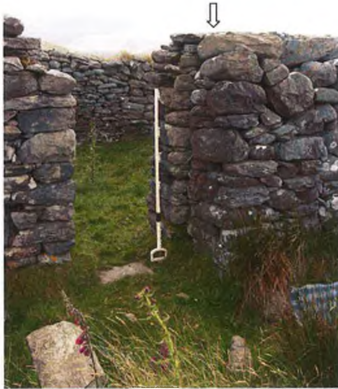
Plate 63 – The buttressed wall (double wall) of Scardaun house indicated by white arrow.
