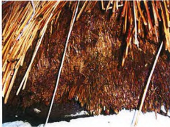
Plate 88 - Close up of rush thatching in Figure 37.
