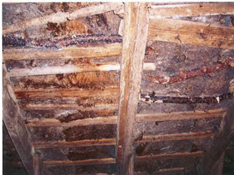
Plate 109 – Note the different types of wood used in the rafters.
