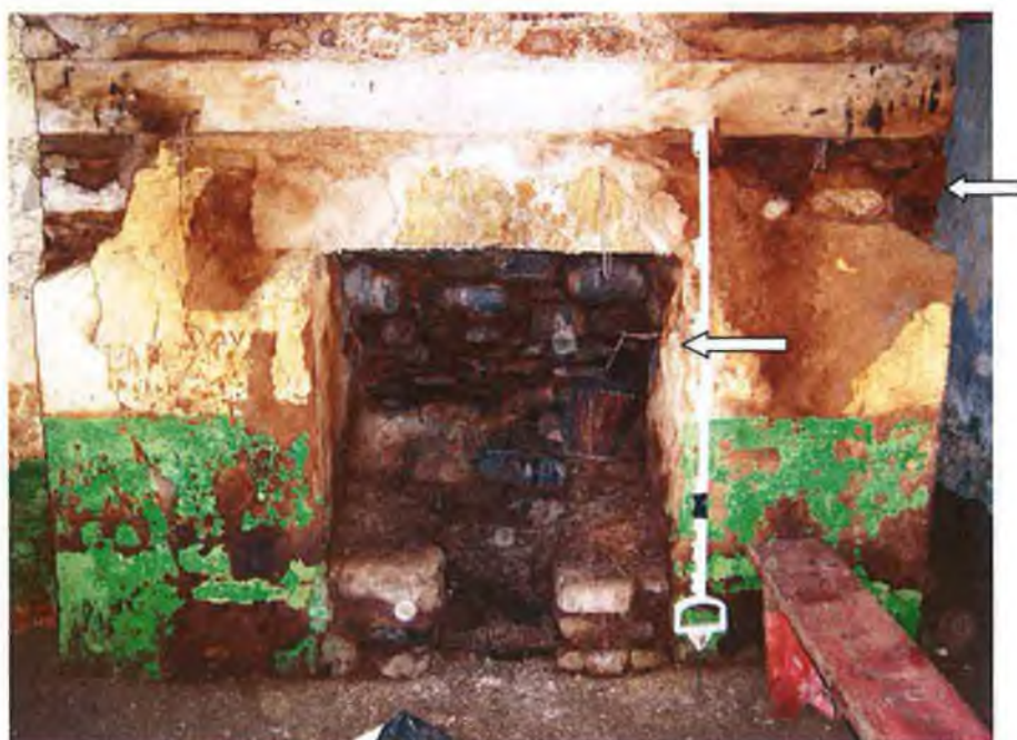
Plate 114 – Iron crook in central kitchen hearth indicated by white arrow at Croaghaun townland. Figure 32 of this study. Note erosion stripping plaster to expose stone underneath indicated by white arrow.
