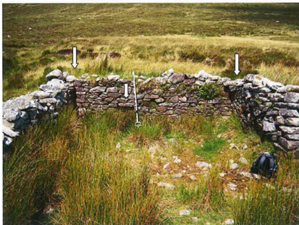
Plate 72 – The east gable wall in livestock enclosure at site 7 with central hearth indicated by white arrows. The white meter stick is used to give scale to the structure (supervisor's meter stick).
