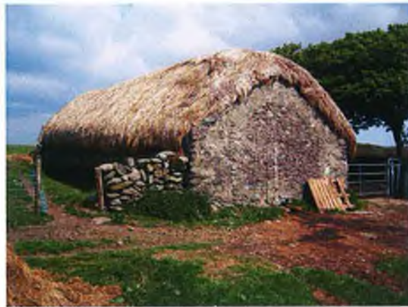
Plate 89 – South facing gable with byre visible beside meter stick (Figure 37).
