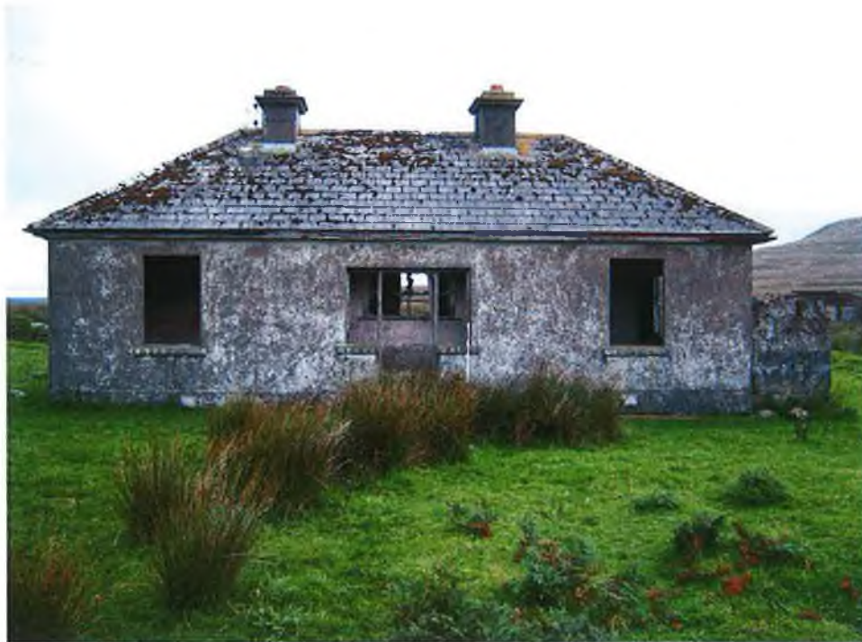
Plate 57 – The Congested Districts Board house at site 5.
