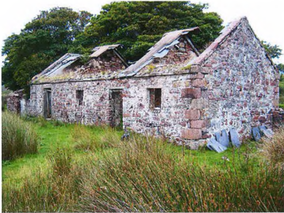
Plate 54 – The house (Figure 36 in section 4.4.1.2) at site 5, Bellagarvaun townland.
