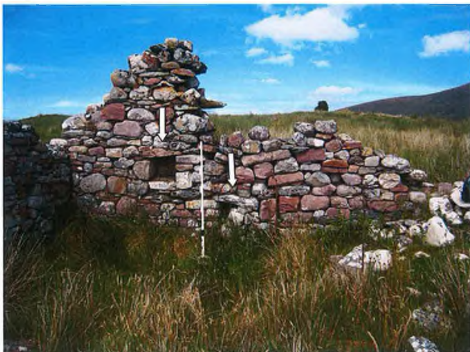
Plate 49 – Keeping hole in east gable wall of house and central hearth (infill). These features are indicated by the white arrows.
