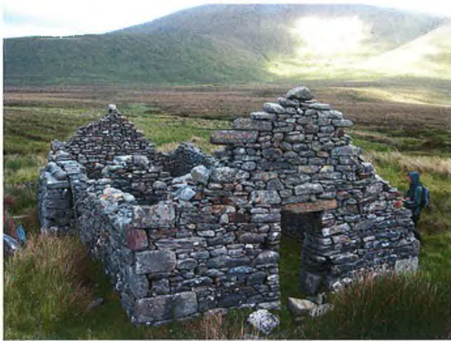
Plate 61 – Scardaun house with the Nephin Beg Mountain range in the background. The buttressed north wall is recognisable and the west gable has been modified with a doorway, as the entrance from the kitchen has been filled in.
