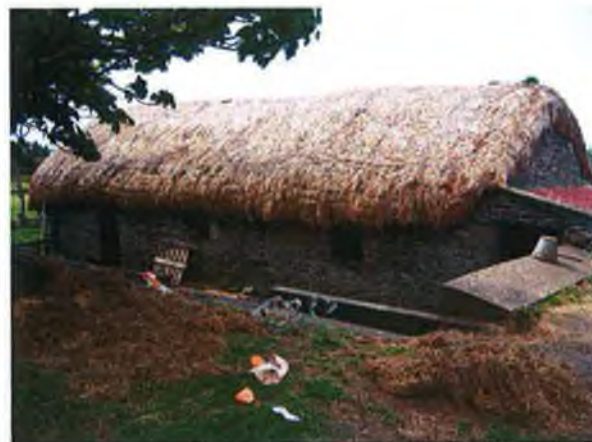
Plate 90 – Note the tiny windows for light and extension on the north gable, a modification for present farming practices.
