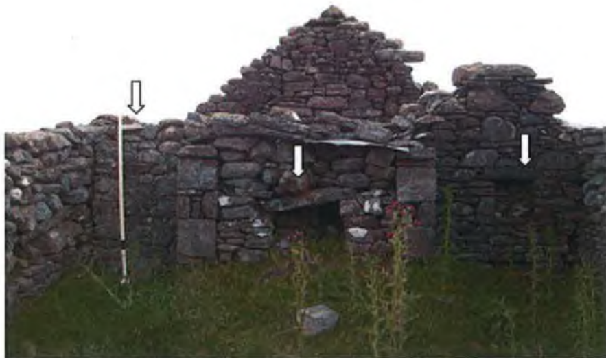
Plate 62 – The interior of Scardaun house. Note the central hearth and keeping hole indicated by white arrows and doorway to second room has been modified (infill).
