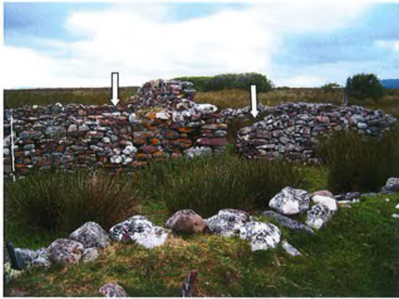
Plate 46 – Note the modifications (windows infill and extension to east gable) to original house structure indicated by white arrows.
