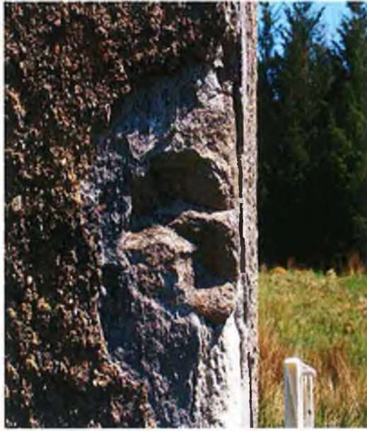
Plate 87 - Illustrates erosion and plaster thickness on the exterior of the stone cottage at Croaghaun townland (Figure 3). Note the two types of mortar on the exterior of house, the sandy limy mortar first on the stone, then the thicker more pebbly mortar orange in colour. Erosion is slowly stripping both these mortar layers to reveal the stone-work underneath.
