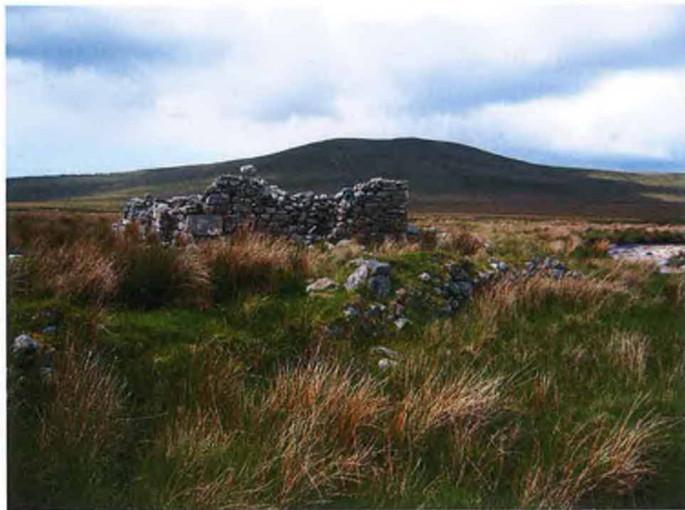
Plate 17 – Shows the proximity of houses, outhouses and stone walls to the rivers edge at site 1.
