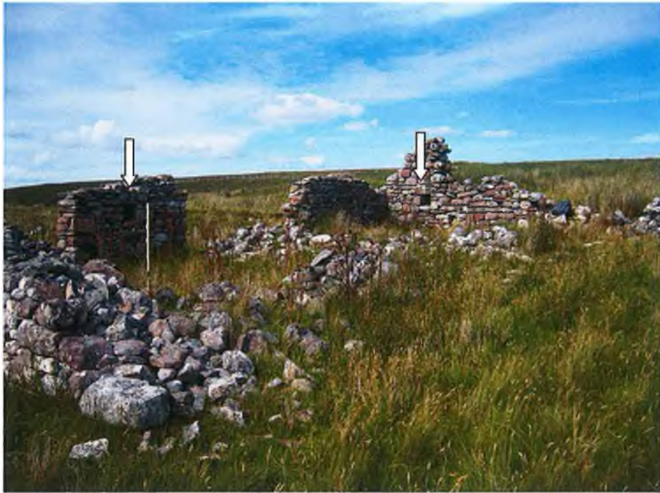
Plate 50 – Figure 35 in section 4.4.1.2. Note the keeping holes in walls indicated by the white arrows.
