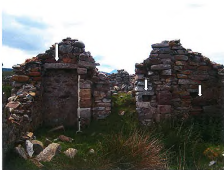
Plate 35 – Central hearth in house at site 3 with keeping holes in walls. The entrance into the second west room has infill (underneath the lintel stone indicated by white arrow), a later modification from the original structure.
