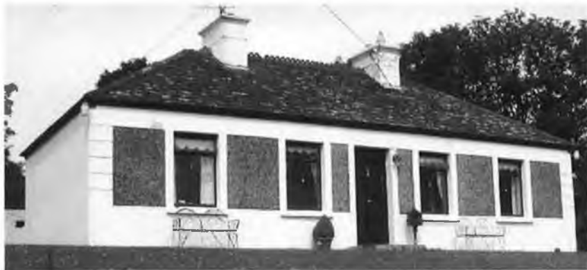
Plate 10. (Hipped Roof Cottage Breaghwy)
