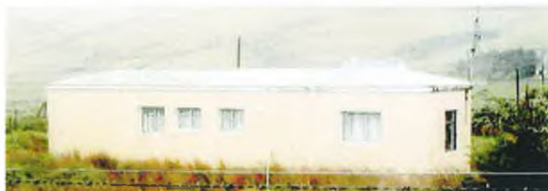
Plate 71 Poor Quality Housing Knockadaff
