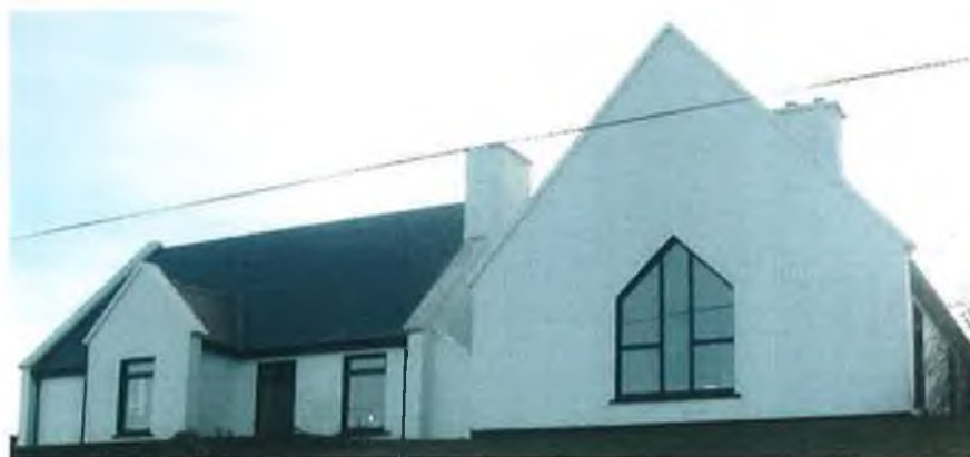
Plate 57 Cottage with modern extension
