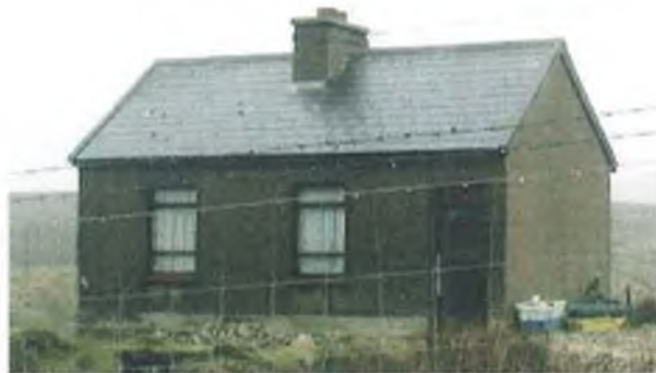
Plate 70 Poor Quality Housing Knockadaff
