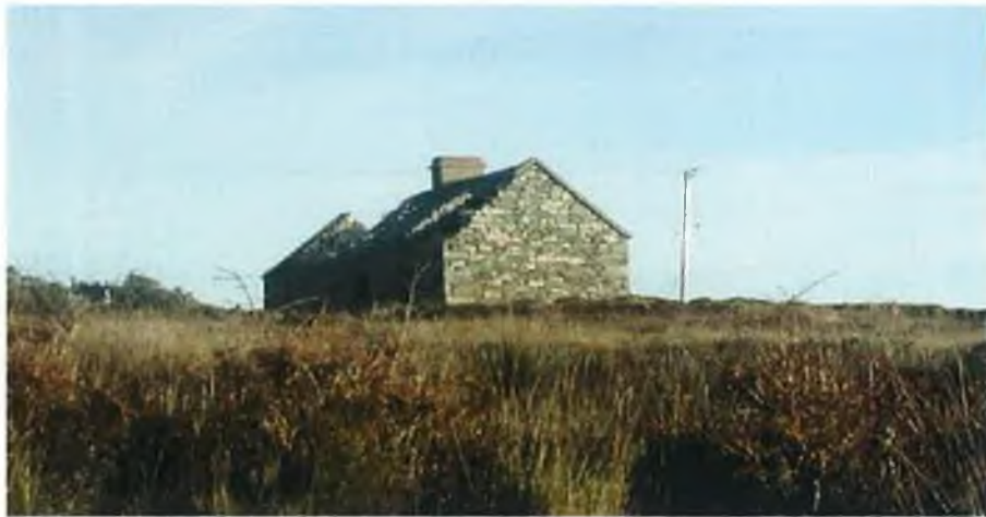
Plate 47. (Derelict cottage Slievemore- note fine stonework)
