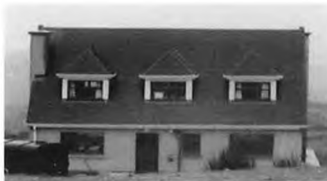
Plate 79 Modern Dormer Knockadaff
