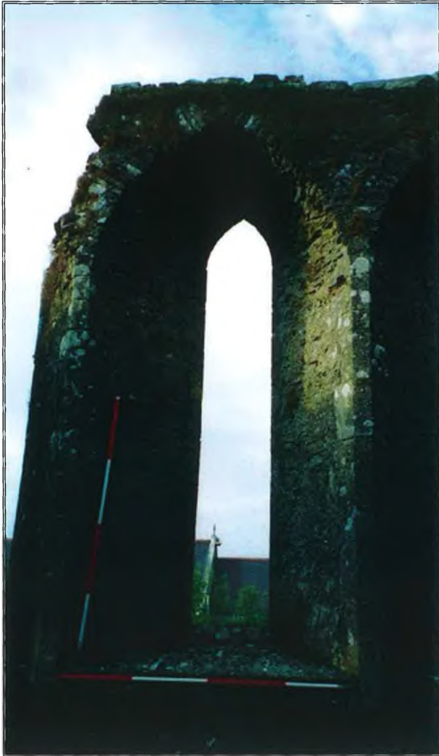
Plate 5.3: Lancet window in the north wall of the choir of Strade Friary, dating from the thirteenth century. It is a characteristic feature of the Early English phase of Gothic architecture.
