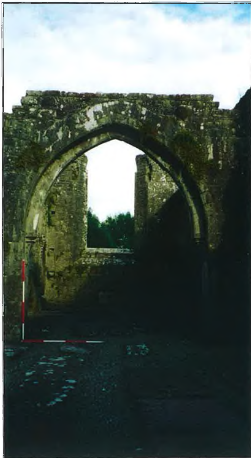
Plate 6.4: Chancel arch in Strade Friary with the remains of the east window behind it
