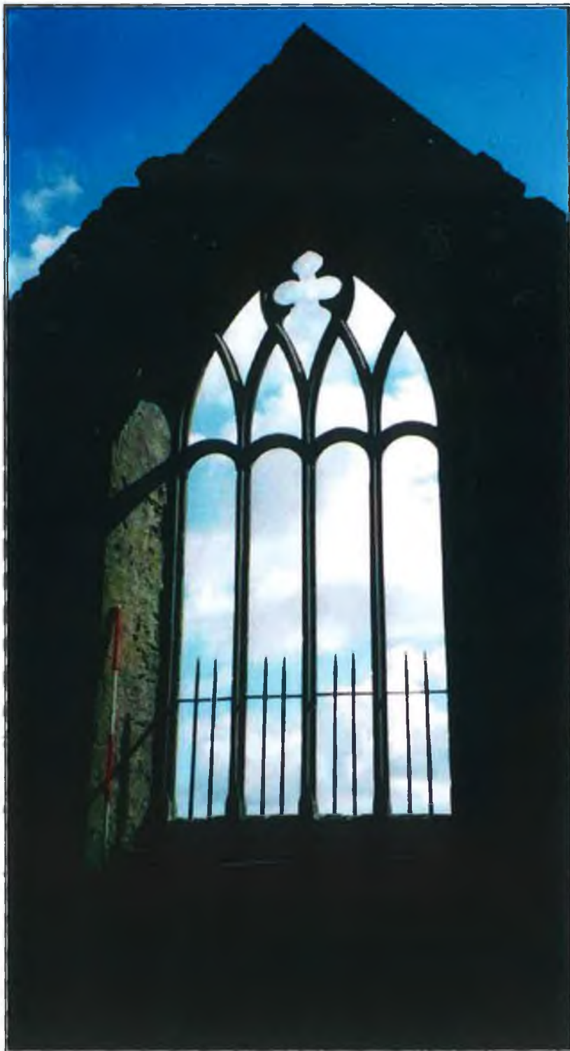
Plate 5.14: Window in the south wall of the transept of Moyne Friary
