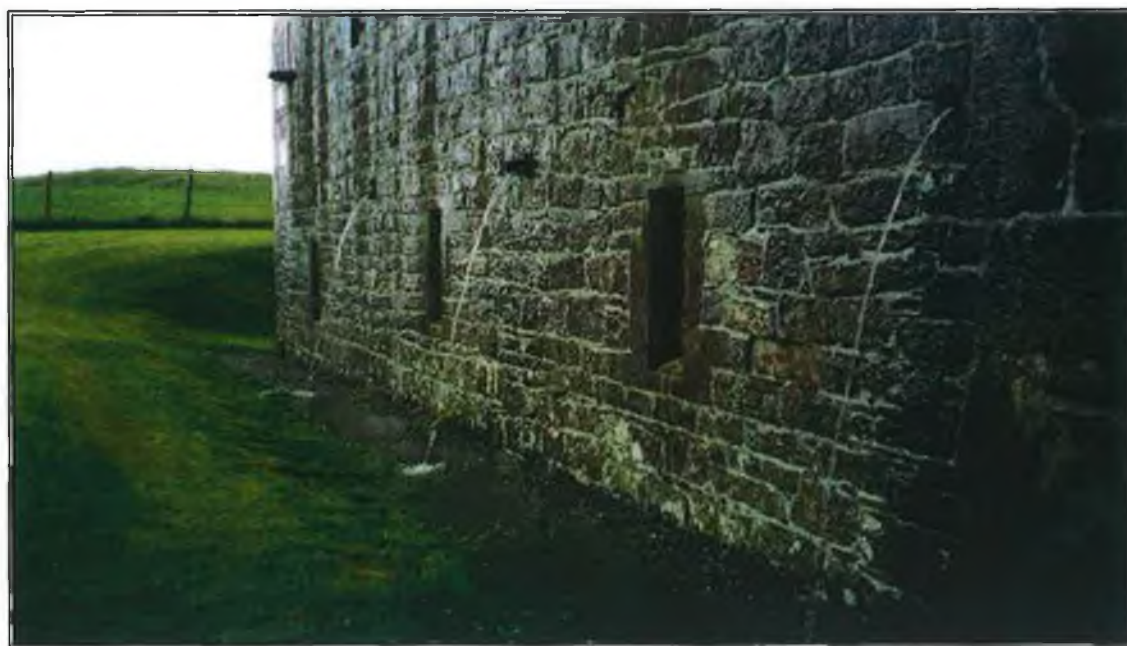
Plate 5.32: Rainwater being channelled away from the east range of domestic buildings at Rosserk
