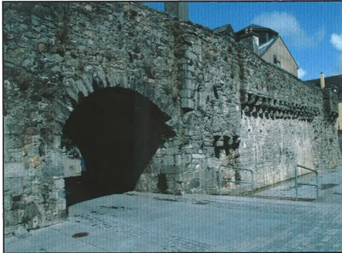
Figure 4.10: Section of Renovated Town Wall, Spanish Arch, Galway 2009. Photo: John Towler.
