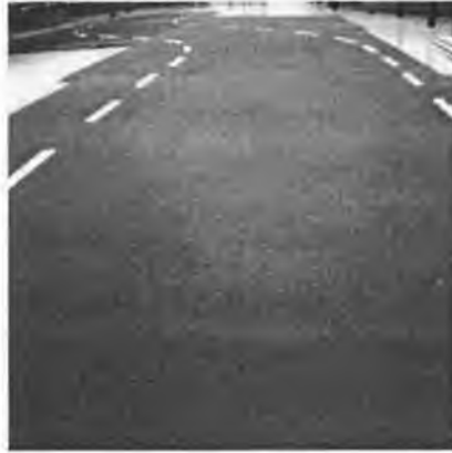
Figure 35. Captured image of roadway section with S-bend
